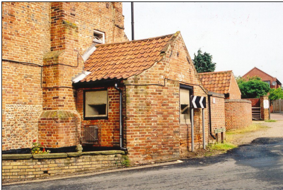
Fig. 1 - UORN 5479: pillbox disguised as an outbuilding (now used as a boiler room) attached to the Manor House in the centre of Acle. The embrasures would have enabled fire to be directed down The Street as well as Old Road.
