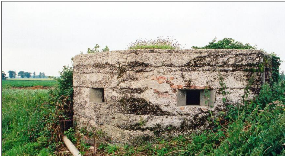
Fig. 4 - UORN 5474: type 22 pillbox on the north-west outskirts of Acle. It has been stripped of its exterior brick shuttering.
