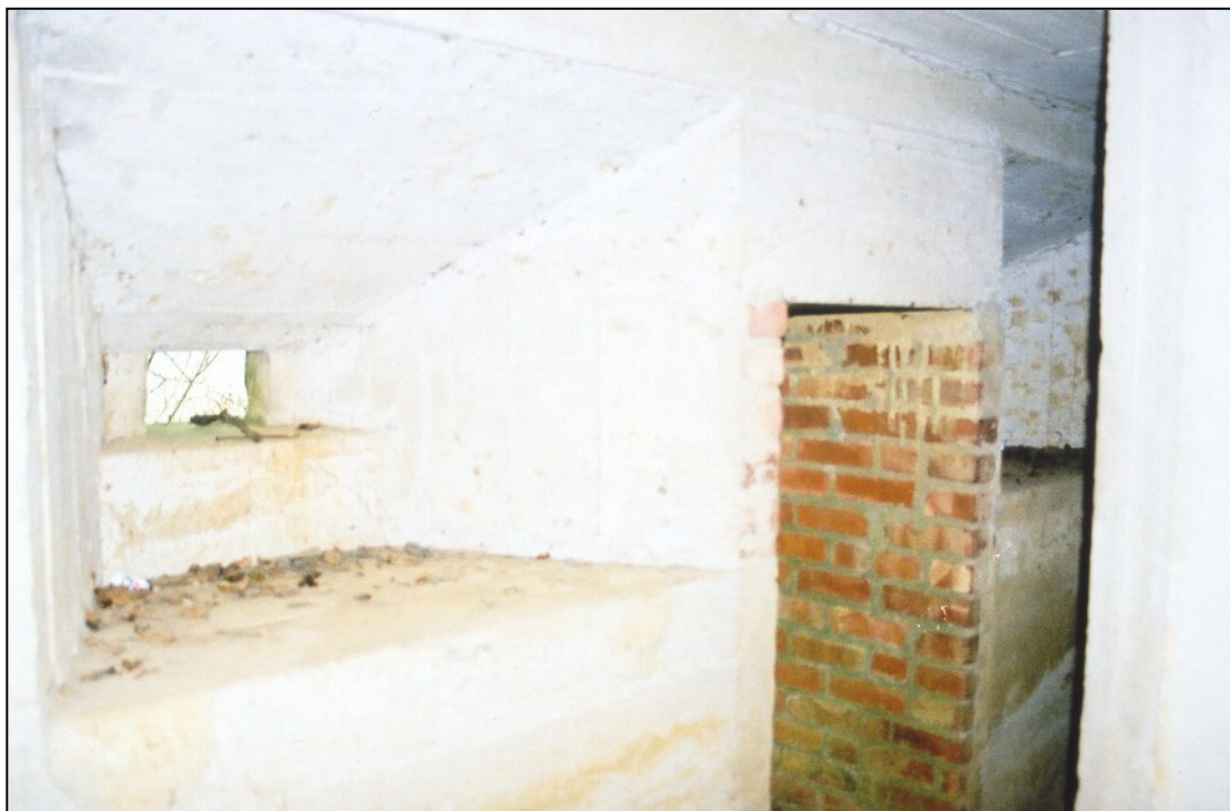
Fig. 6 - UORN 2412: concrete firing shelf at an embrasure for a Bren gun. Many of the interiors of the Penshurst area pillboxes are in a clean condition with little evidence of vandalism.
