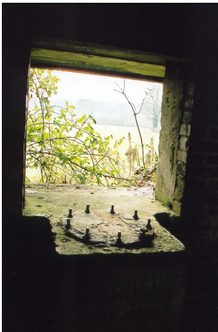
Fig. 8 - UORN 2434: the holdfast for the positioning of a 6pdr. gun, with its nine bolts still intact.
