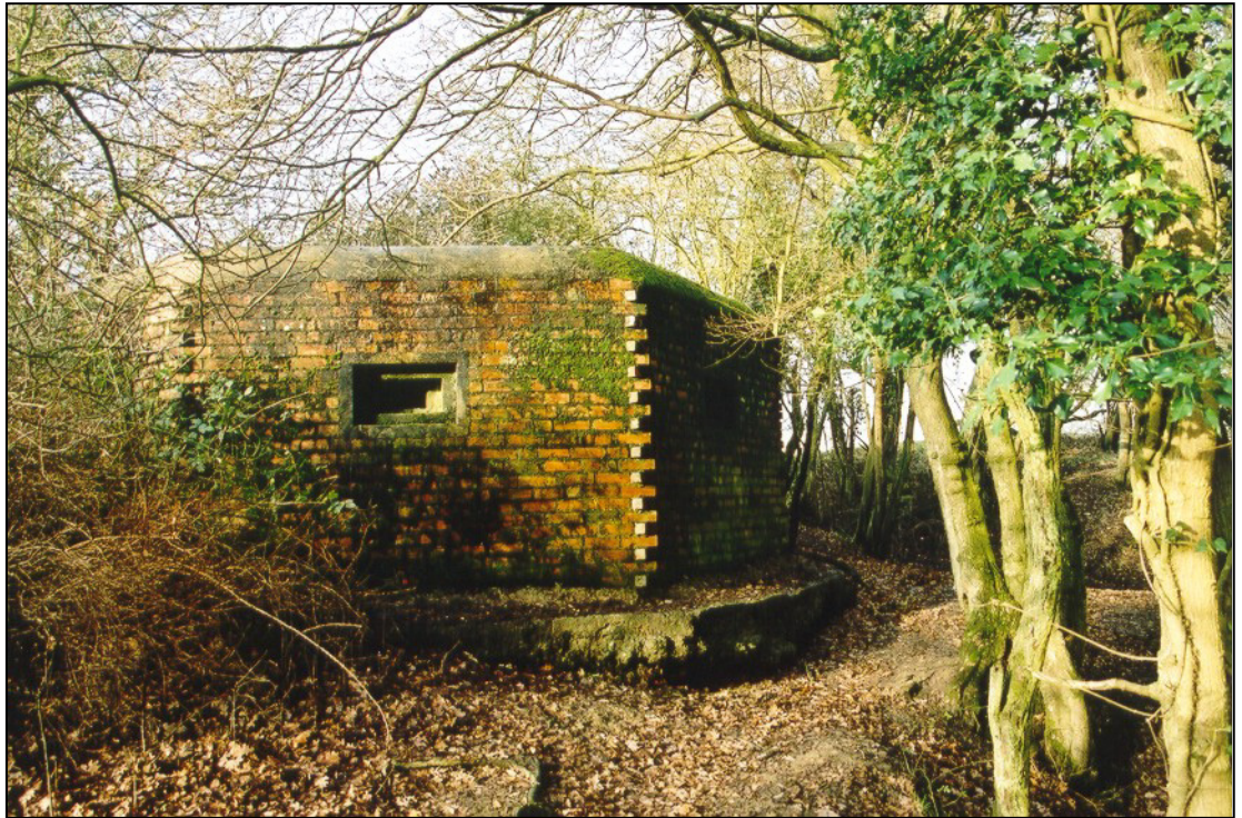
Fig. 4 - UORN 1883: type 24 pillbox on wooded bluff above the River Medway. The untrimmed bricks projecting at the angle of the faces can be seen.
