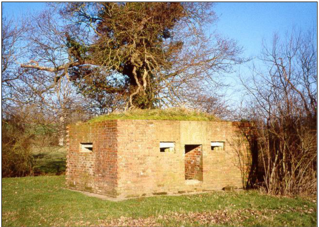
Fig. 5 - UORN 2428: the 'classic shape' of the type 24 infantry pillbox, with an embrasure each side of the entrance. The soil and grass on the roof is probably from its original camouflage.
