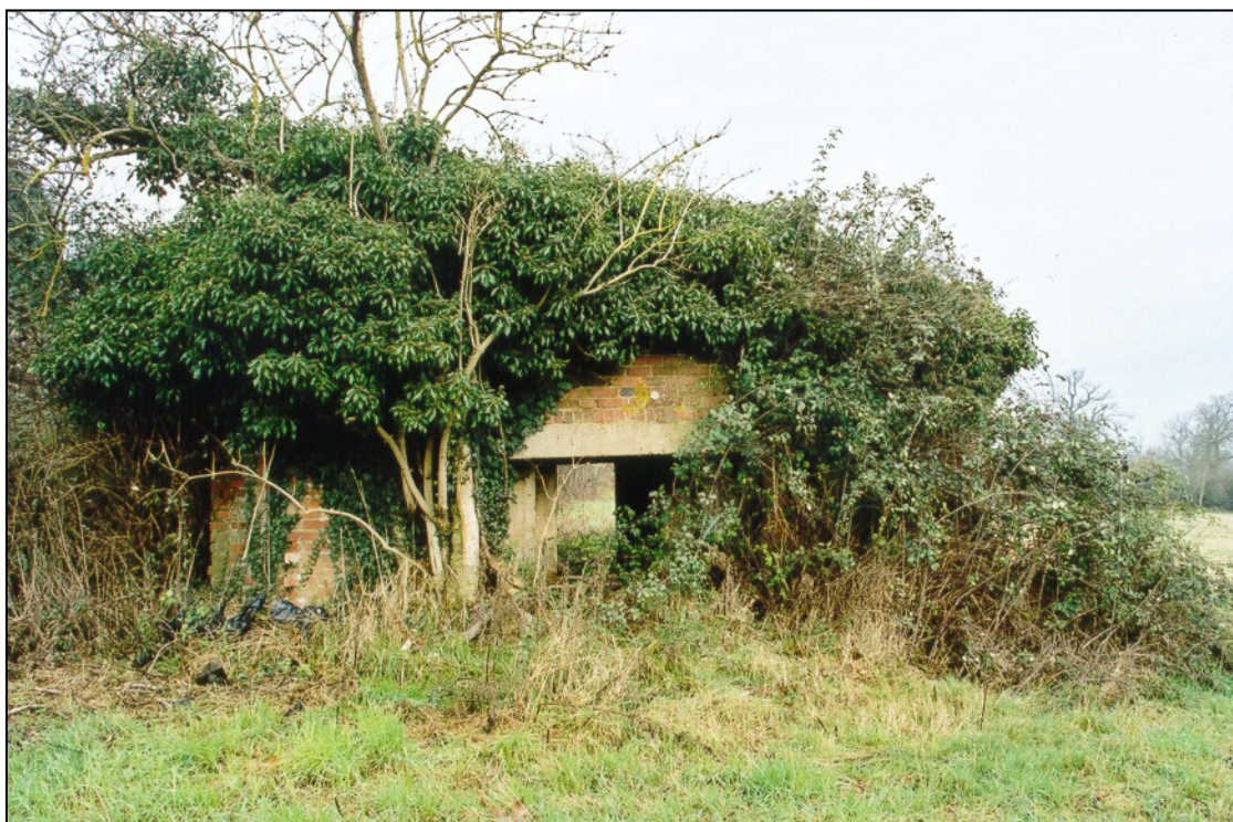
Fig. 7 - UORN 2434: heavily-overgrown type 28 anti-tank gun emplacement to take a 6pdr. gun. It was positioned to fire downhill at the important crossing of the GHQ Line at Long Bridge south of Penshurst village.
