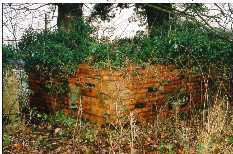
Fig. 5 - UORN 9552: brick pillbox of an unusual trapezoidal shape made to fit its site at a corner in the southern line of anti-tank blocks.
