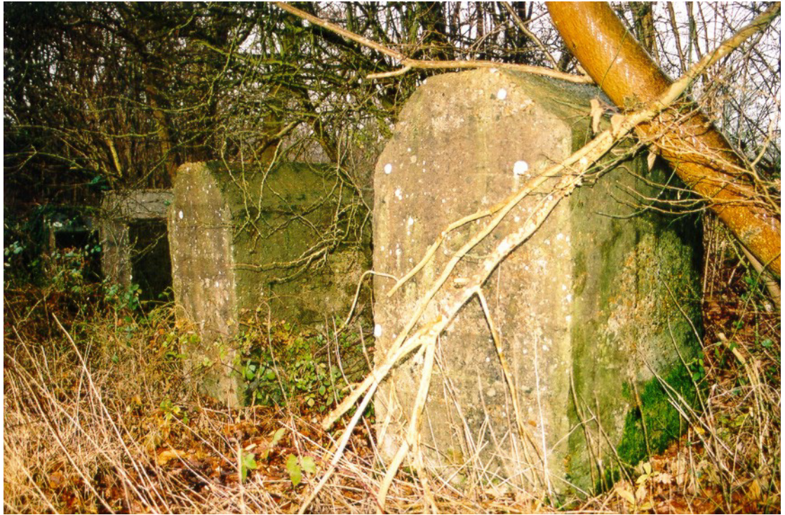
Fig. 8 - The distinctive 'tombstone' shape of the Cripp's Corner anti-tank blocks can be seen from these examples [UORN 9553].
