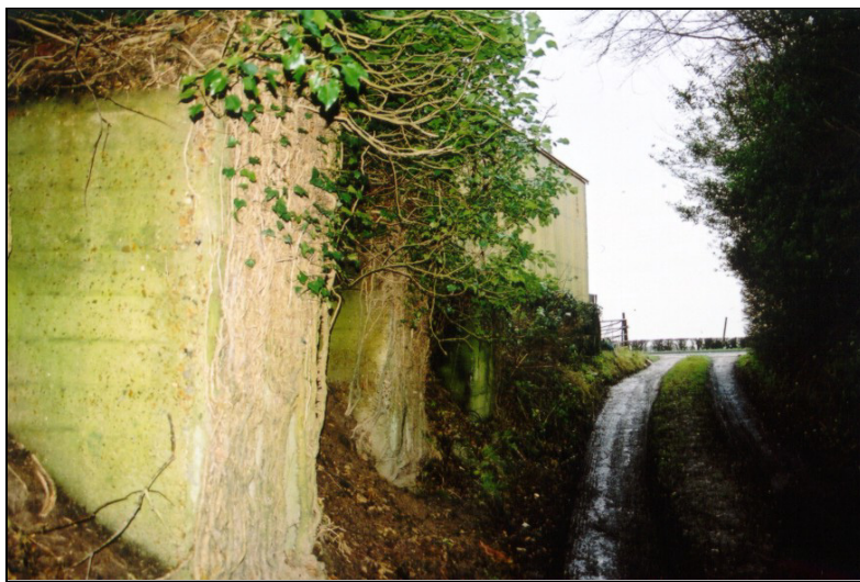
Fig. 7 - UORN 16915: anti-tank blocks exposed in the bank of Compasses Lane at Swaile's Green, showing their full height of nearly seven feet.
