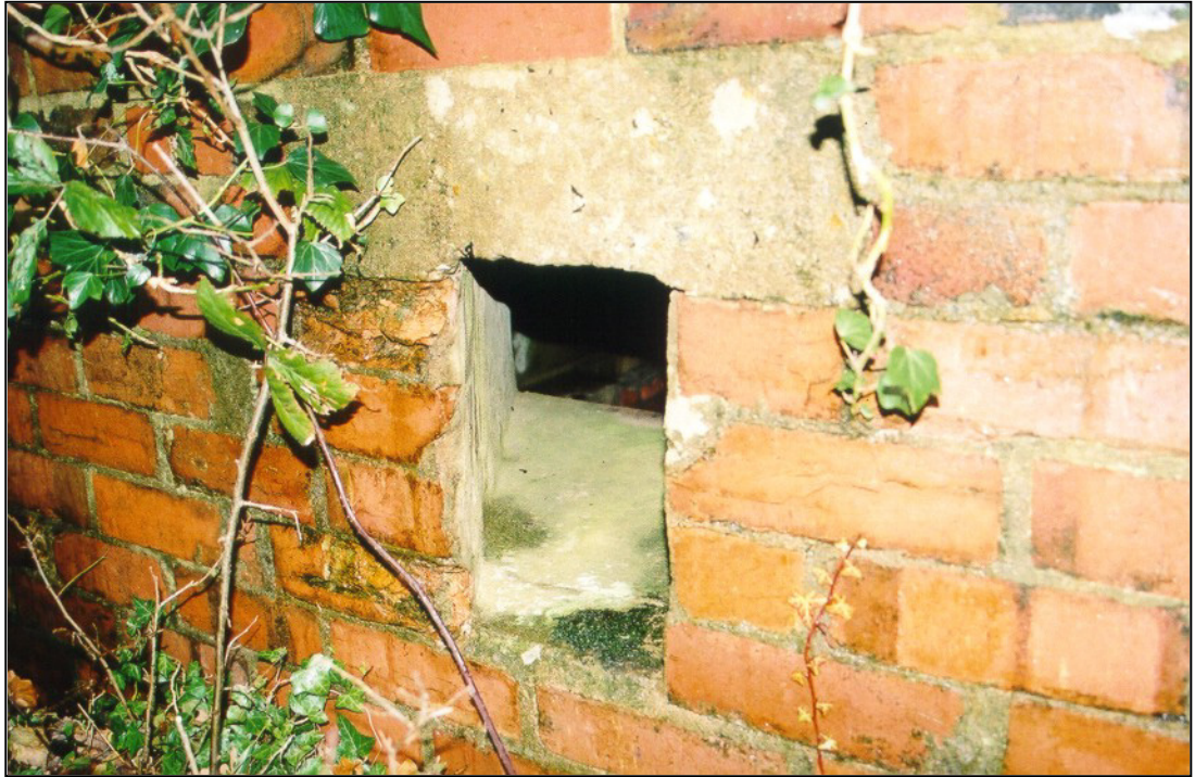
Fig. 6 - UORN 9552: rifle port set at a slant to the pillbox face to enable fire to be directed to the north.
