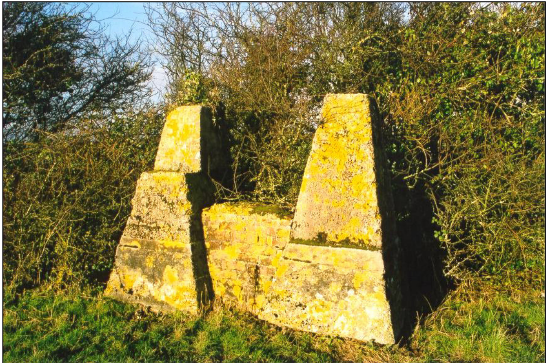
Fig. 9 - UORN 16330: fragment from a roadblock, consisting of two tetrahedrons ('pimples') set on concrete bases and connected by brickwork. How this related to the main structure of the roadblock, now destroyed, is unknown.
