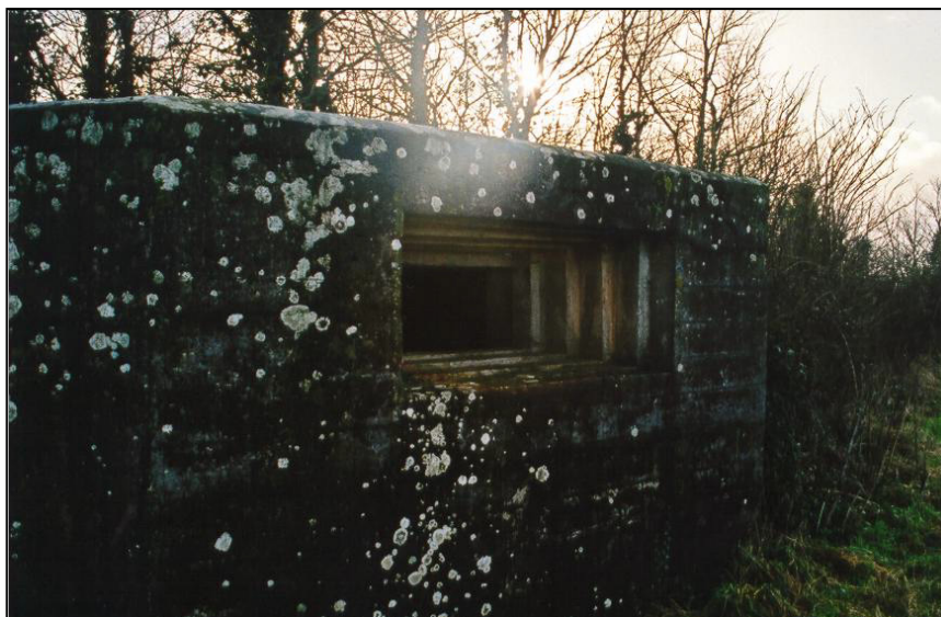
Fig. 6 - UORN 309: the main embrasure of a Vickers machine gun emplacement on Pawlett Hill.
