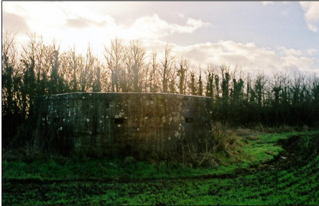
Fig. 7 - UORN 307: shell-proof, thick-walled type 24 pillbox positioned to fire north over the summit of Pawlett Hill.
