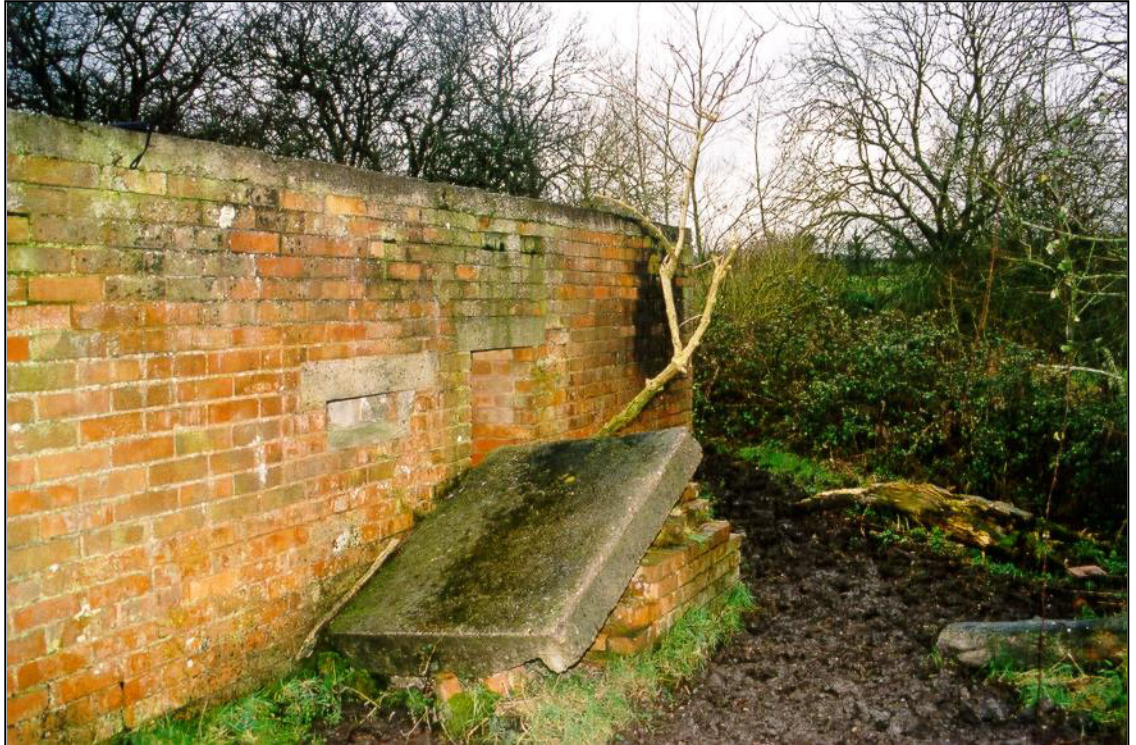
Fig. 5 - UORN 13970: the brick entrance porch with its concrete roof slab has collapsed.
