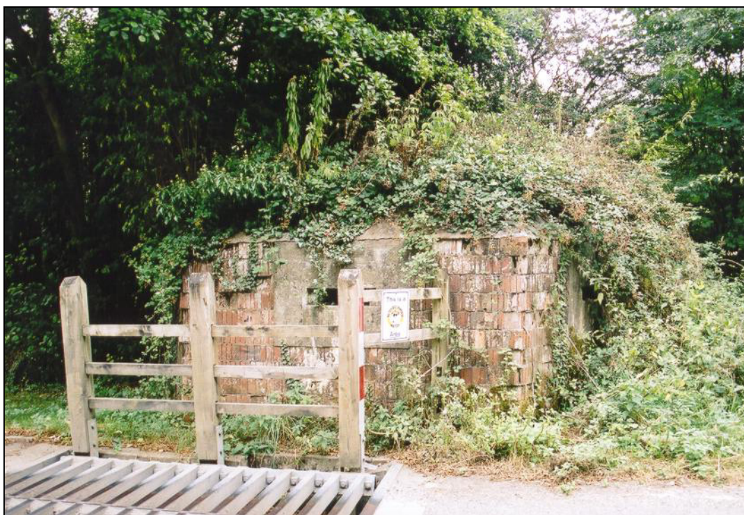
Fig. 9 - UORN 6478: brick-shuttered type 22 pillbox by the lane at Lower Denford. It is considered that the removal of its overgrowth would enhance its historic interest rather than detract from the locality in which it stands.
