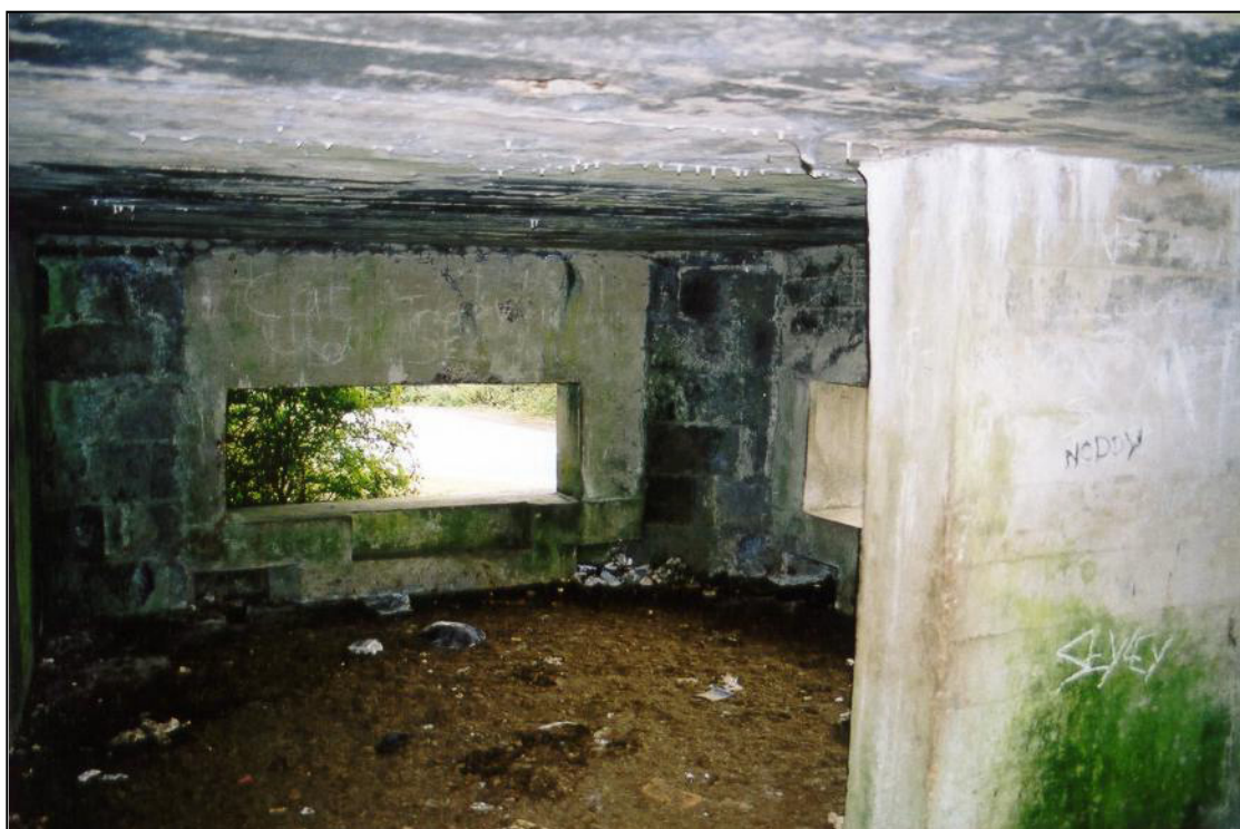
Fig. 7 - UORN 6479: interior of the anti-tank gun emplacement showing the dividing wall of the separate LMG chamber to the right. The condition of this structure, although essentially 'Good', is dirty and dilapidated, and it is in urgent need of some protection.
