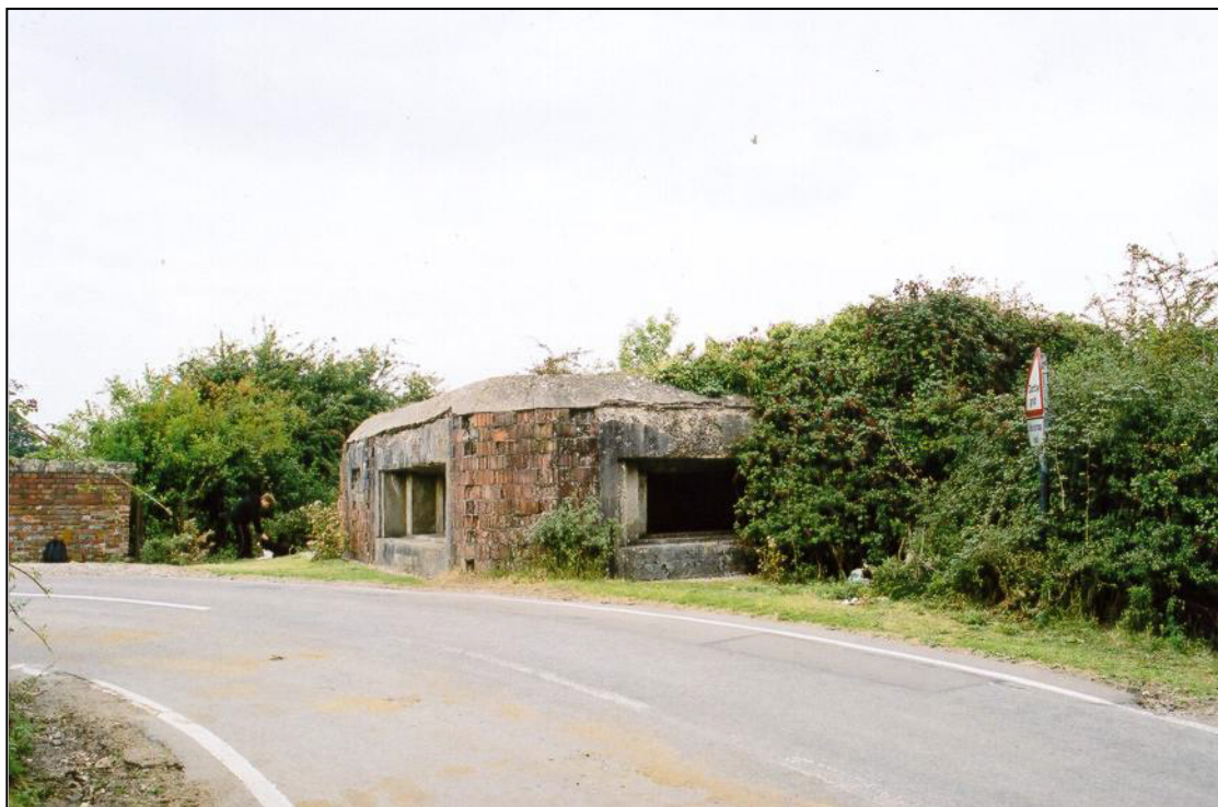
Fig. 6 - UORN 6479, showing its two anti-tank gun embrasures covering both directions of the road.
