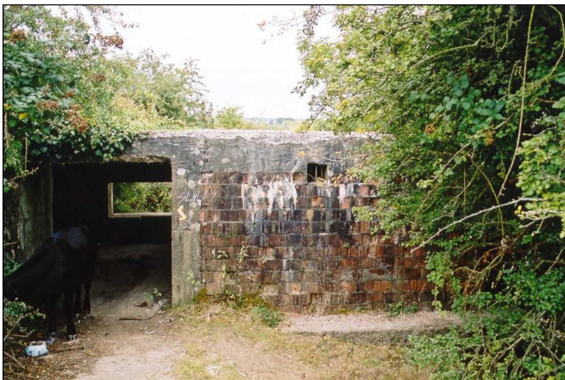
Fig. 8 - UORN 6480: 2pdr. anti-tank gun emplacement, with a single main embrasure, adjacent to UORN 6479 and in a similar dirty condition. The northern edge (right hand) of its concrete base is being undermined by the erosion of the bank above the canal on which it stands.
