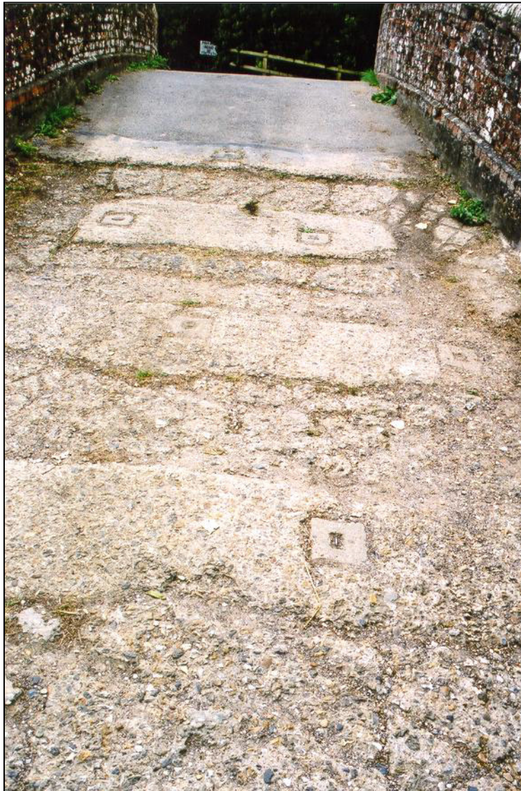
Fig. 10 - UORN 8822: concrete plugs in the surface of the bridge at Wire Lock, which, when lifted, would reveal square sockets for the insertion of blocking posts or rails.
