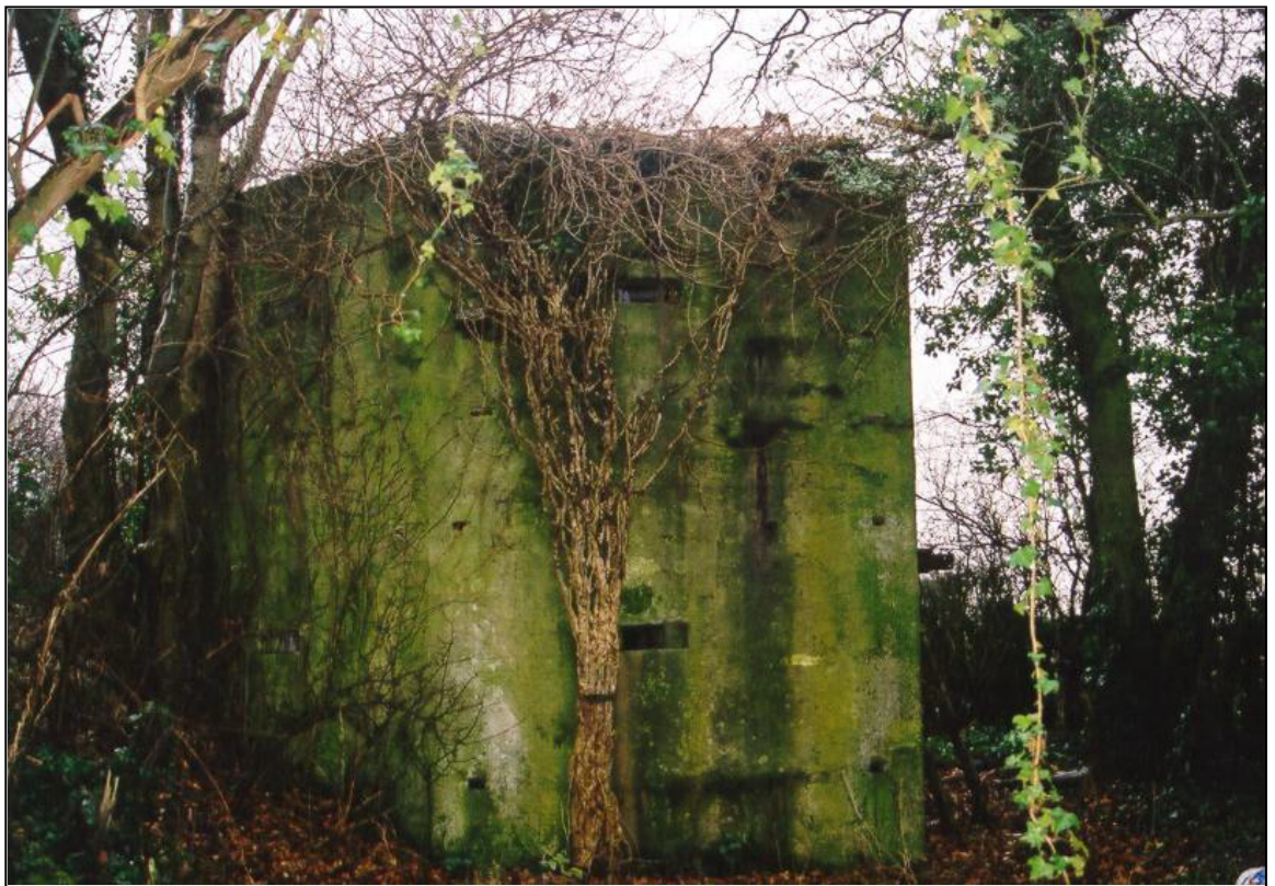
Fig. 5 - UORN 6780: rare double-decker pillbox with firing points on two floors.
