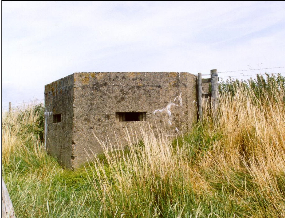
Fig. 8 - UORN 6083: good example of a type 22 pillbox dug into the sea bank on Bawdsey Marshes.
