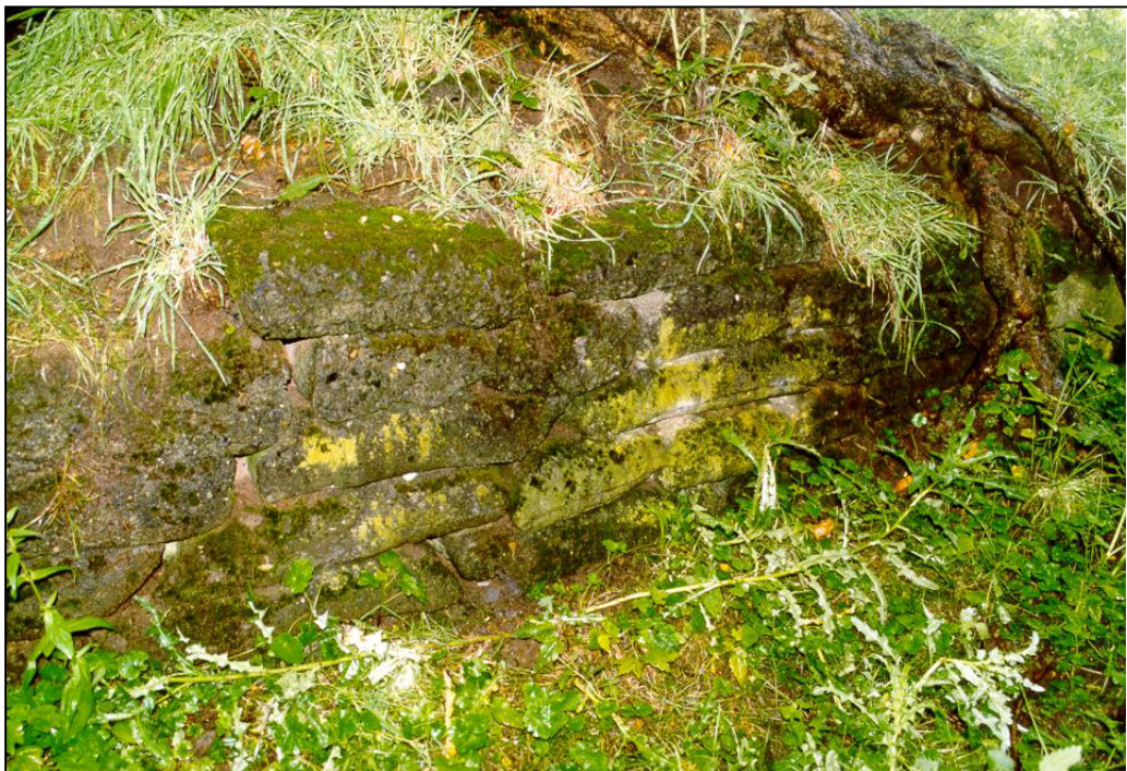
Fig. 11 - UORN 6061: detail of concreted sandbags forming a surrounding reinforcement to the pillbox.
