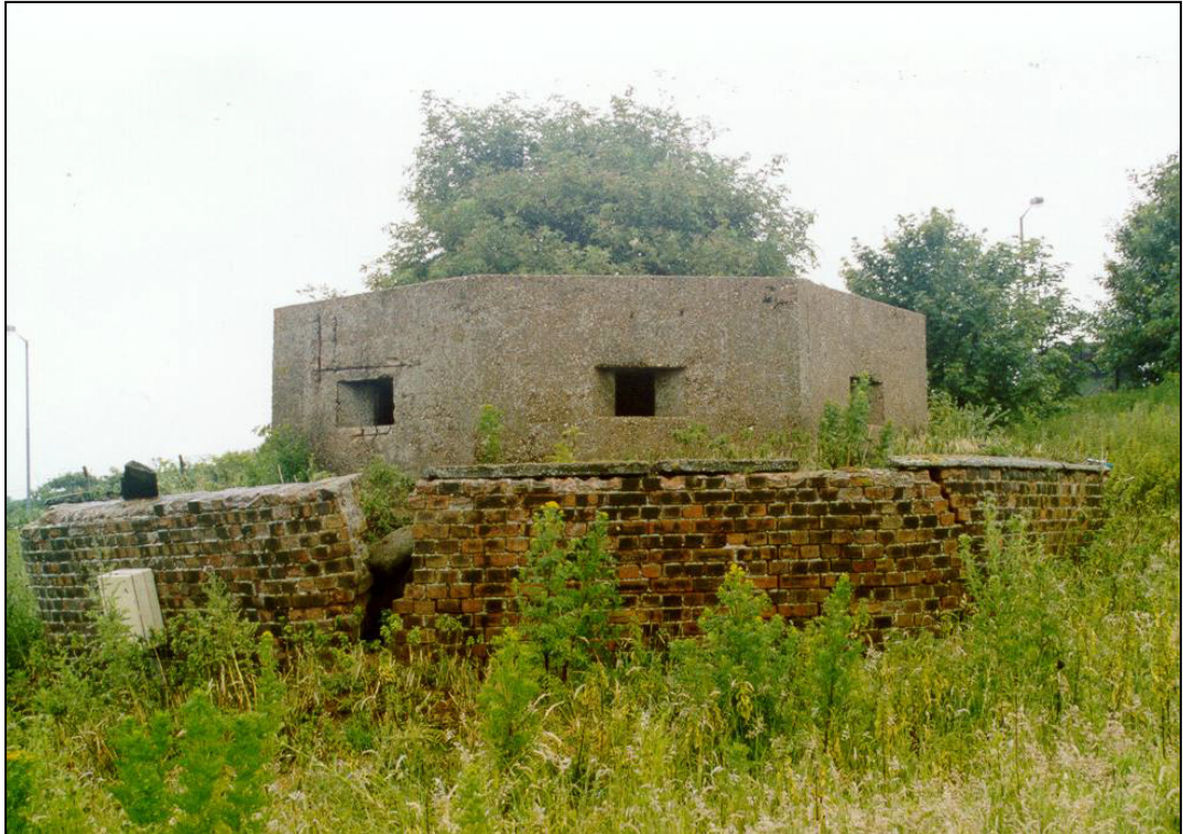
Fig. 10 - UORN 7488: type 24 pillbox with distinctive 'skirt' at eastern end of Bawdsey Manor estate.
