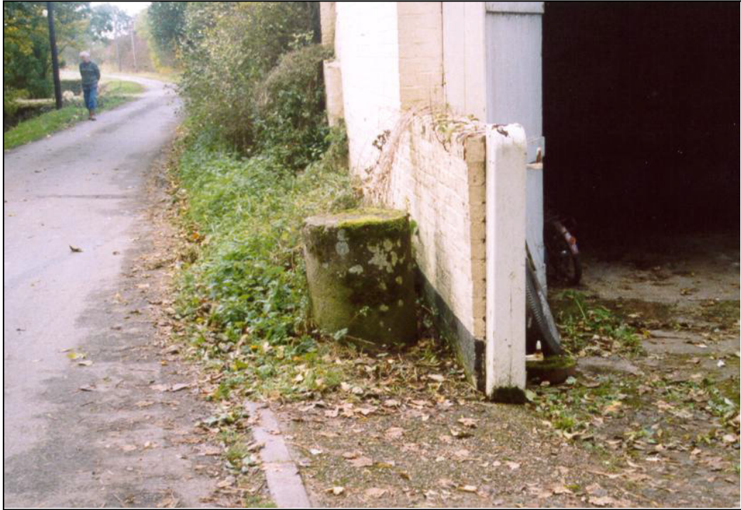
Fig. 8 - UORN 5138: the only surviving evidence of one of several roadblocks within the area. The concrete obstacles were fronted with anti-tank mines set beneath the road surface ready for detonation.
