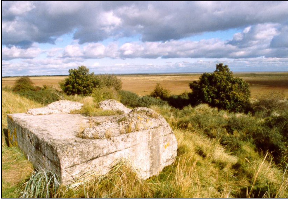
Fig. 4 - UORN 5131: pillbox dug into the sand dunes above Sea View, with concrete lumps on the roof to break up its outline.
