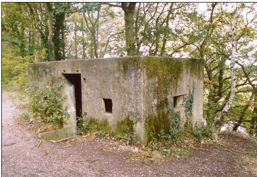
Fig. 3 - UORN 6255: type 24 pillbox, with a step down to its entrance, positioned on the slope of the canal bank overlooking the River Tame that is flowing on a parallel course beneath.
