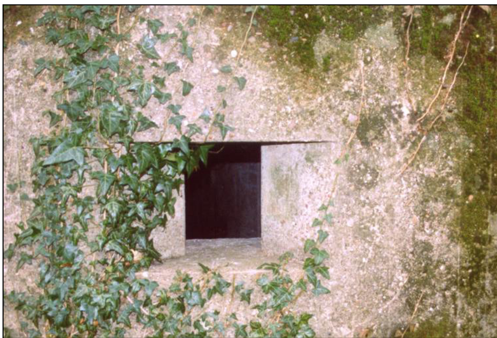
Fig. 4 - UORN 6255: detail of one of the pillbox's square, splayed embrasures.
