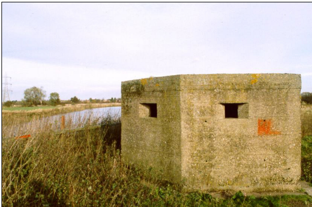
Fig. 6 - UORN 5335: type 24 pillbox, already suffering from some spray-can damage, which may be vulnerable to possible future development here.
