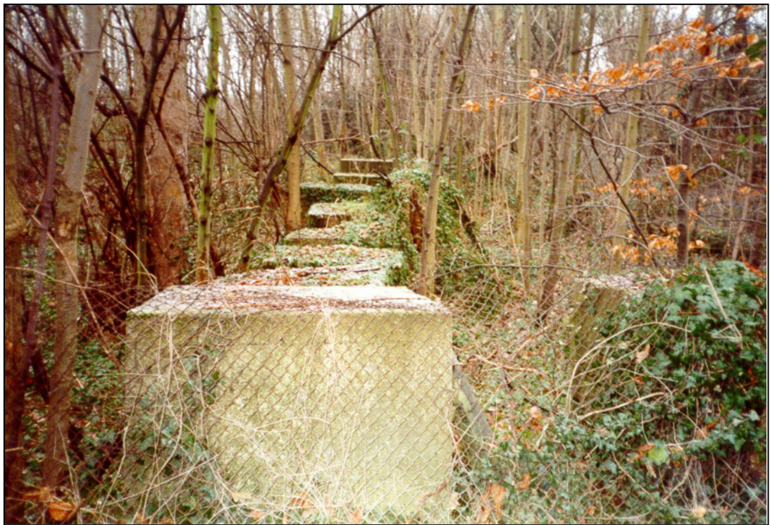
Fig. 8 - UORN 2645: anti-tank cubes, forming the front-edge anti-tank obstacle on the Outer London Anti-Tank Line, running through woodland east of the Drift Bridge.
