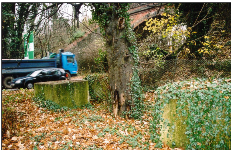
Fig. 9 - UORN 2644: the gap between the terminal of the anti-tank ditch and the road west of the Drift Bridge was blocked by anti-tank cubes. This was also the position of a roadblock.
