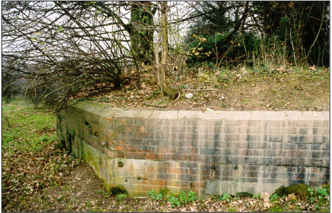
Fig. 6 - UORN 2642: this octagonal type 27 pillbox is now overgrown and partly buried, but, if cleared, would probably prove to be in relatively good condition.
