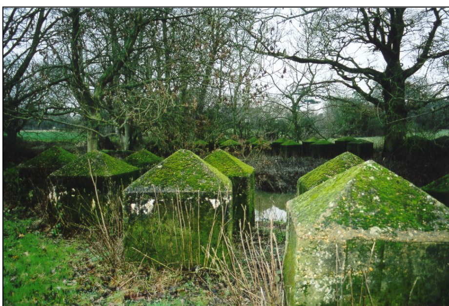
Fig. 8 - UORN 2455: anti-tank cubes strengthening the banks of the River Mole as an obstacle to enemy armoured vehicles.
