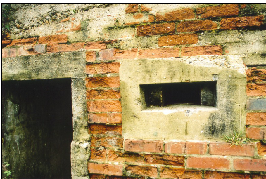
Fig. 7 - UORN 2477: an embrasure of a reinforced concrete, brick-shuttered pillbox.
