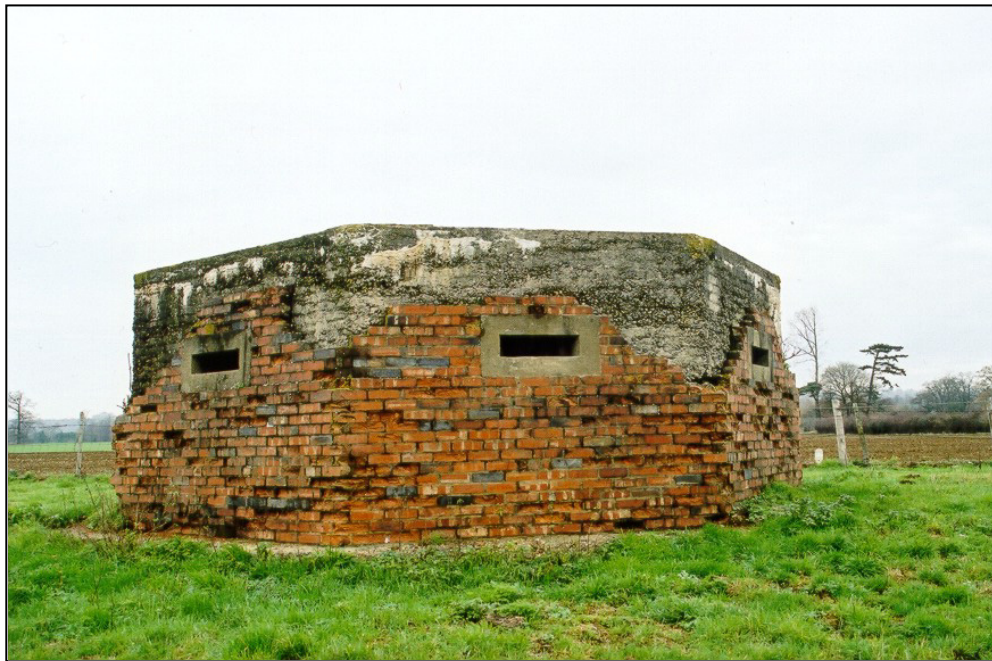
Fig. 5 - UORN 2476: type 24 infantry pillbox with large sections of brick shuttering apparently deliberately removed.
