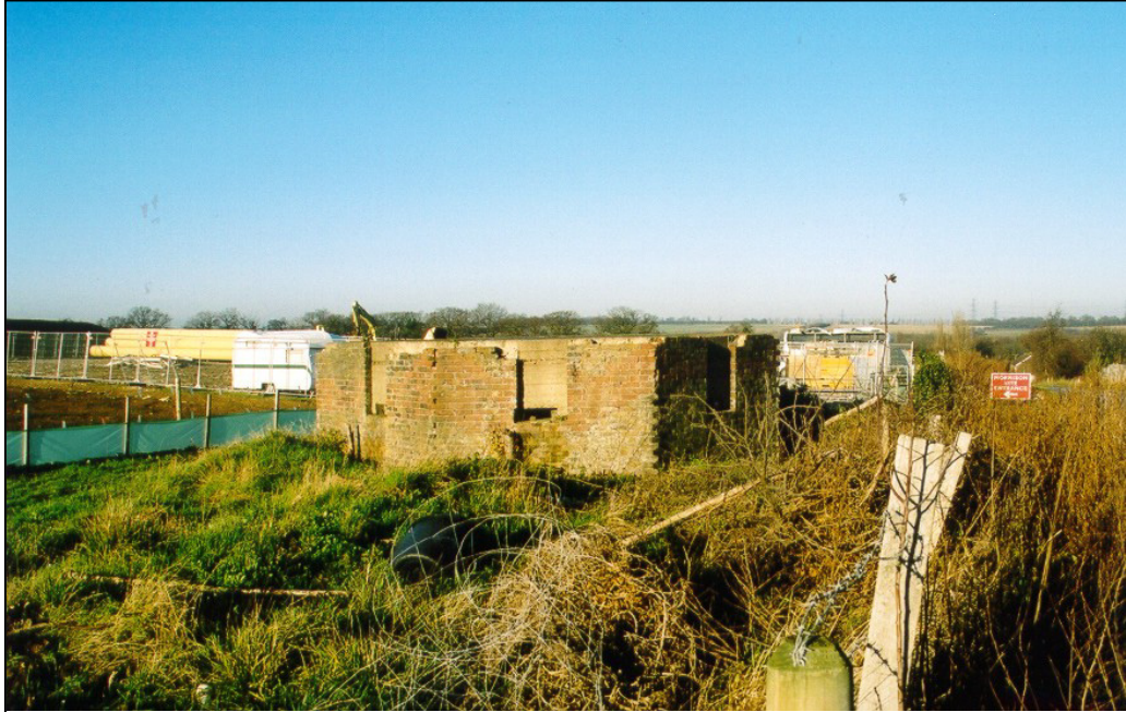
Fig. 7 - UORN 2706: type 24 infantry pillbox at the Deangate crossroads, showing the unusual 'cut outs' above the embrasures, a feature of pillboxes in this area. This pillbox will be destroyed in current road-works.
