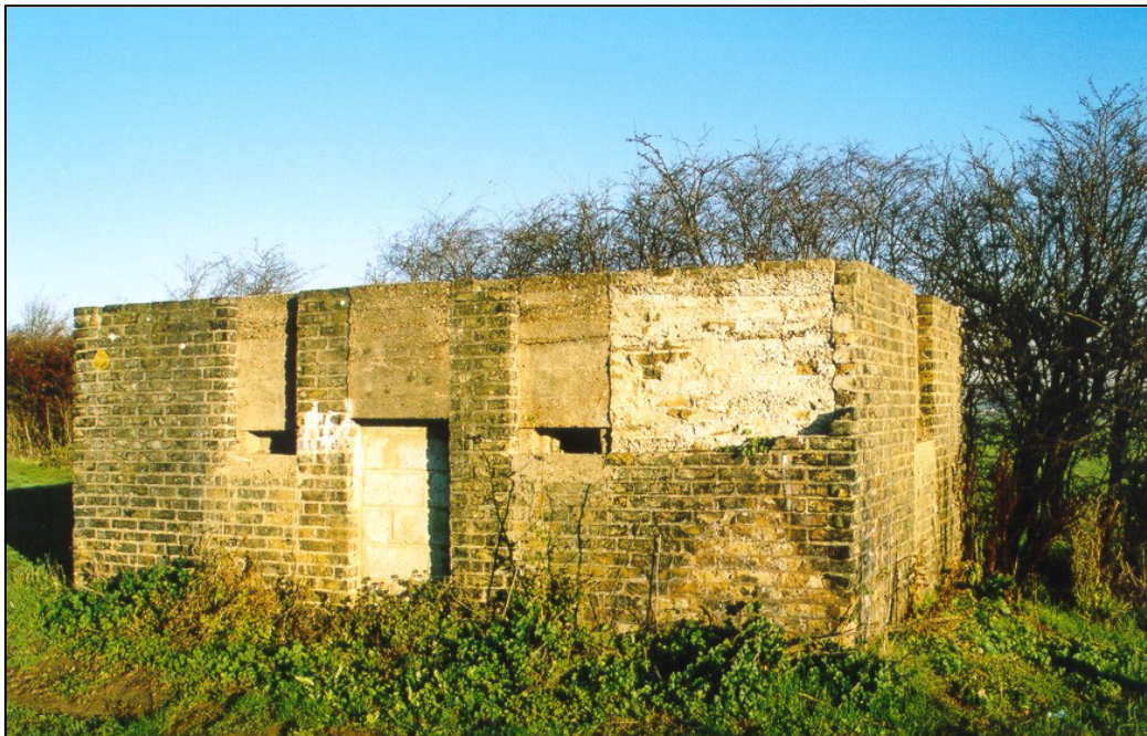
Fig. 8 - UORN 2672: type 24 infantry pillbox with its entrance now blocked up. It faced E across the anti-tank ditch which ran on the other side of the hedgerow.
