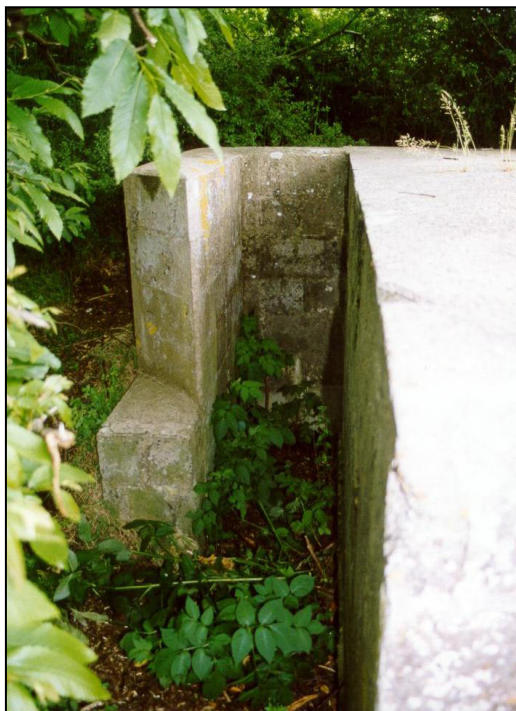
Fig. 5 - UORN 11782: a large pillbox made of concrete blocks, with an attached external blast wall and twin embrasures in each face (except that with the entrance) - sometimes termed a 'Suffolk square' type.
