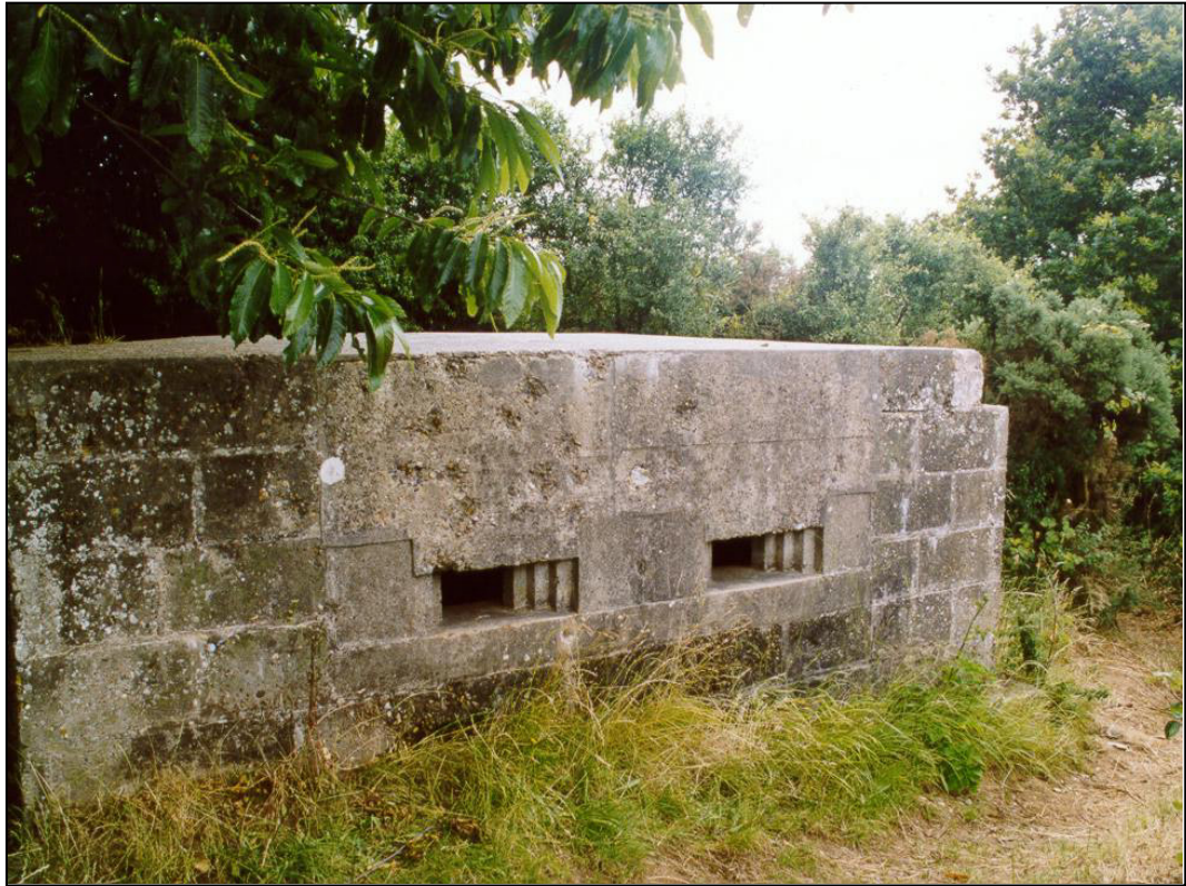
Fig. 5 - UORN 11782: a large pillbox made of concrete blocks, with an attached external blast wall and twin embrasures in each face (except that with the entrance) - sometimes termed a 'Suffolk square' type.
