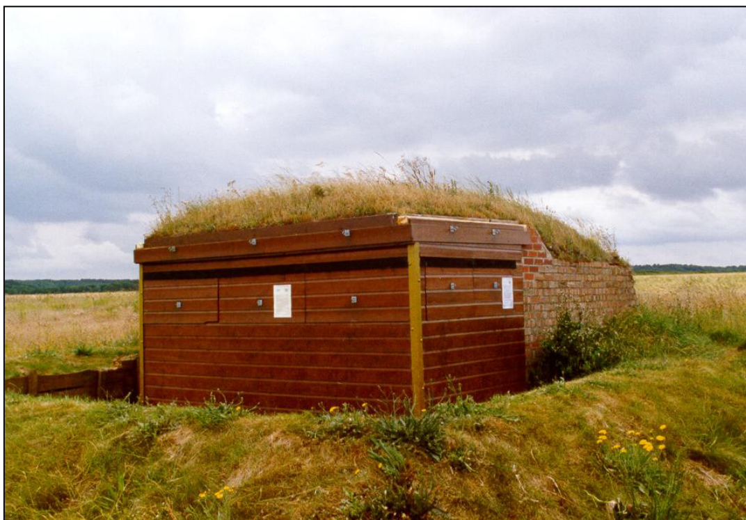
Fig. 16 - UORN 1054: rectangular pillbox converted in 1993 into a bird observatory. Although some conversion of Second World War defence works is acceptable, and even desirable for their future preservation, in this case the alterations have destroyed the integrity of the structure, which is now hard to interpret.
