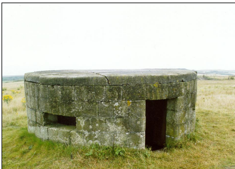
Fig. 3 - UORN 1057: First World War pillbox on land of the former army camp, now the Muckleburgh Collection military museum. It has an iron door still in place. In the Second World War it was sandbagged and used as an air raid shelter. The roof is now badly cracked and needs urgent conservation work.
