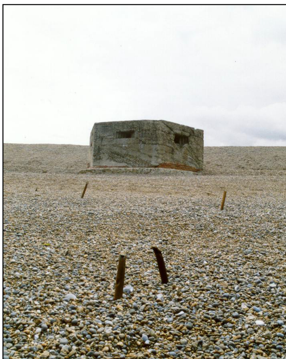
Fig. 9 - UORNs 1090 and 16122: remains of tubular beach scaffolding projecting from the shingle. The scaffolding ran in front of the pillbox and was added after it was built.
