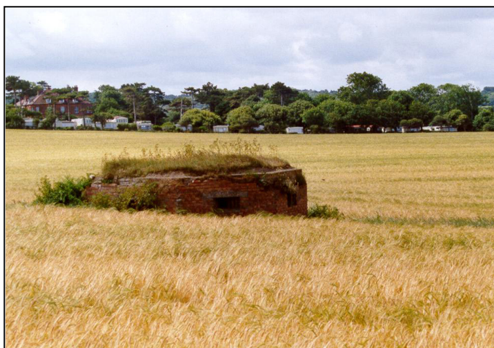
Fig. 13 - UORN 1068: emplacement for a Vickers medium machine gun, built to provide fire west across Weybourne Hope. It stands now on the very cliff edge, but was originally set some twenty feet back. Before long, it will follow at least two other pillboxes at this point that have fallen to the beach beneath.
