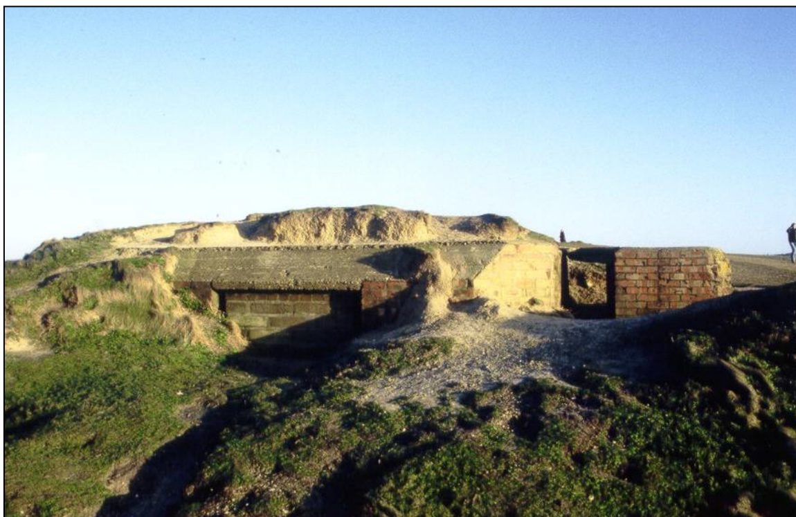
Fig. 13 - UORN 1068: emplacement for a Vickers medium machine gun, built to provide fire west across Weybourne Hope. It stands now on the very cliff edge, but was originally set some twenty feet back. Before long, it will follow at least two other pillboxes at this point that have fallen to the beach beneath.
