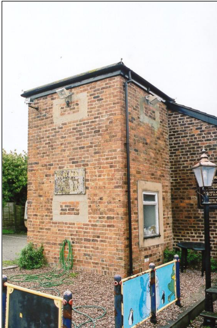
Fig. 6 - UORN 11732: loopholed tower attached to the Farmers Arms public house. The loopholes are at two levels.
