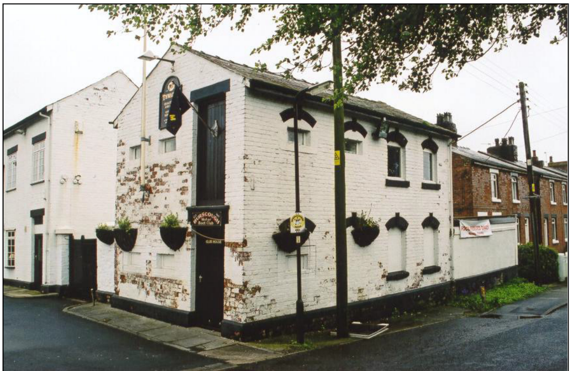
Fig. 5 - UORN 11731: loopholed former stables at The Slipway public house. The lower loopholes are now blocked, but the upper have been glazed.
