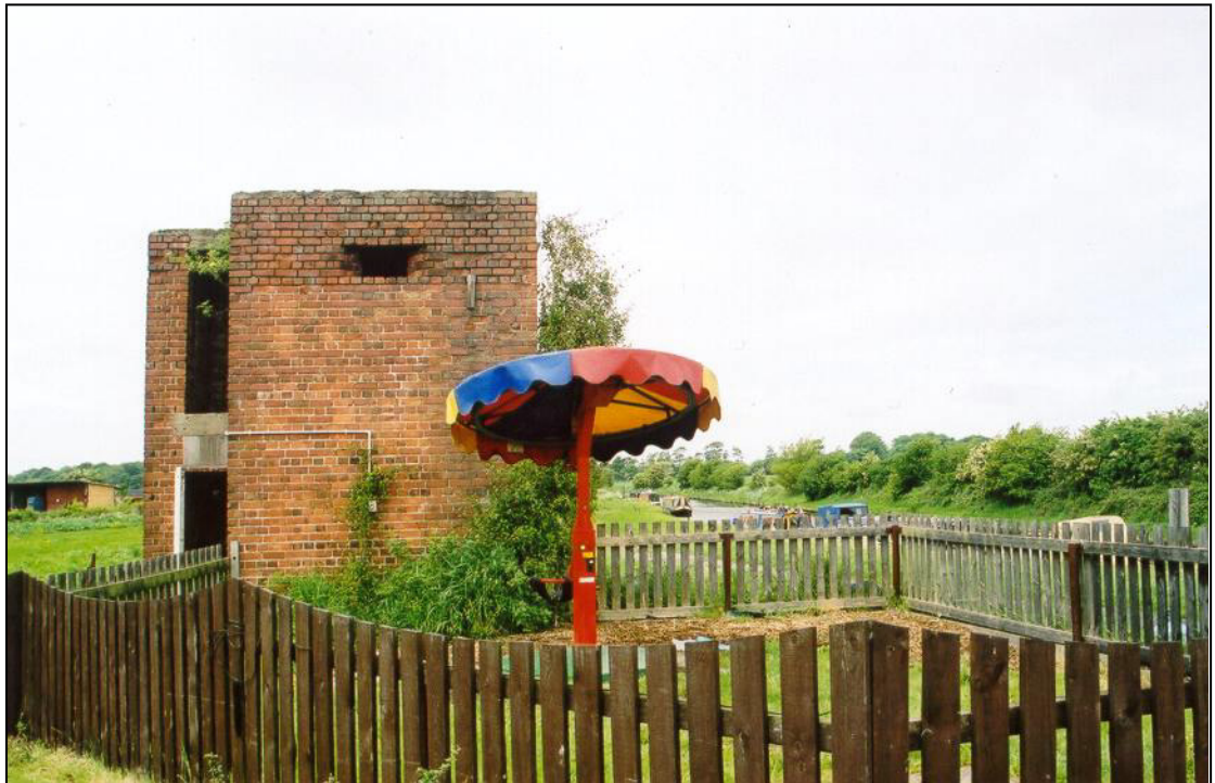
Fig. 10 - UORN 7807: a view showing the doorways at two levels; the upper must have been accessed by a ladder.
