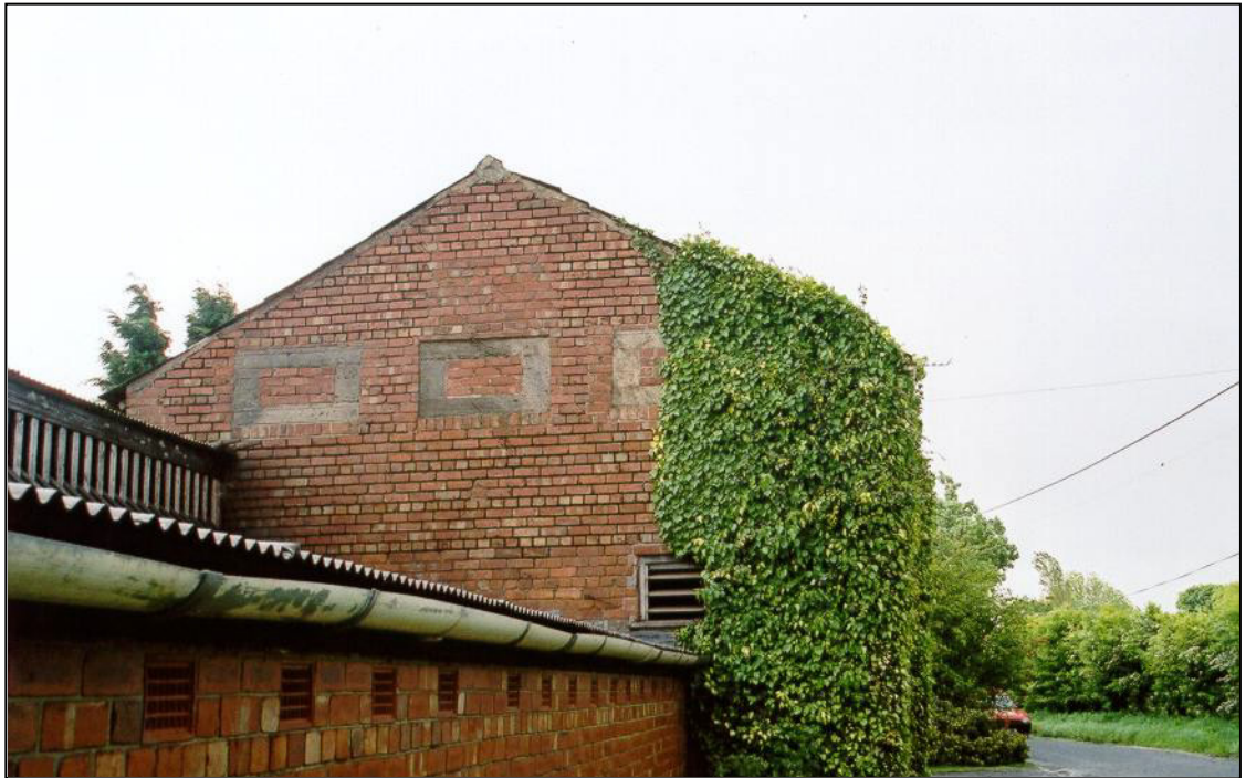
Fig. 8 - UORN 7805: an outbuilding of Gregsons Bridge Farm loopholed for defence. Other loopholes may be hidden by the ivy.
