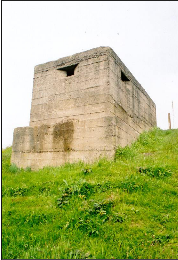
Fig. 9 - UORN 16618: type 23 pillbox set on a thick concrete base on the side of a former railway cutting.
