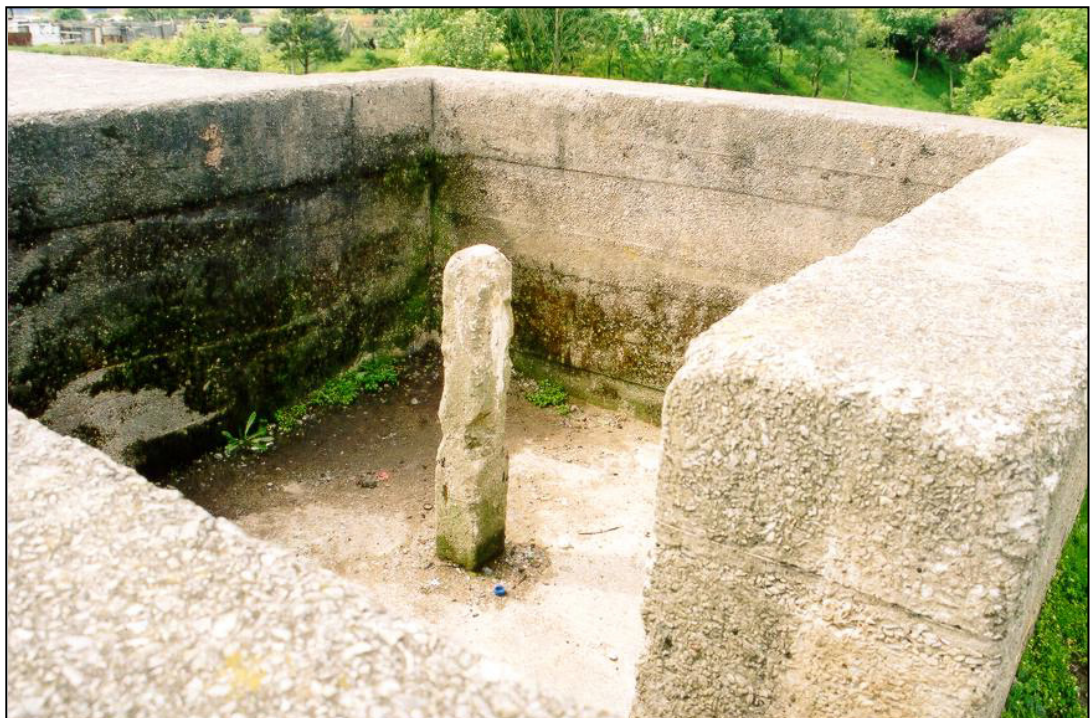
Fig. 10 - UORN 16618: the anti-aircraft gun mount in the open bay attached to the pillbox.
