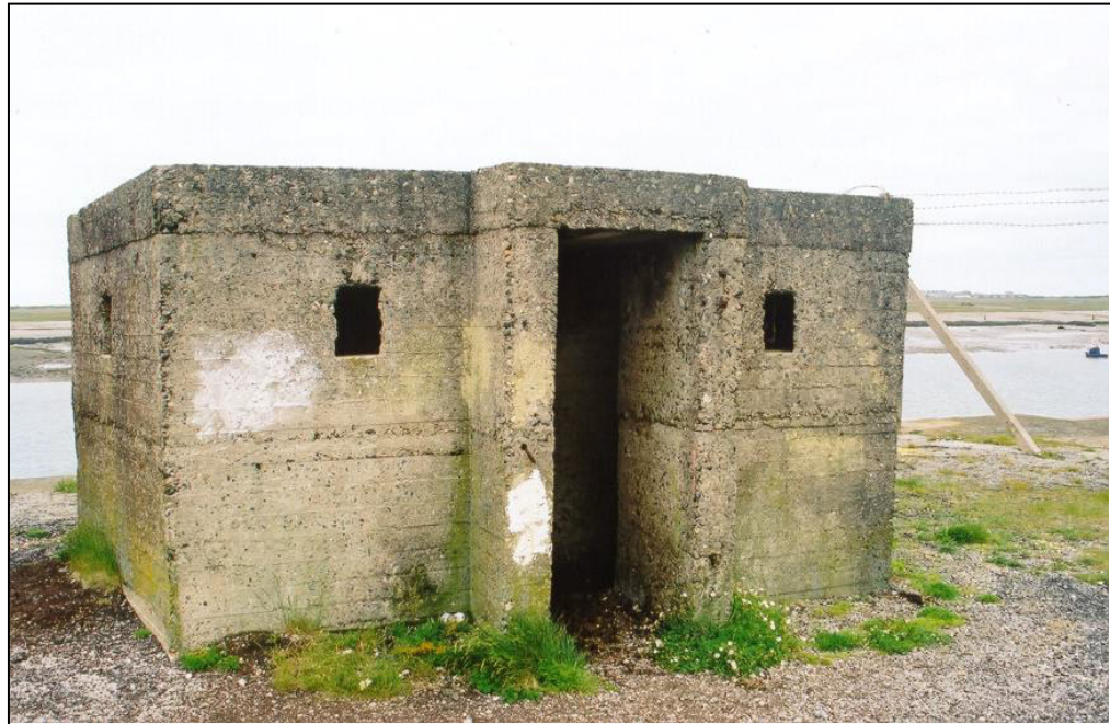
Fig. 4 - UORN 16490: type 24 pillbox at the edge of the Walney Channel, showing the unusual projecting doorway.
