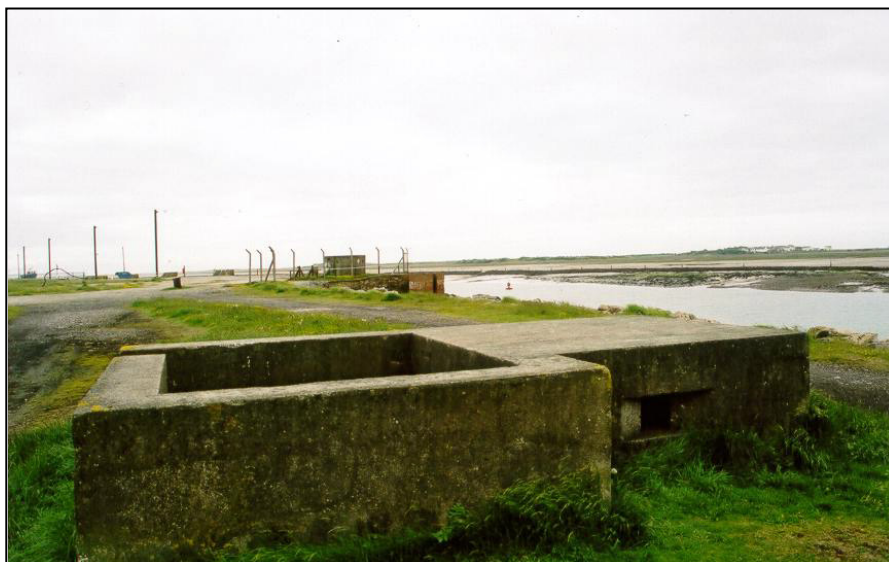
Fig. 8 - UORN 16617: type 23 pillbox with open anti-aircraft bay.
