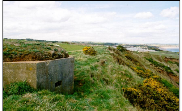
Figs. 6 and 7 - UORNs 2776 [left] and 2807 [right]. Excellent examples of the local lozenge-shaped variant of an infantry pillbox, the latter well dug in and positioned to enfilade the cliff top to the east.
