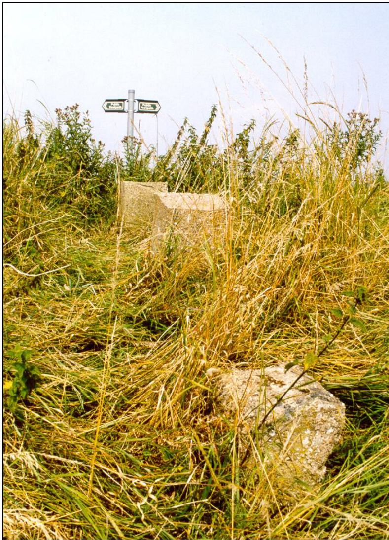
Fig. 3 - UORN 5204: still in place across the sea bank, these are probably the country's smallest concrete cubes having a role in the 1940 anti-invasion defences.
