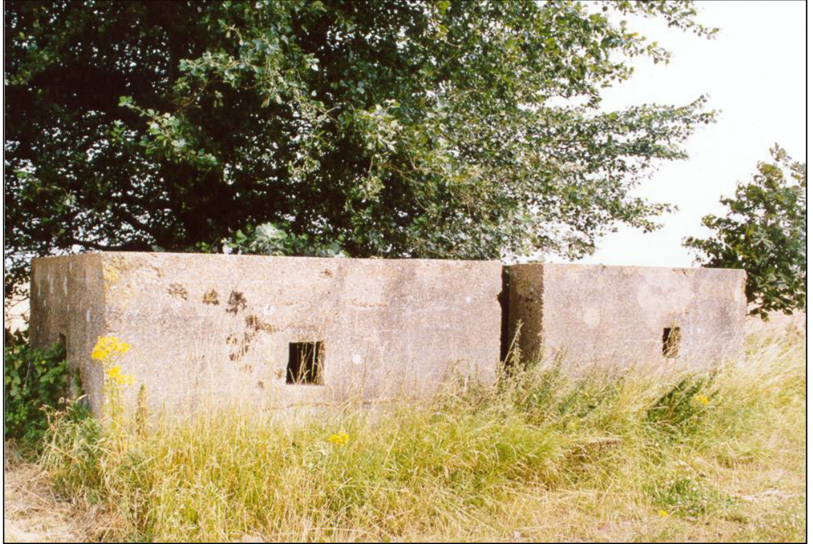
Fig. 4 - UORN 5203: Lincolnshire-type pillbox, with two chambers separated by an open bay for anti-aircraft fire.
