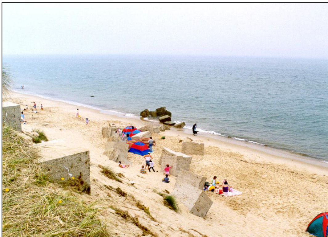
Fig. 6 - UORN 9102: anti-tank cubes toppled down the eroded sand dunes. At the time of the Second World War, the sea's edge was some 20 metres further out. A pillbox, and lines of barbed wire and tubular scaffolding, once stood where there is now open water.
