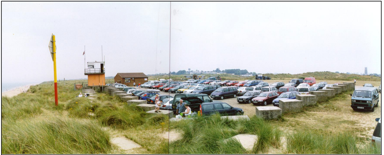
Fig. 5 - UORN 9102: the lines of anti-tank blocks, now the site of the beach car park. The coastguard lookout hut is set on stilts resting on the blocks. Many blocks are now buried deep in the sand, and, to the left of the picture, they have tumbled onto the beach.
