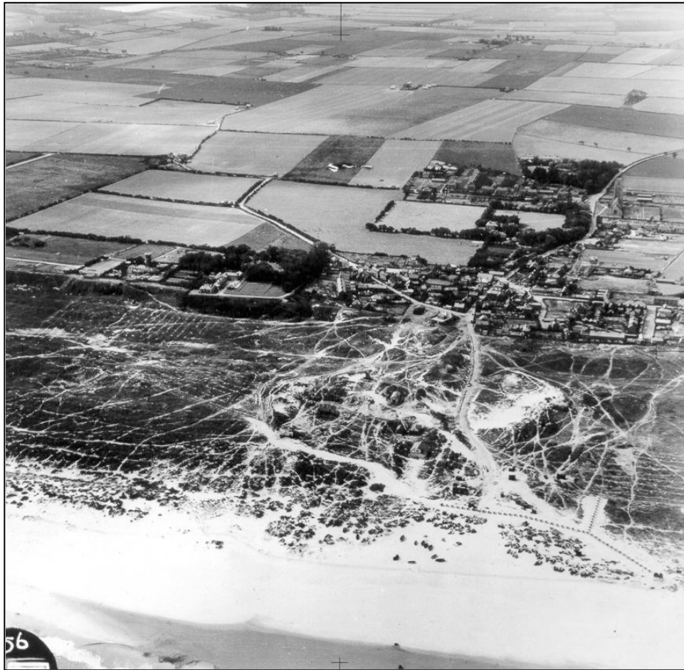
Fig. 8 - The single lines of anti-tank blocks as further developed by 19 Sept. 1940 .
