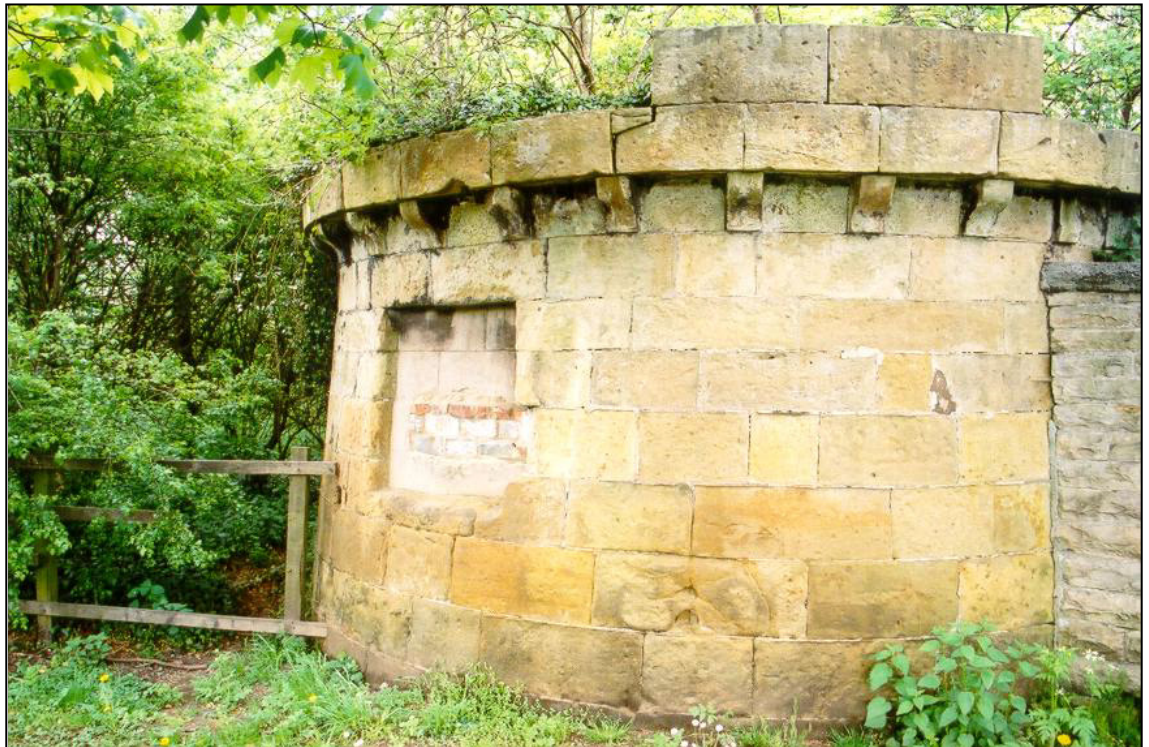
Fig. 6 - UORN 10148 - 18th century drum tower pierced for defence in 1940. The loophole has been crudely blocked in.
