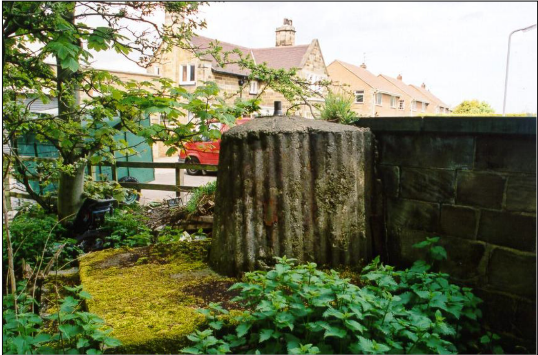
Fig. 7 - UORN 10722: spigot mortar pedestal by the perimeter wall at the eastern end of Kirkleatham Hall grounds, positioned so that the weapon could fire over the wall across open fields now occupied by housing. The pedestal was constructed with corrugated iron shuttering.
