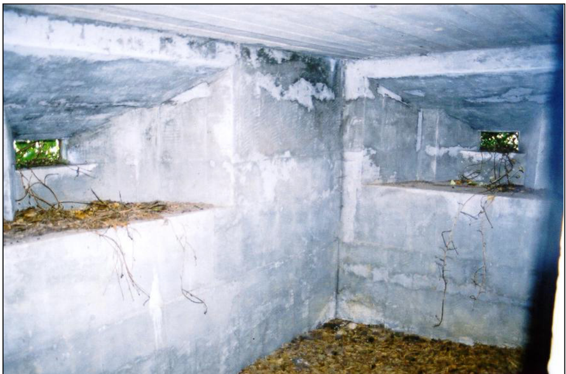
Fig. 9 - Interior of anti-tank gun emplacement, UORN 11971, showing its LMG chamber.
