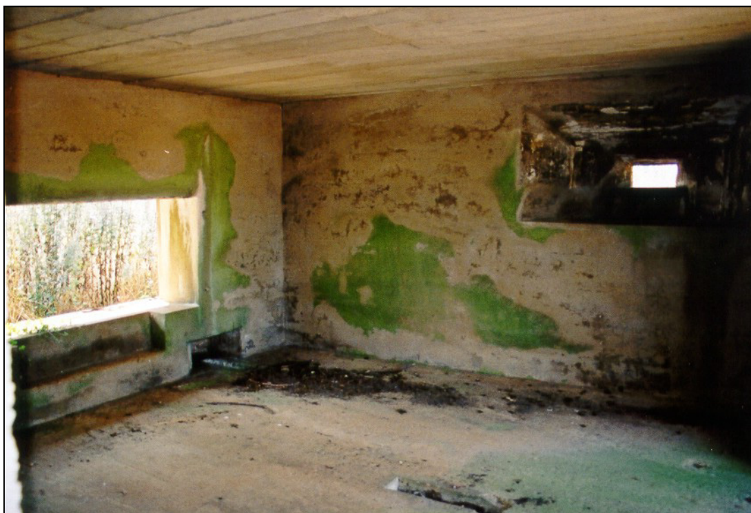
Fig. 6 - The interior of anti-tank gun emplacement, UORN 11973. The slot in the floor is to take the trail of the 2pdr. anti-tank gun. This structure is in excellent, clean condition, although it is doubtful if the green paint is original.
