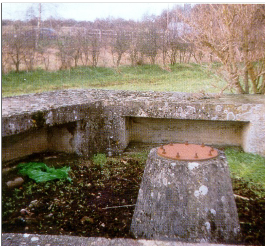
Fig. 11 - UORN 7200: 6pdr. gun pit, with central pedestal and holdfast to mount the swivelling Hotchkiss 'QF' gun. Lockers for ammunition surround the emplacement.
