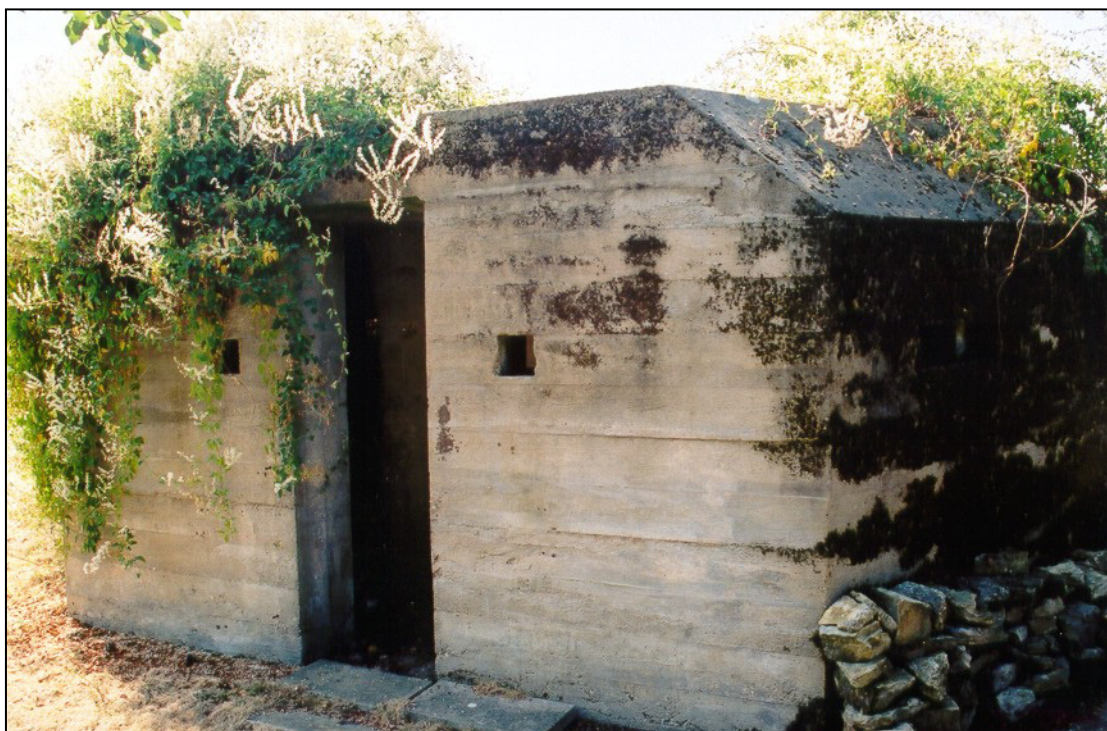
Fig. 12 - UORN 11974: type 22 pillbox strengthened to withstand shell fire. The roof has chamfered edges, a feature found usually on heavier emplacements.
