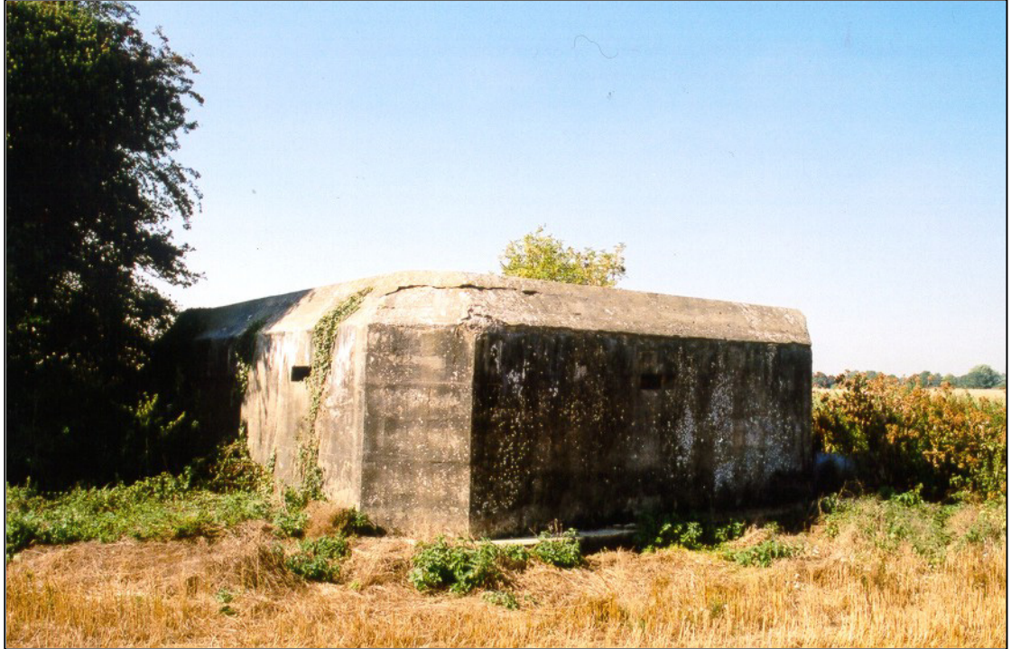
Fig. 8 - UORN 11972: this type 28A anti-tank gun emplacement is in relatively good condition, with only a small amount of interior graffiti. As it stands by a public footpath, it can easily be inspected.
