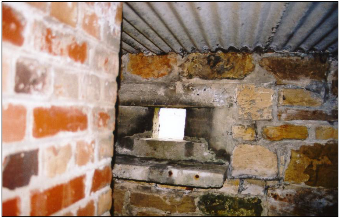
Fig. 9 - UORN 7011: the interior showing a brick anti-ricochet wall, an embrasure with concrete shelf, and a reinforced concrete roof made with corrugated-iron shuttering.
