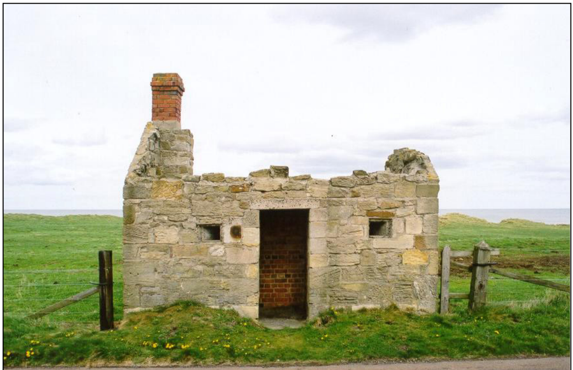
Fig. 8 - UORN 7011: pillbox disguised as a ruined cottage. The pillbox has not been inserted in a pre-existing building, but has been purpose-built with its disguised exterior.
