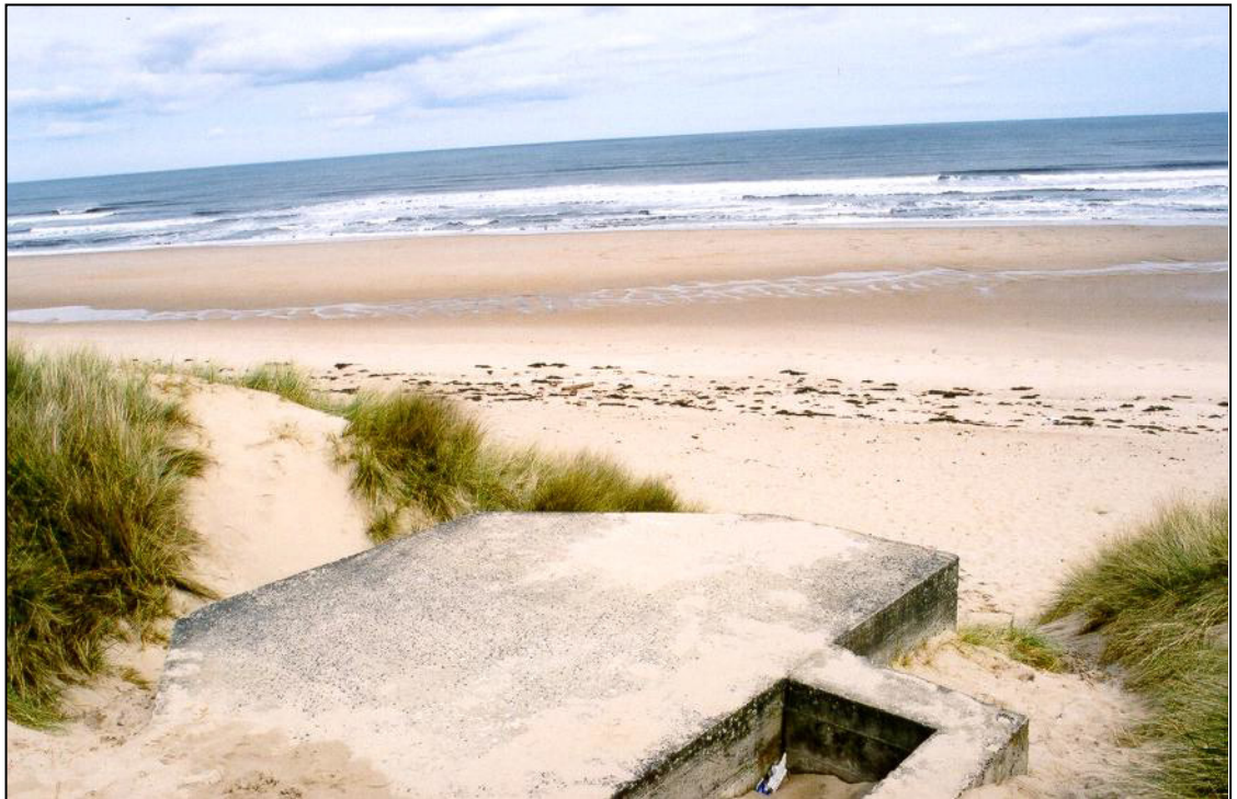
Fig. 7 - UORN 7135: hexagonal infantry pillbox with protected entrance positioned to enfilade the beach with its fire.
