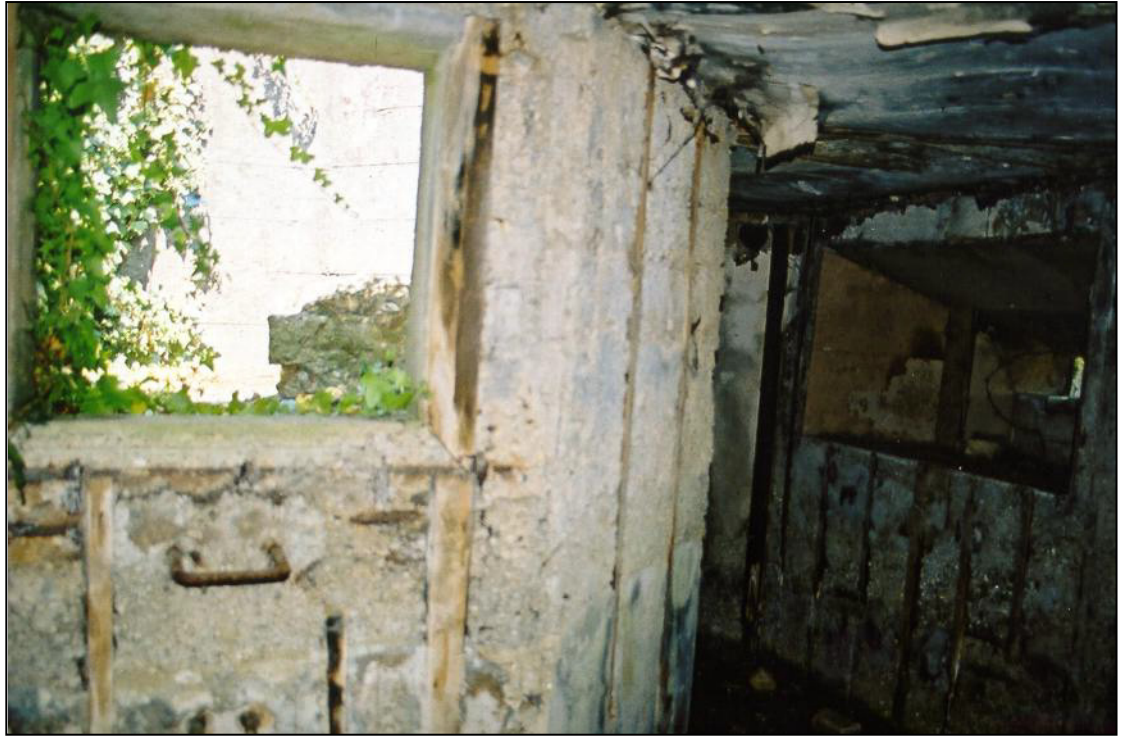
Fig. 5 - UORN 5065: the interior of a type 27 pillbox showing the access to the central well for anti-aircraft fire.
