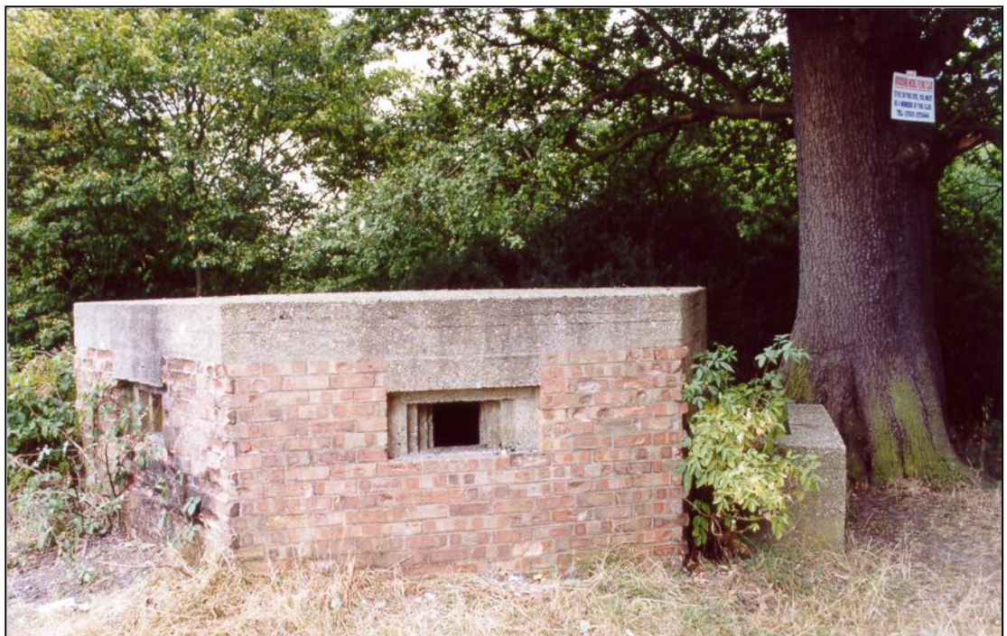
Fig. 8 - UORN 584: type 22 pillbox in Cheshunt Park with good examples of stepped embrasures and a low entry porch.. It has been damaged recently by a fire being lit against it, and the interior is littered with rubbish.
