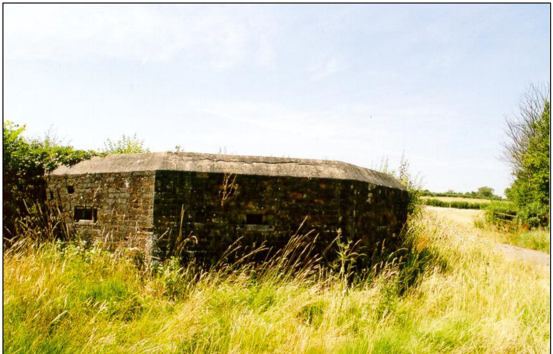
Fig. 6 - UORN 5065: exterior of a type 27 pillbox. The anti-tank ditch ran across its front.
