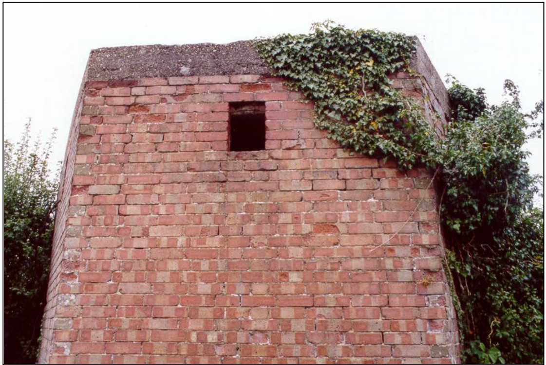
Fig. 7 - UORN 5061: unusual heightened type 22 pillbox facing east across Bread and Cheese Lane. The embrasures are of the rarer vertical pattern, i.e. higher than they are wide.
