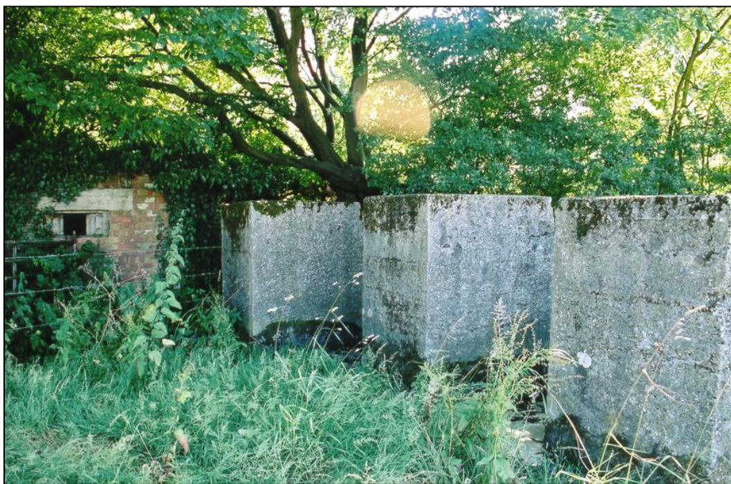
Fig. 9 - UORN 16689: three cubes strengthening the anti-tank obstacle, overlooked by type 22 pillbox, UORN 5062.
