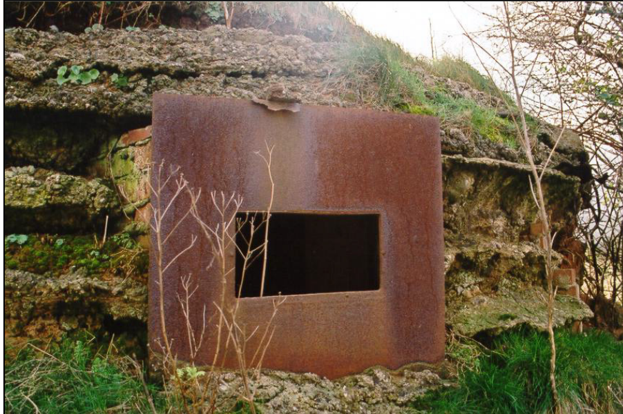
Fig. 11 - UORN 424: a steel embrasure surround is still in place on this pillbox.
