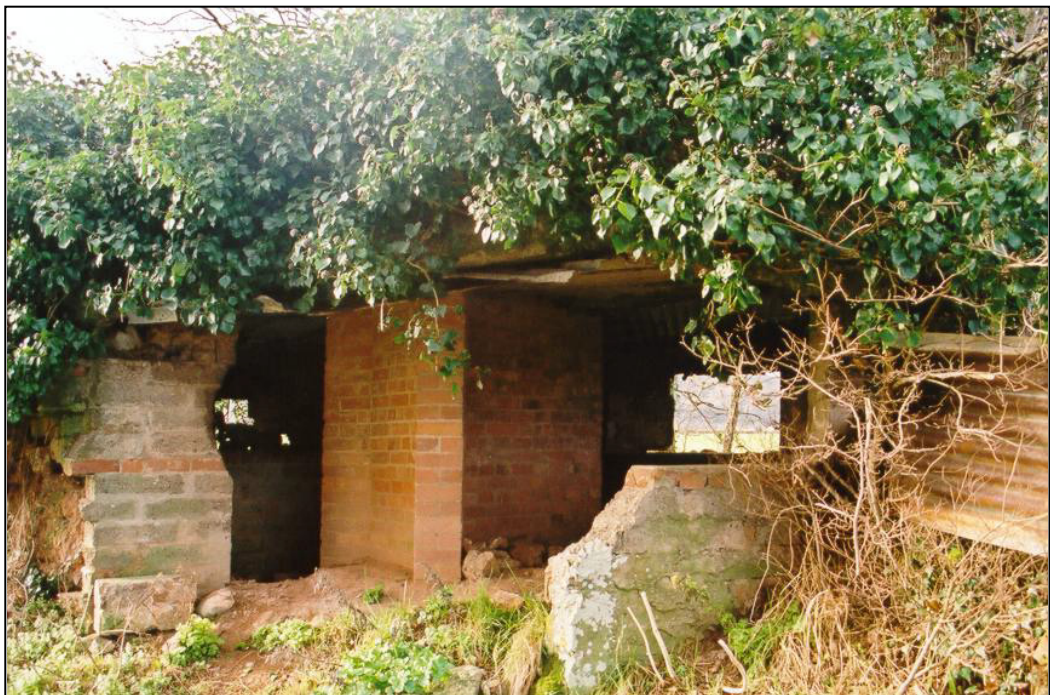
Fig. 10 - UORN 1563: remains of a type 24 pillbox, instructive in showing the method of construction and the different building materials.
