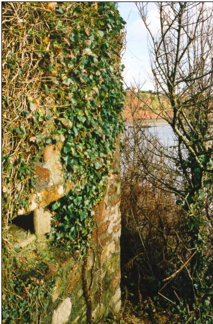
Fig. 5 - UORN 1394: an hexagonal pillbox faced with the local sandstone. Its small embrasures overlook Hollicombe Beach and the waters of Tor Bay.
