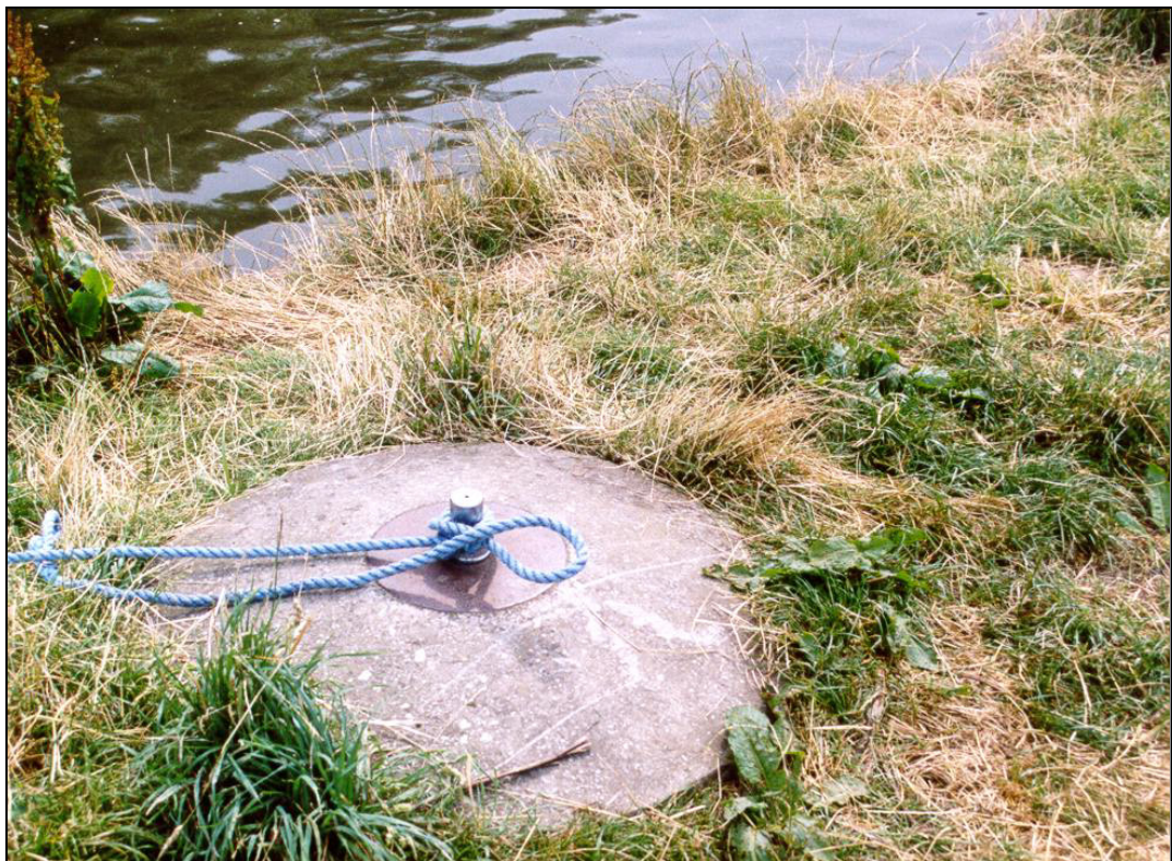
Fig. 1 - UORN 15768: the top of a spigot mortar pedestal used today as a boat mooring.
