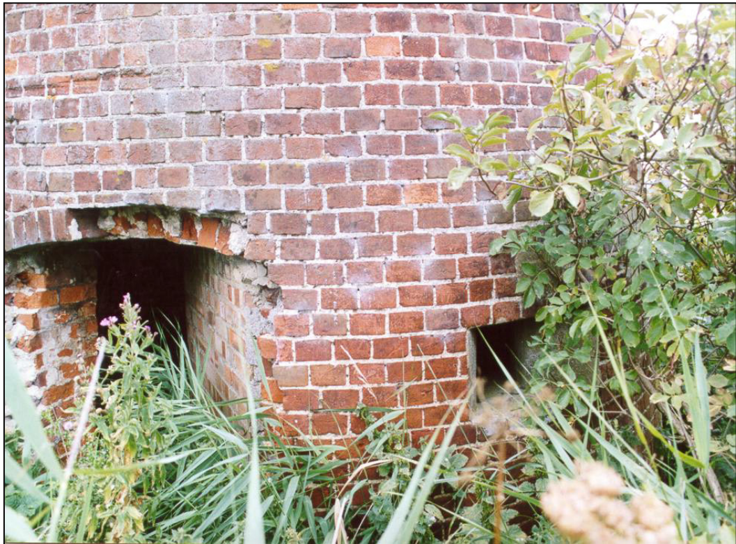
Fig. 4 - UORN 2348: the entrance to the tower protected by an angled blast wall and a loophole. A spigot mortar emplacement stands close to the entrance [UORN 2347]. The site is very overgrown.
