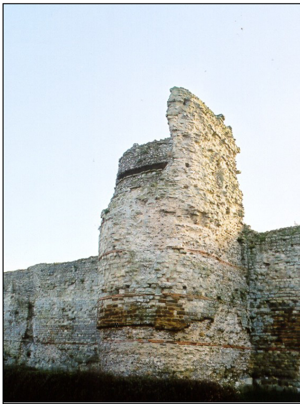
Fig. 13 - UORN 1511: machine gun emplacement erected within a medieval tower built on top of a Roman bastion.
