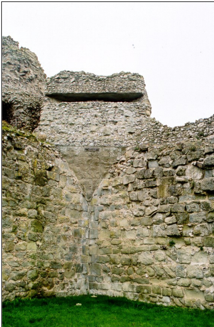
Fig. 7 - UORN 1512: machine gun emplacement constructed to look like the medieval masonry of the keep and firing through two horizontal embrasures to east and west. The long, narrow embrasures are a feature of the Castle defences, and are a rare type for machine gun fire also found in emplacements at Rye.
