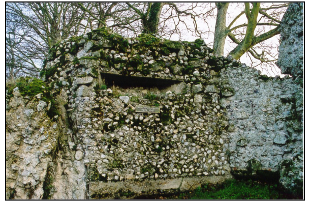
Fig. 11 (left) - UORN 1506: machine gun emplacement built amongst fallen masonry south of the Roman west gate.
