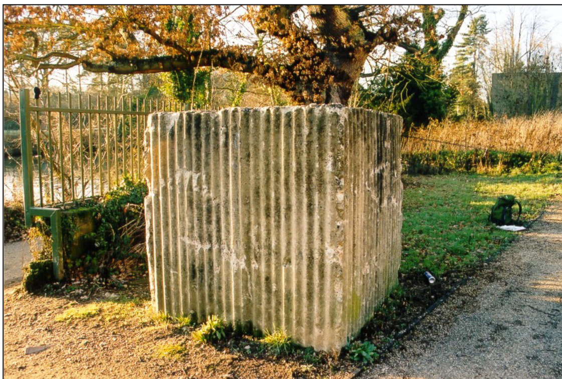
Fig. 11 - UORN 9509: one of the anti-tank cubes showing it was constructed using corrugated iron for shuttering. It has a height of nearly six feet.
