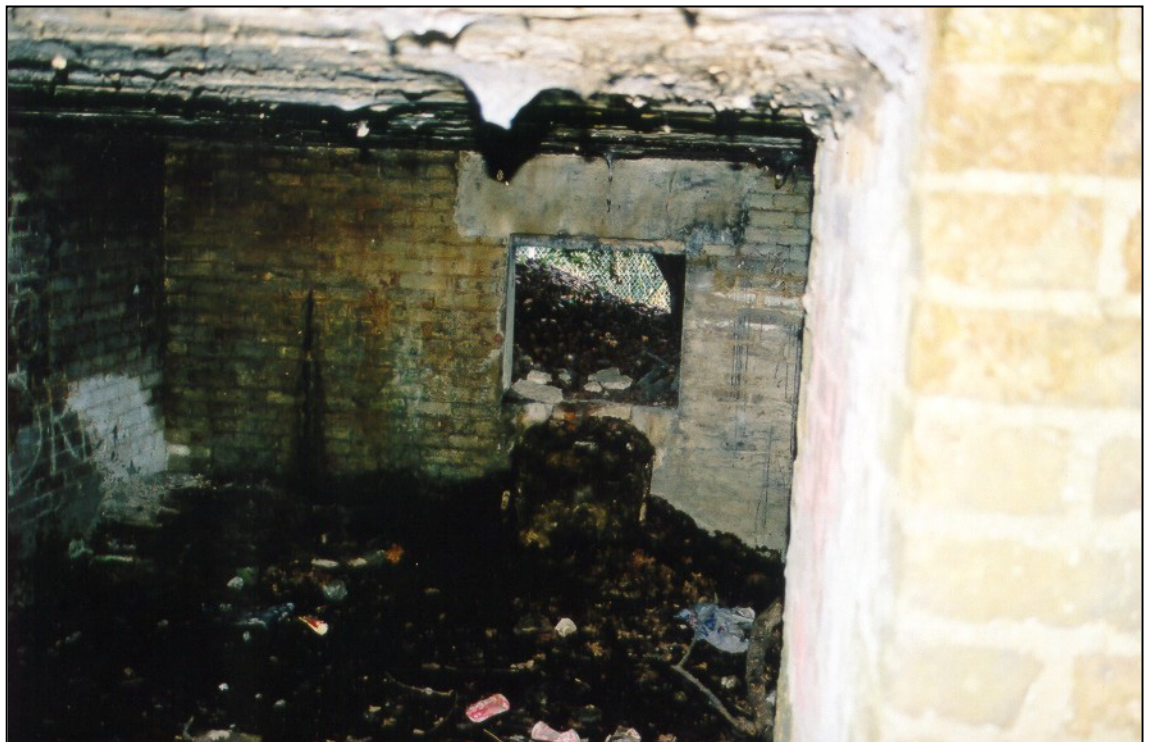
Fig. 6 - UORN 9513: much neglected anti-tank gun emplacement standing now on waste land close to the M20. The holdfast for a 6pdr. gun can be made out in front of the square embrasure.
