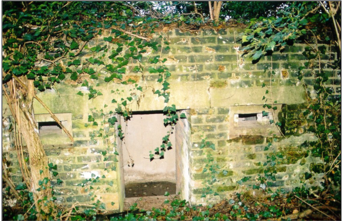
Fig. 7 - UORN 16798: rear face of brick-shuttered type 24 pillbox previously unrecorded.
