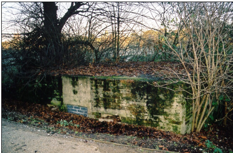
Fig. 7 - UORN 16798: rear face of brick-shuttered type 24 pillbox previously unrecorded.
