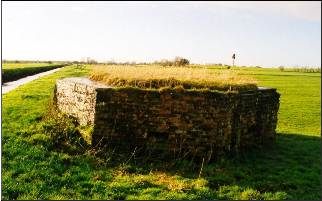
Fig. 8 - UORN 2994: a type 24 infantry pillbox stands on the north bank of the Division Rhyne, which at this point provides the main anti-tank obstacle for GHQ Line Green.
