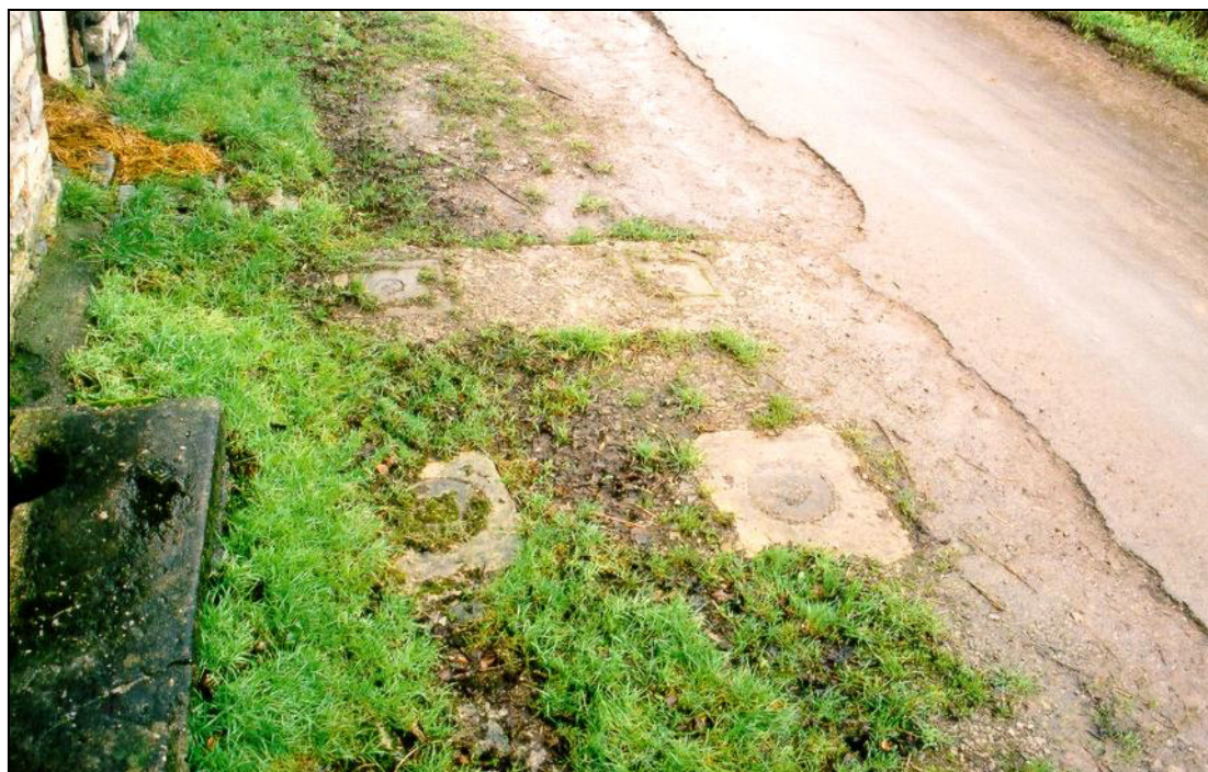
Fig. 7 - UORN 15669: concrete sockets to take upright steel rails mark the site of a roadblock. More sockets probably survive under the grass.
