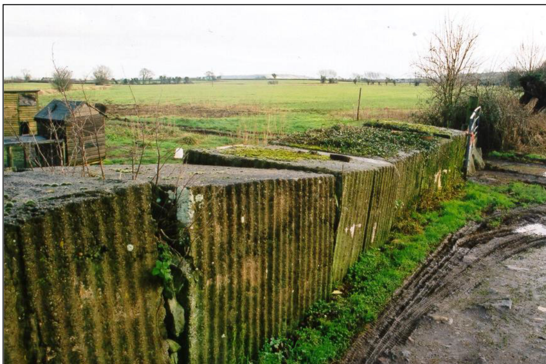
Fig. 6 - UORN 13973: anti-tank cubes lined up at Higher Bridge Farm, not far from their original situation. It is clear that they were made using corrugated-iron shuttering at the sides.
