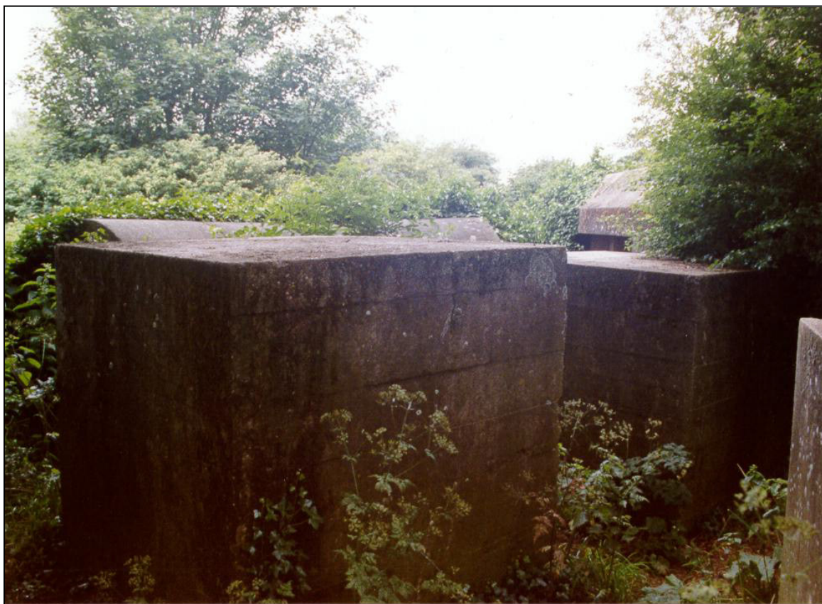
Fig. 4 - UORN 16085: concrete cubes with cylinders behind that form two lines of obstacles on the east side of the viaduct.
