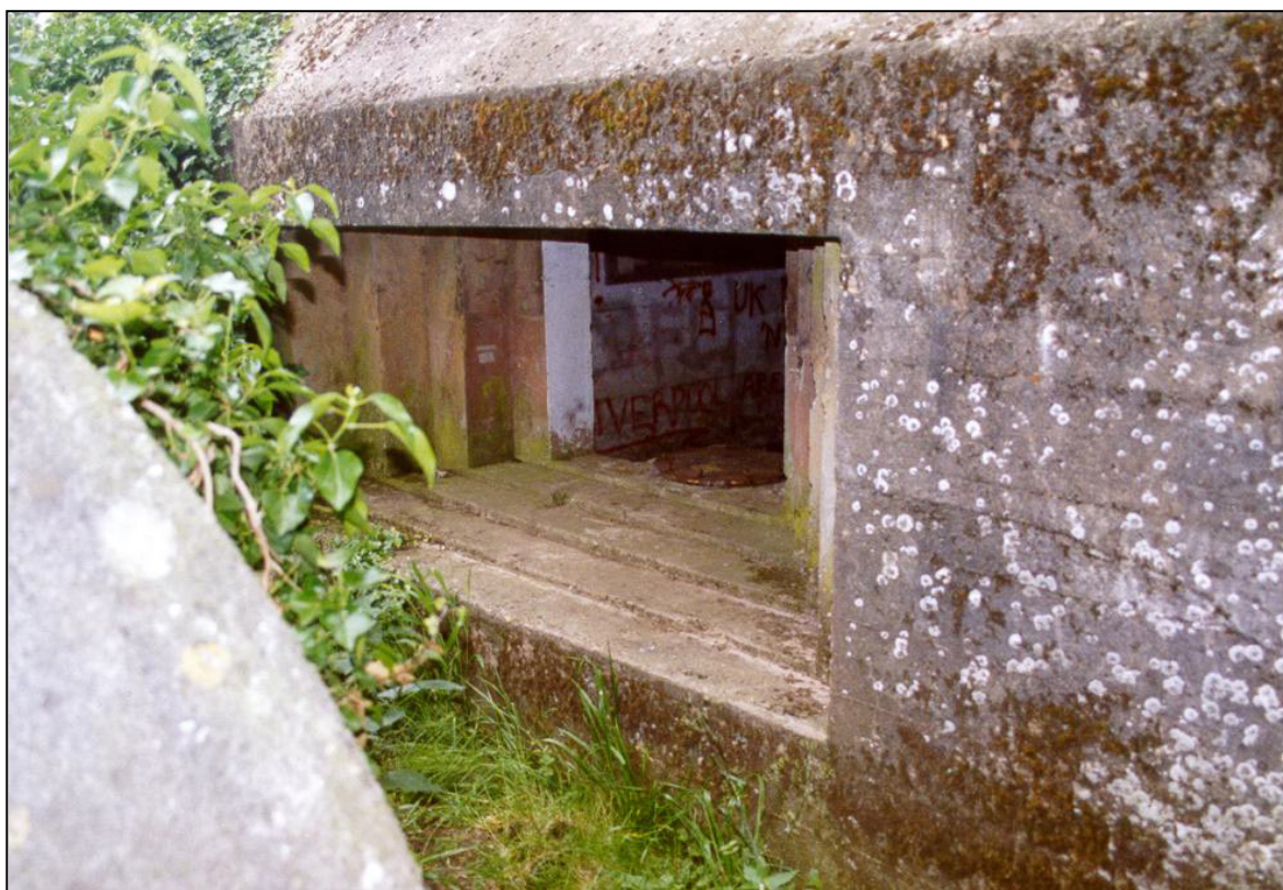
Fig. 5 - UORN 15696: the main embrasure of the type 28 anti-tank gun emplacement.
