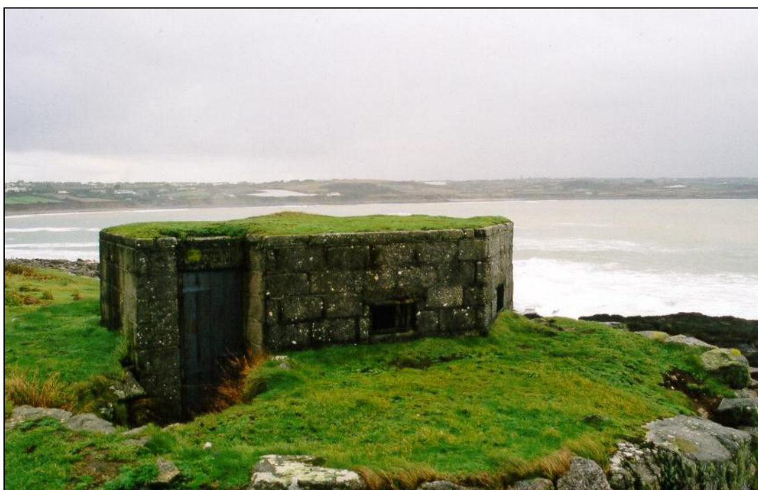
Fig. 7 - UORN 150: hexagonal pillbox, with attached blast wall and entrance porch, facing east across Mount's Bay from St. Michael's Mount.
