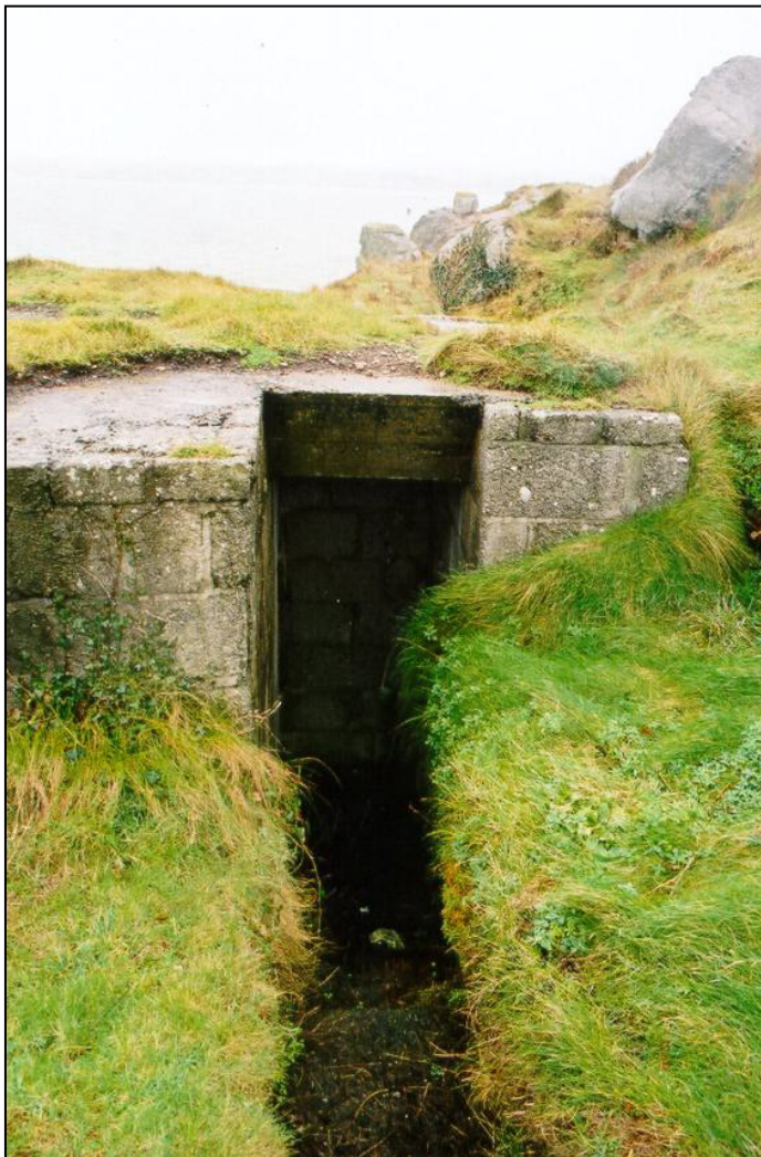
Fig. 9 - UORN 151, showing the sunken entrance way protected by a blast wall attached to the pillbox.
