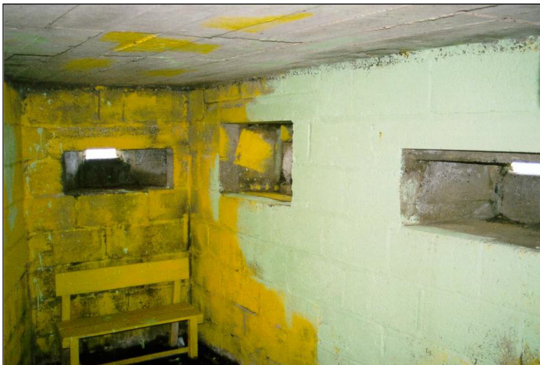
Fig. 11 - The interior of UORN 153, showing the small, splayed embrasures. The pillbox has been used as a play area by local children.
