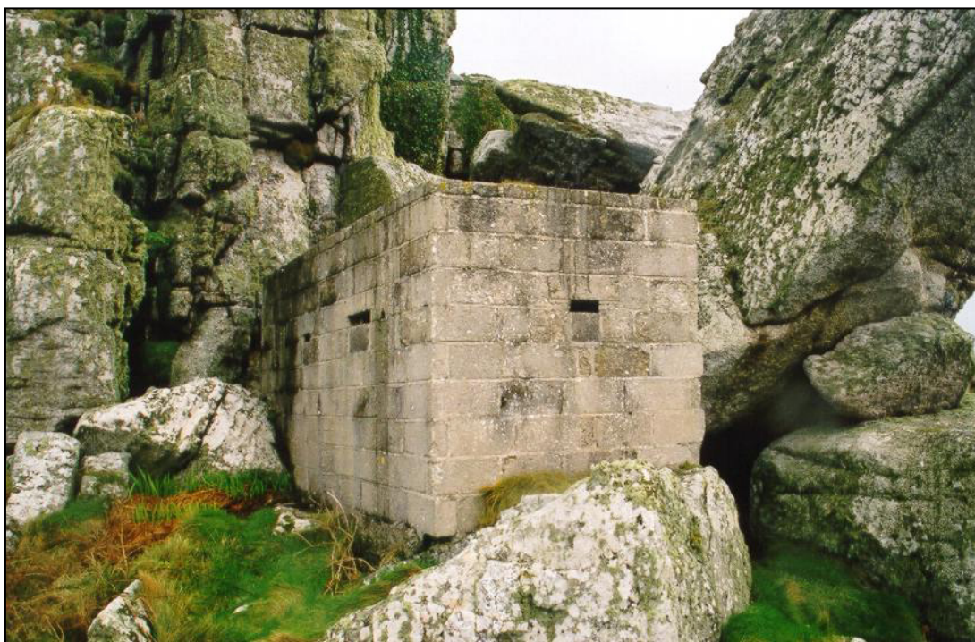
Fig. 10 - UORN 153: trapezoidal-shaped pillbox built to fit in a cleft in the rocks. It is made of concrete blocks and has very small embrasures. The entrance at the rear can be accessed with difficulty through a narrow gap in the rocks.
