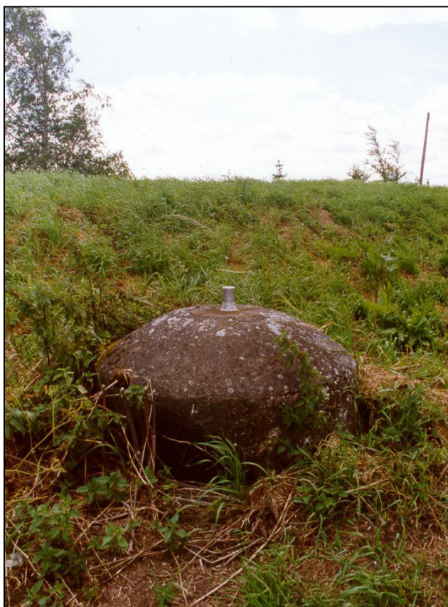
Fig. 6 - UORN 4699: spigot mortar pedestal south-west of Littleport Bridge, dug into the embankment of the River Great Ouse.
