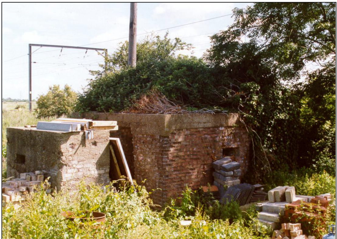
Fig. 3 - UORN 4697: Square 'Eastern Command-type' pillbox, with detached loopholed blast wall. It survives in poor condition behind houses in Victoria Street.
