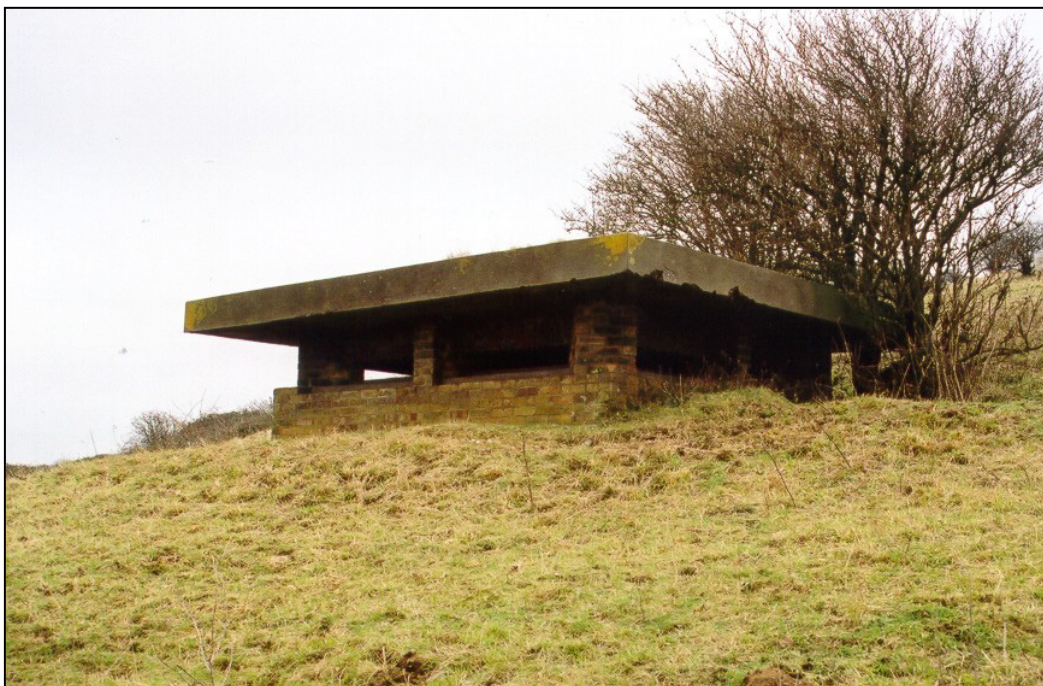
Fig. 6 - UORN 967: example of the 'Dover' variant' pillbox with its overhanging roof slab. Large open embrasures provide good all-round visibility but would have been highly vulnerable to incoming fire.
