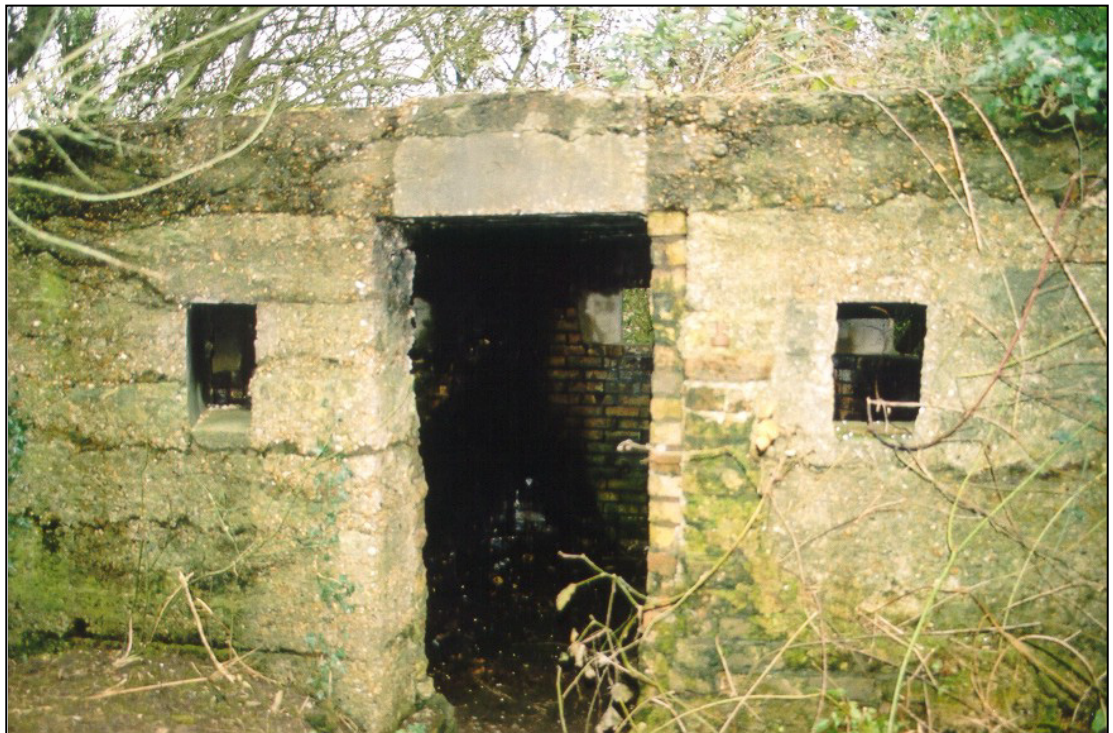
Fig. 10 - UORN 964: the entrance to this type 24 pillbox, showing splayed rifle ports on either side. The interior anti-ricochet wall has been removed, probably so that the structure can be used as a sheep shelter.
