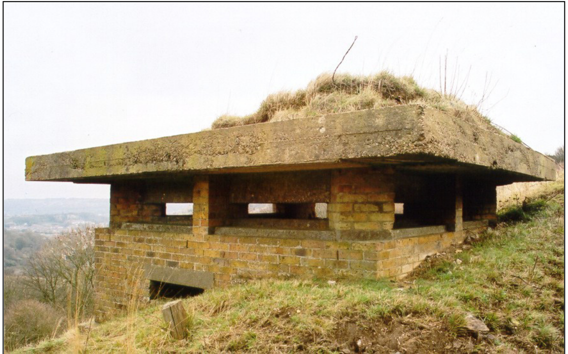
Fig. 7 - UORN 14814: taking advantage of the steep slope on which it was built, this 'Dover variant' type pillbox has an additional lower level embrasure. The pillbox type has distinctive brick corner supports for the roof turned at an angle to the rest of the square structure.
