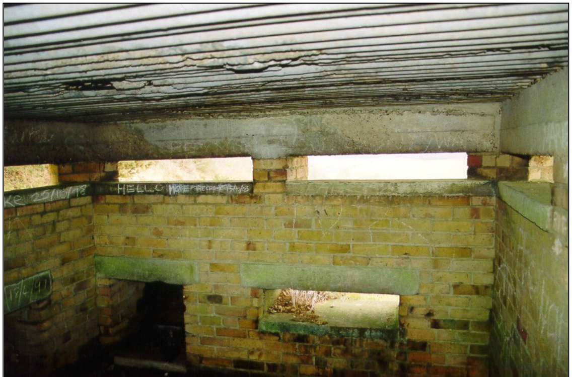
Fig. 8 - UORN 14814: the view from inside firing north towards Farthingloe. The lower level embrasure can be seen.
