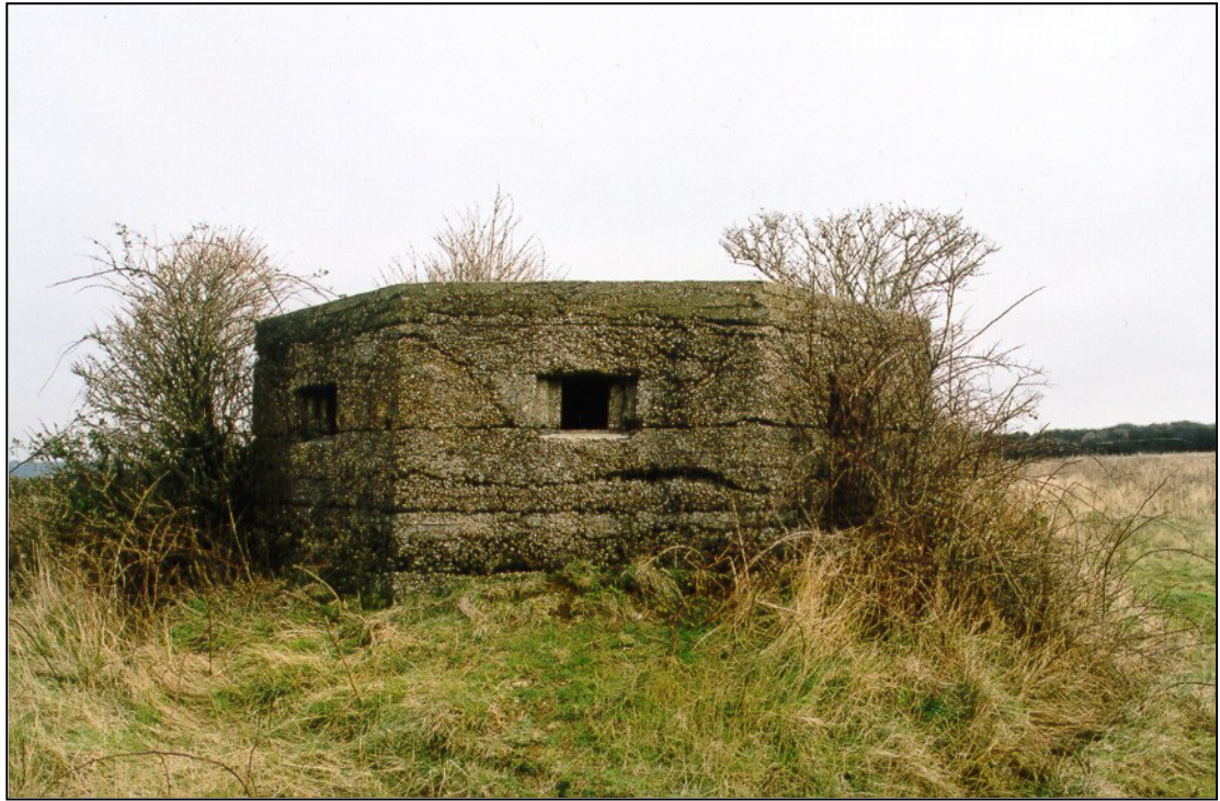
Fig. 9 - UORN 962: type 24 pillbox on Coney Hill, denuded of its outer brick shuttering.
