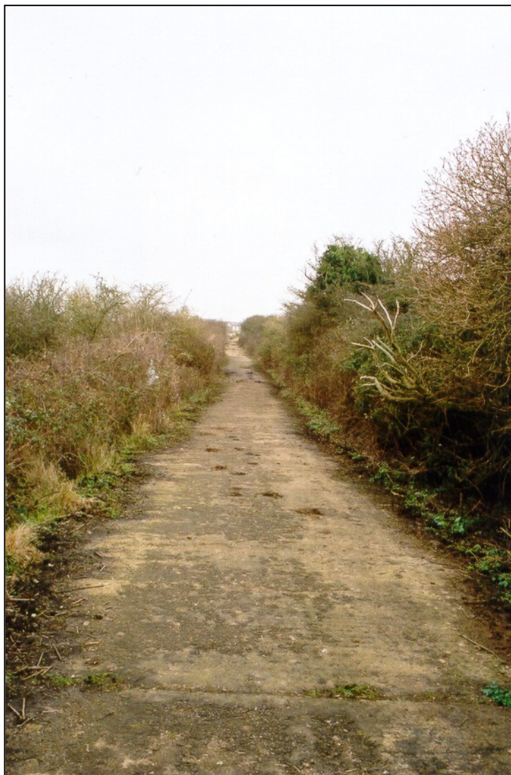
Fig. 15 - This Second World War military road,, surfaced with concrete slabs, runs between the Citadel and the Farthingloe anti-aircraft battery. Other military roads descend the hillside towards Farthingloe.
