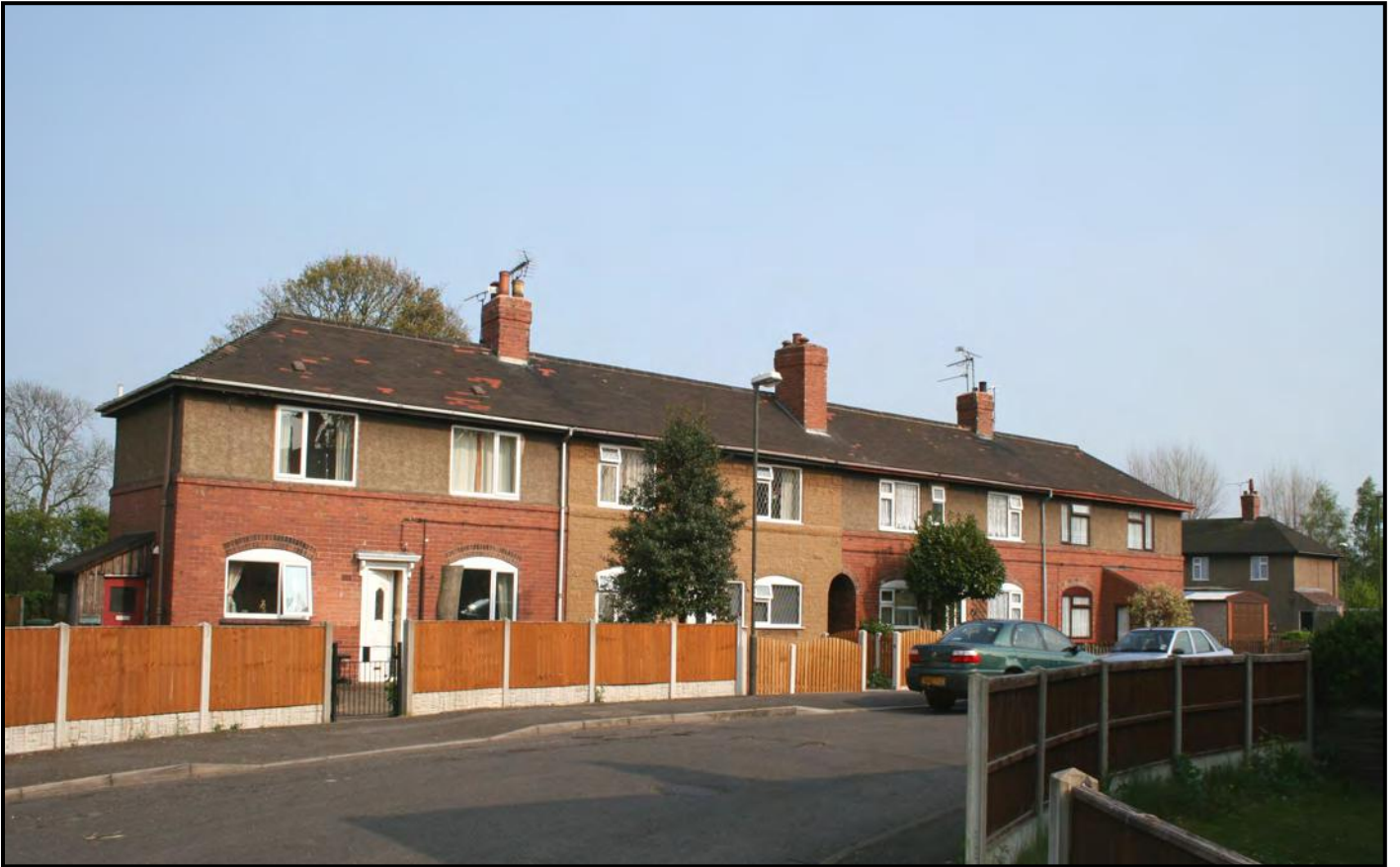
Fig. 70 A block of four houses built at The Woodlands, Whaley Thorns by the Industrial Housing Association in the early 1920s.
