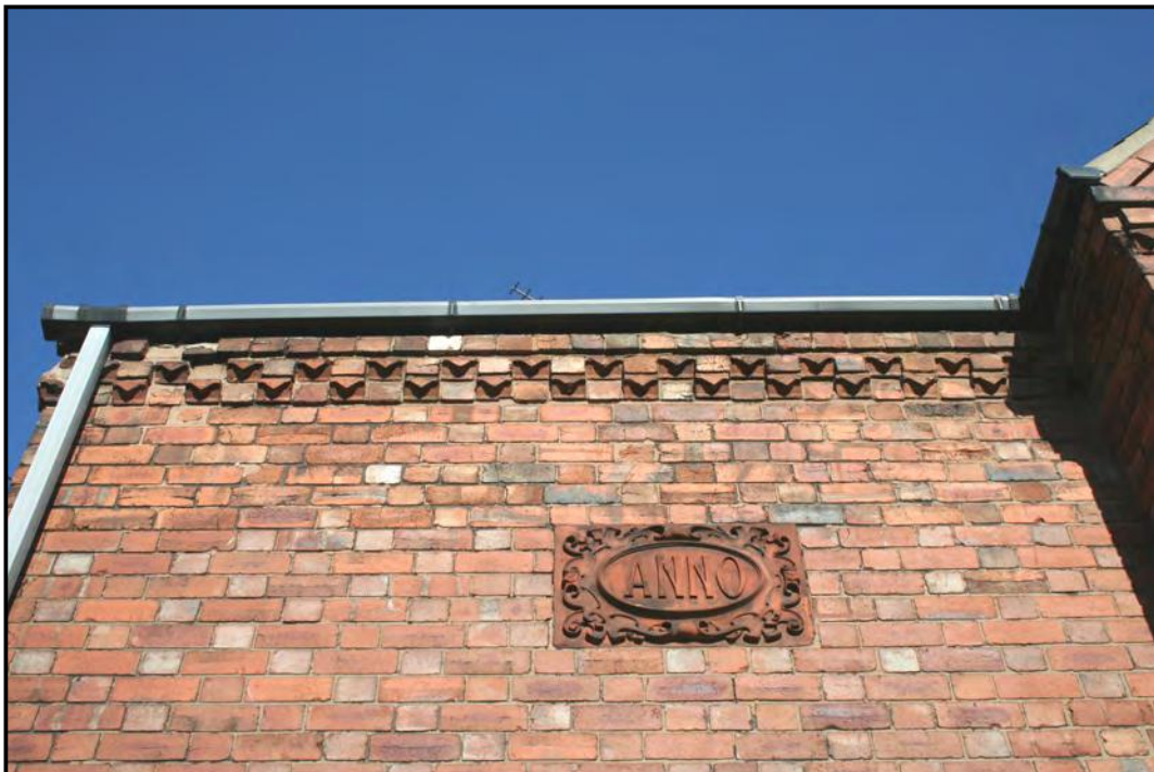
Fig. 19 Decorative brickwork and terracotta plaque on the frontage of one of The Villas at New Bolsover.
