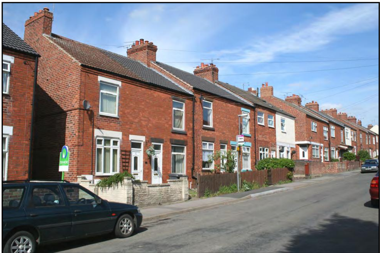
Fig. 35 Terraced houses, built mainly in blocks of 6, on the north side of Charlesworth Street, Carr Vale. These may be the houses built by Hill and Dakin in 1902.
