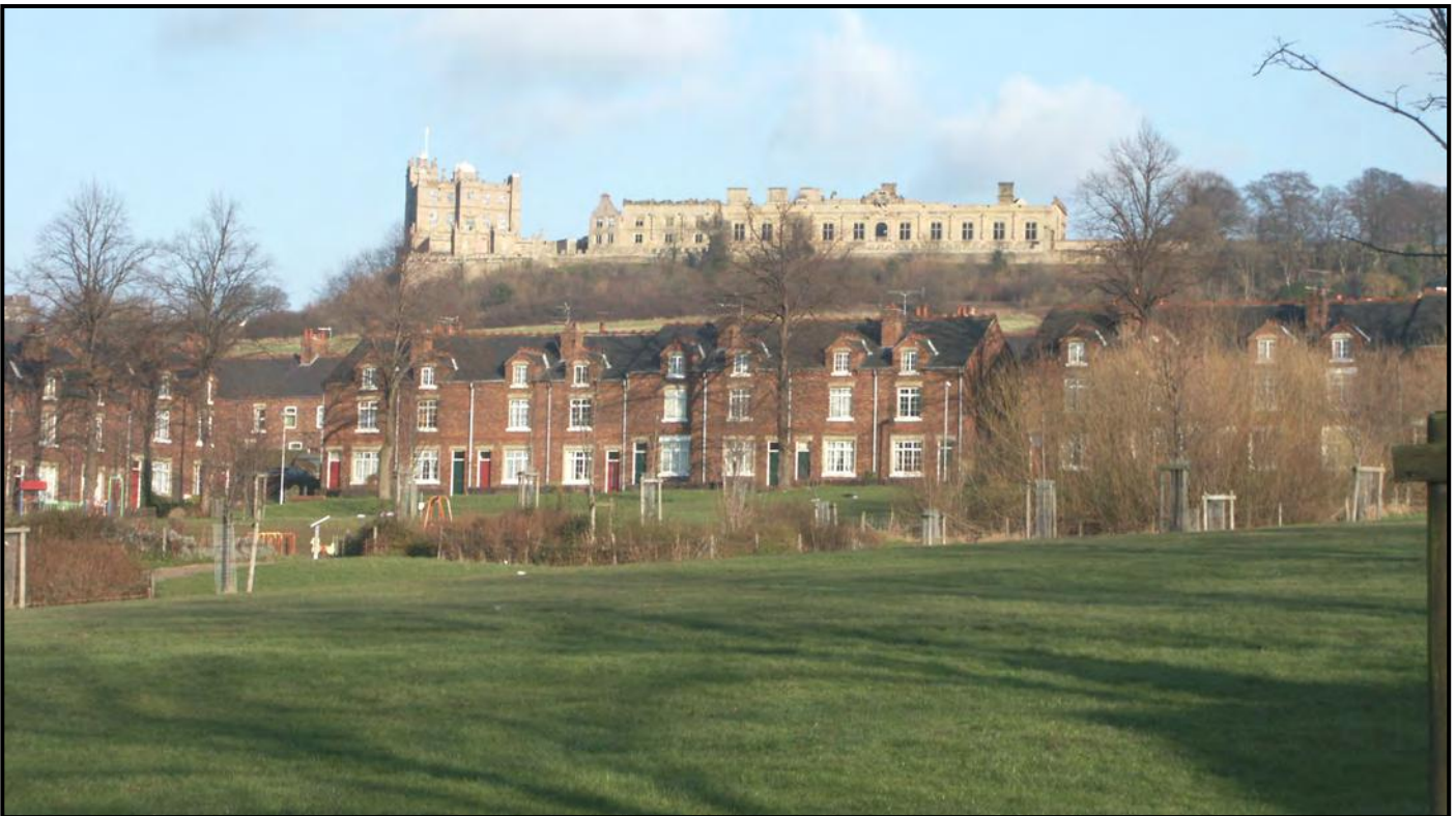
Fig. 7 Houses at New Bolsover that overlook the central green and have Bolsover Castle as a backdrop.
