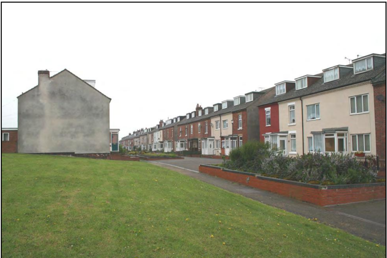
Fig. 52 View along Bentinck Road showing the now pedestrianised central road, the attic dormer windows, added porches and, to far left, part of a single storey extension to the rear of the houses.
