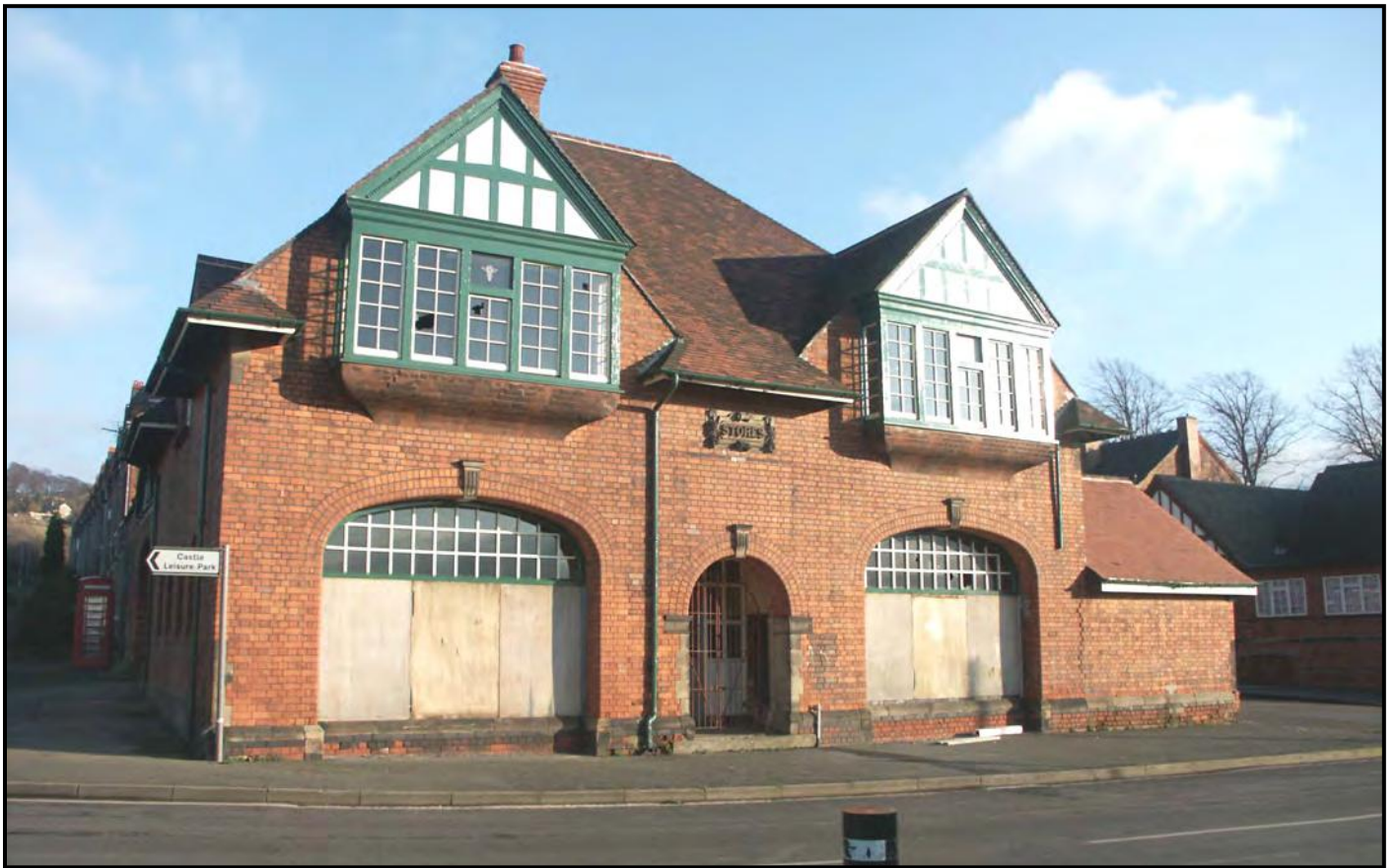
Fig. 21 The former Co-operative stores at New Bolsover, currently being refurbished for domestic use.
