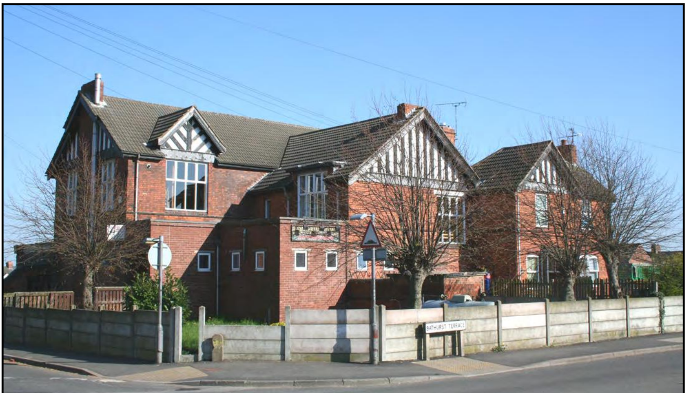
Fig. 67 The large but architecturally uninspiring Miner's Institute building on Main Street, Whaley Thorns, situated close to the centre to the older part of the village.
