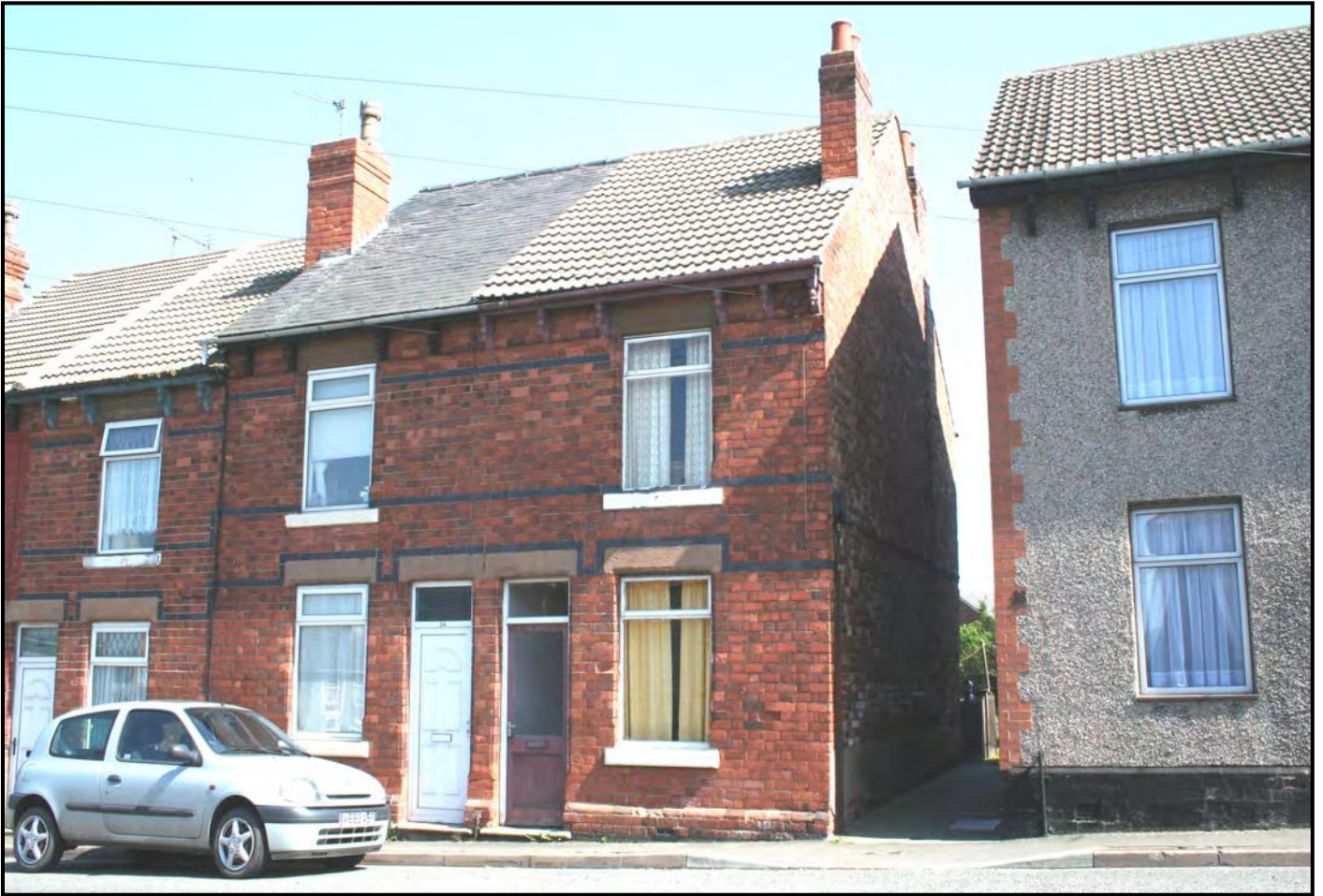
Fig. 49 Houses built on the south side of Chesterfield Road, Shuttlewood after 1900.
