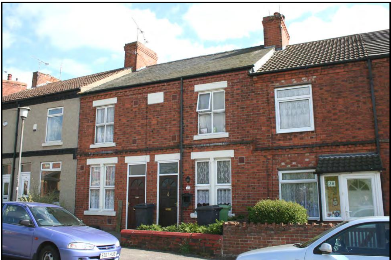
Fig. 33 A pair of largely still intact original frontages (centre) of Allerton Cottages, North View Street, some of the first houses built at Carr Vale Street.
