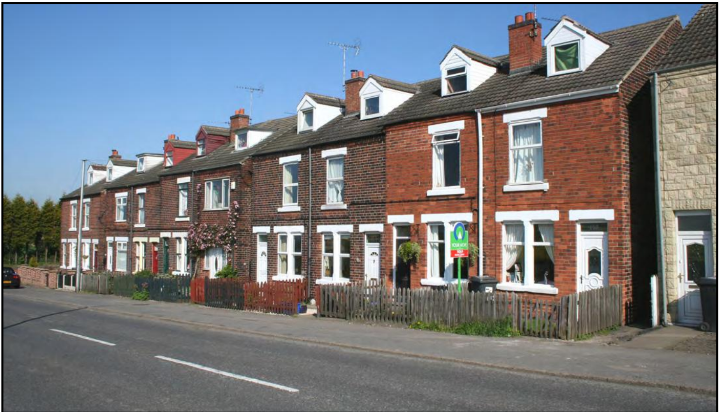
Fig. 48 Part of Springfield Terrace on Clowne Road, Stanfree. Ten good-quality and largely unaltered terraced houses with attic dormer windows, central window columns similar to ones used in Carr Vale, and small front gardens. The pair at the south end are built with a different coloured brick.
