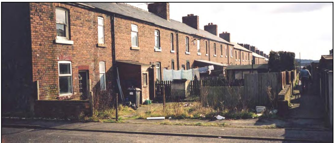
Fig. 62 View showing part of the cramped yard space between Bathurst Terrace and Scarcliffe Terrace, Whaley Thorns, now demolished. The houses' internal interlocking plan is indicated by the pattern of windows of differing width. Courtesy of Whaley Thorns Heritage Centre.
