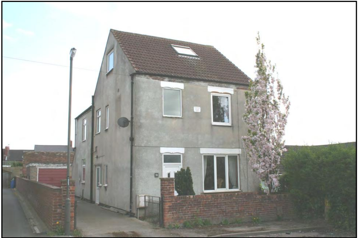
Fig. 40 A detached house built at the end of Railway Side Street, Carr Vale, by Mr Lyme, a colliery deputy at Bolsover Colliery in 1904.
