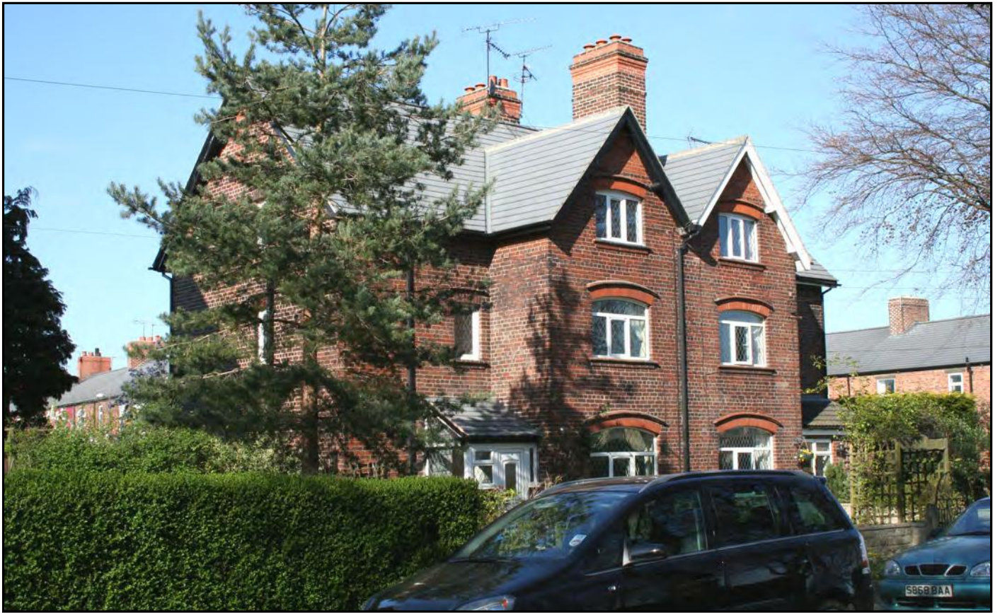
Fig. 68 One of the two relatively large semi-detached villas built for colliery officials on West Street, Whaley Thorns.
