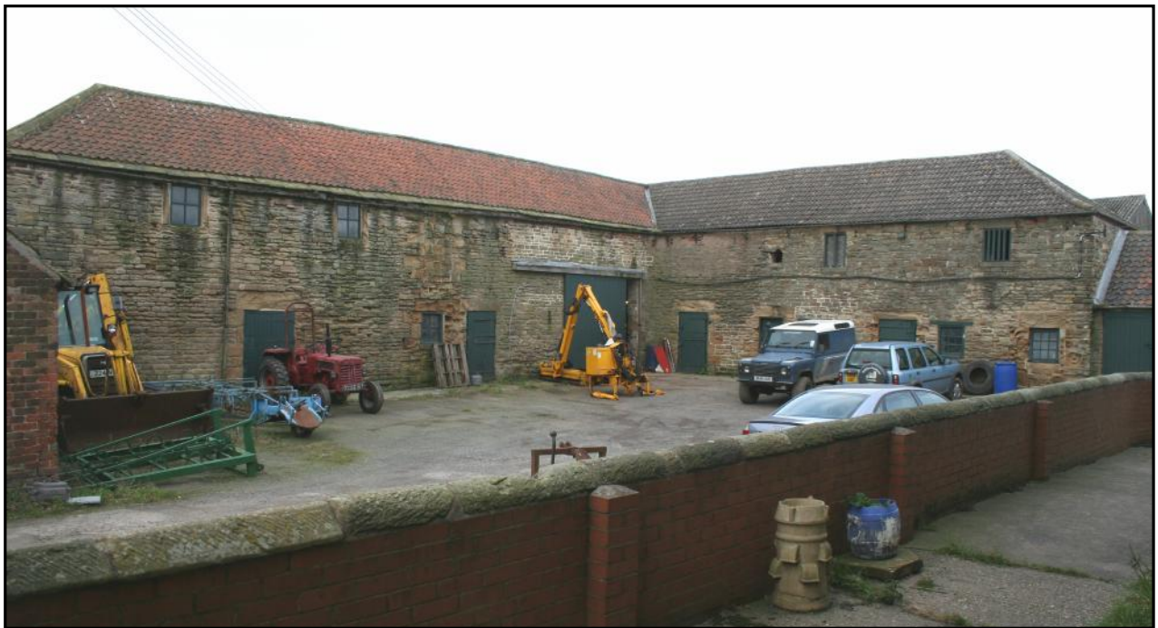
Plate 10: The continuous west and north ranges at High House Farm, probably of 18th century origin, but with much evidence of infilled doorways, differing window styles, stonework patching and replacement, and re-roofing.
