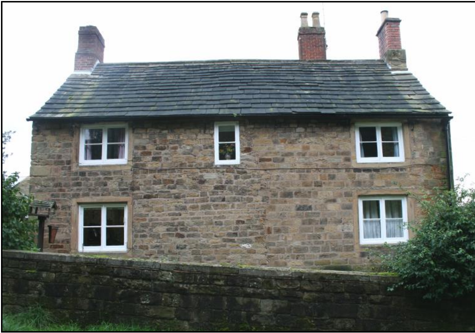
Plate 13: Street frontage of the original 18th century part of the farmhouse at Stainsby Farm. The off-centre entrance doorway has been lost during re-facing.
