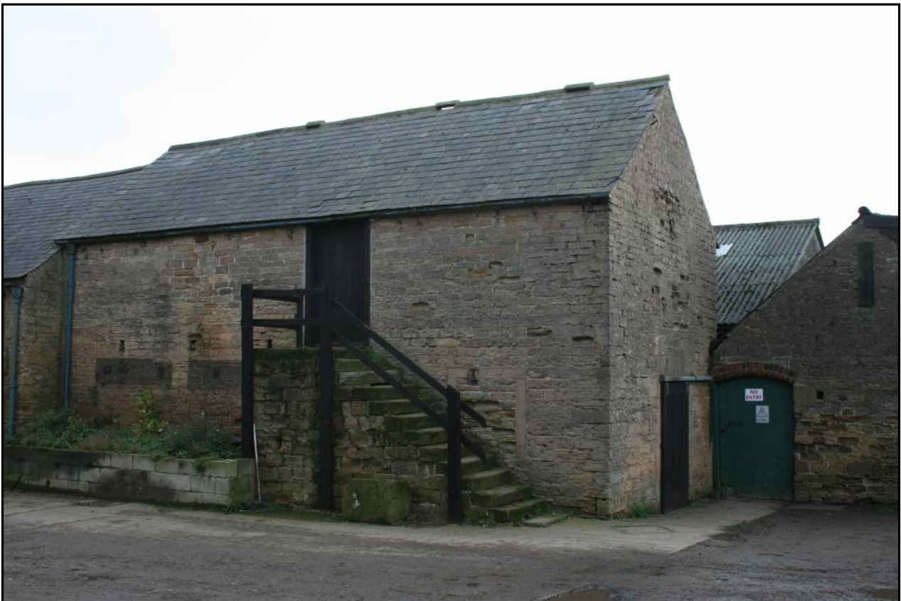
Plate 23: Building (stable with chamber over) added to the west end of the old barn at Top Farm, Rowthorne, probably in 1862.
