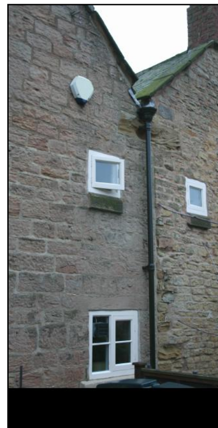
Plate 3: Distinct differences in the stonework showing on the west side of the building.
