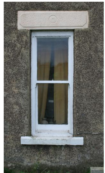
Plate 9: Victorian ornamental window lintel at the east end of the south wing.
