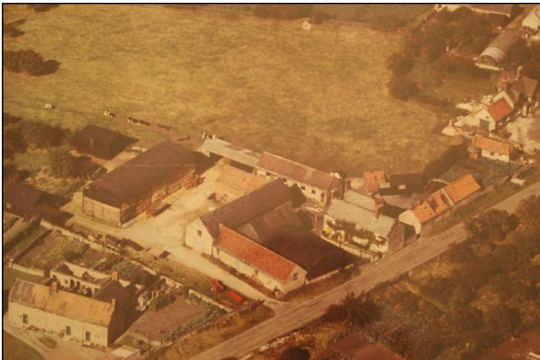
Plate 1 Aerial view of Pea Tree Farm, Rowthorne taken in the 1970s when it was still a working farm
