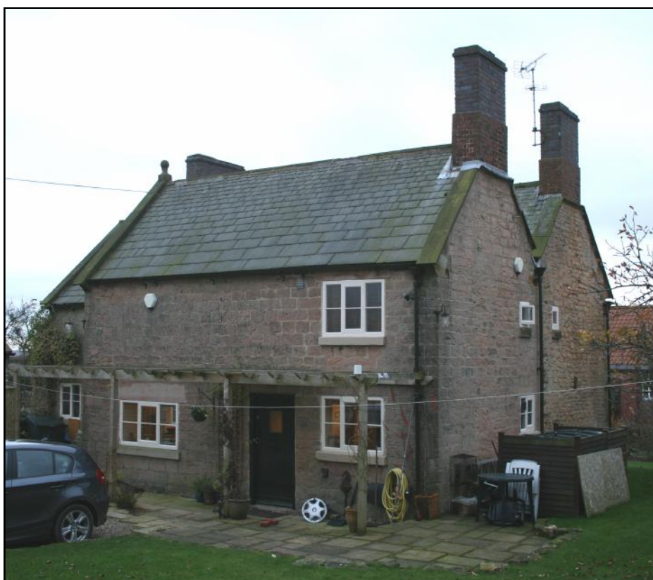
Plate 2: North, rear kitchen part of the listed former farmhouse of Pear Tree Farm, Rowthorne, showing the double gable roof-line and similar brick end stacks.
