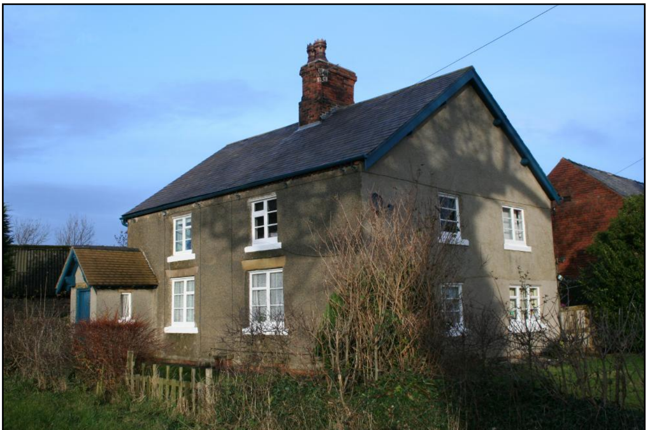
Plate 28: View of the former cottages built near existing farm buildings at Batley Barn / Farm, in 1878. To the far right there is a larger window where a side entry used to be. The building had become a single farmhouse before 1900.
