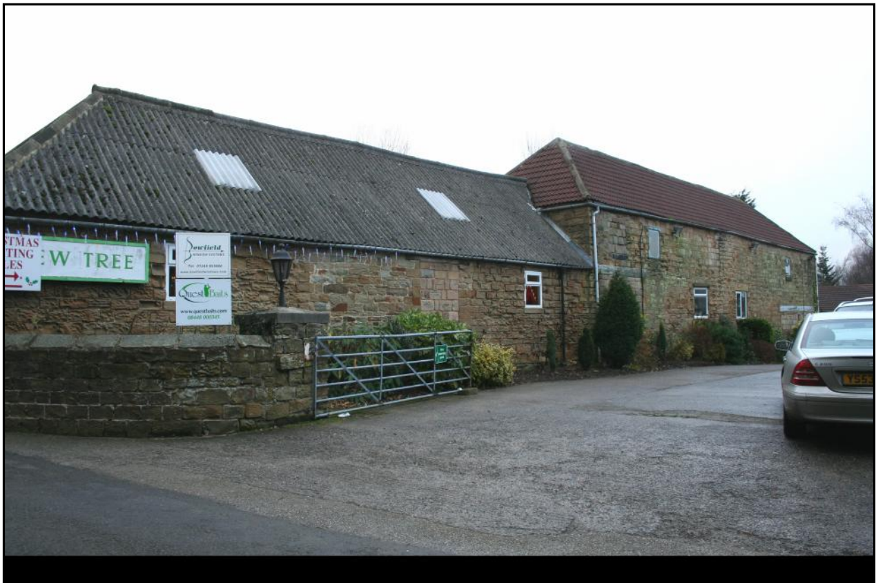
Plate 26: The east range built at Yew Tree Farm, Hardstoft, between 1870-74, with cowhouses to left and the barn to right.
