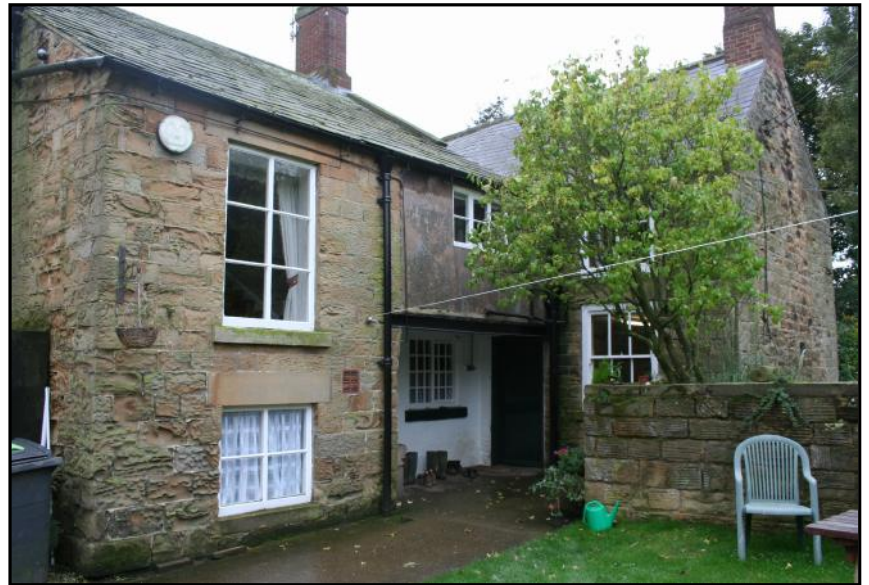
Plate 14: The back of the farmhouse, showing the older part to right and the central projecting part of the 19th century extension to the left. The middle part shows a later bedroom addition.
