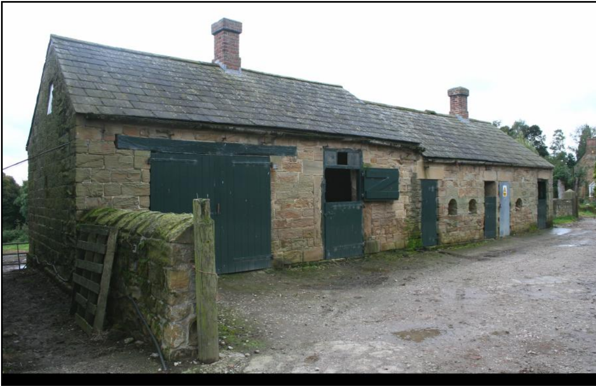
Plate 20: The mid-19th century single-storey south range (F) at Stainsby Farm, a combined gig house, stable, piggeries and wash-house at Stainsby Farm.
