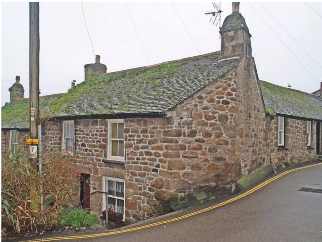
38. Context: houses west of Keigwins (17 th century dressed granite stack but rebuilt front wall)
