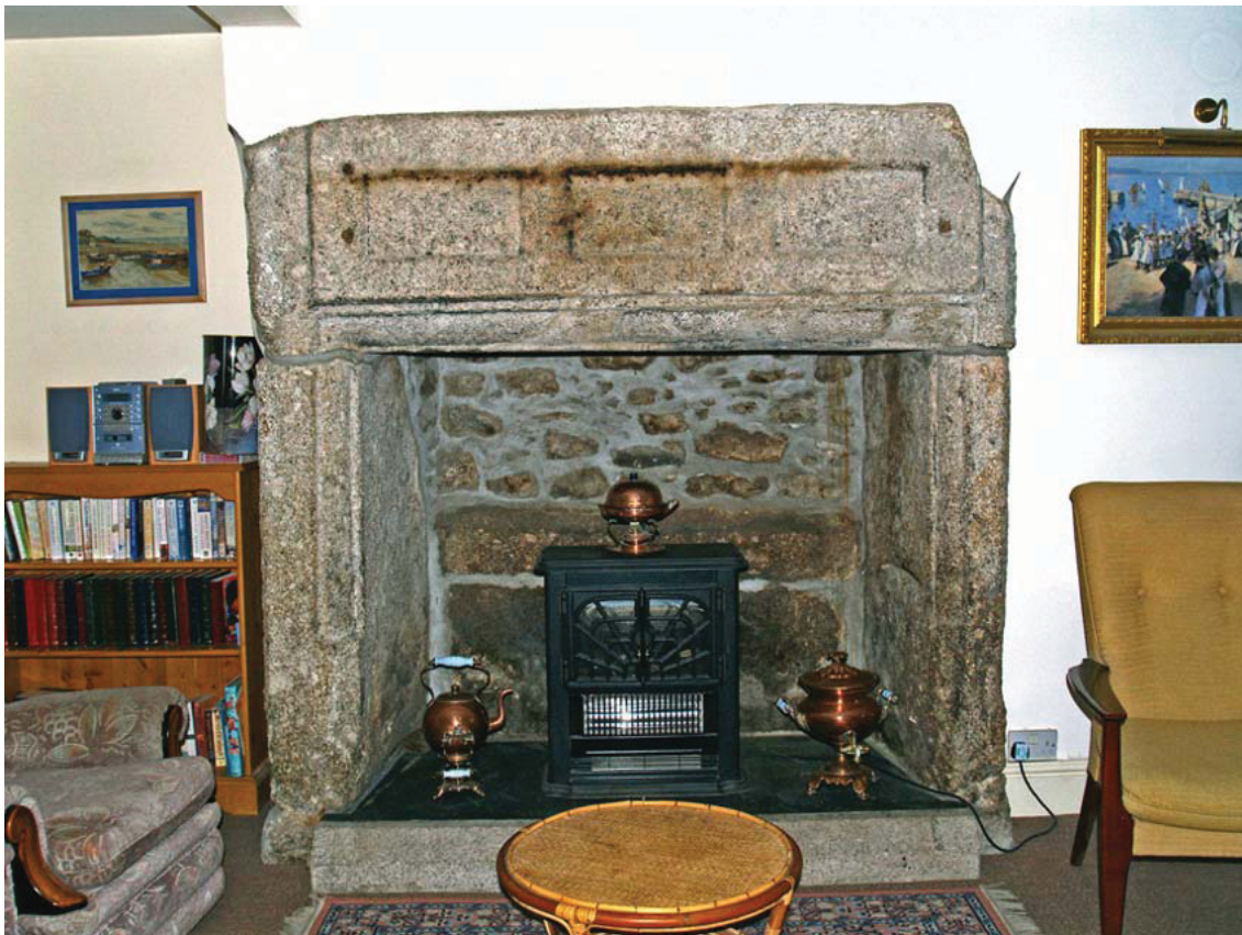
32. Old Standard: moulded granite hall fireplace with panelled lintel, at west gable end
