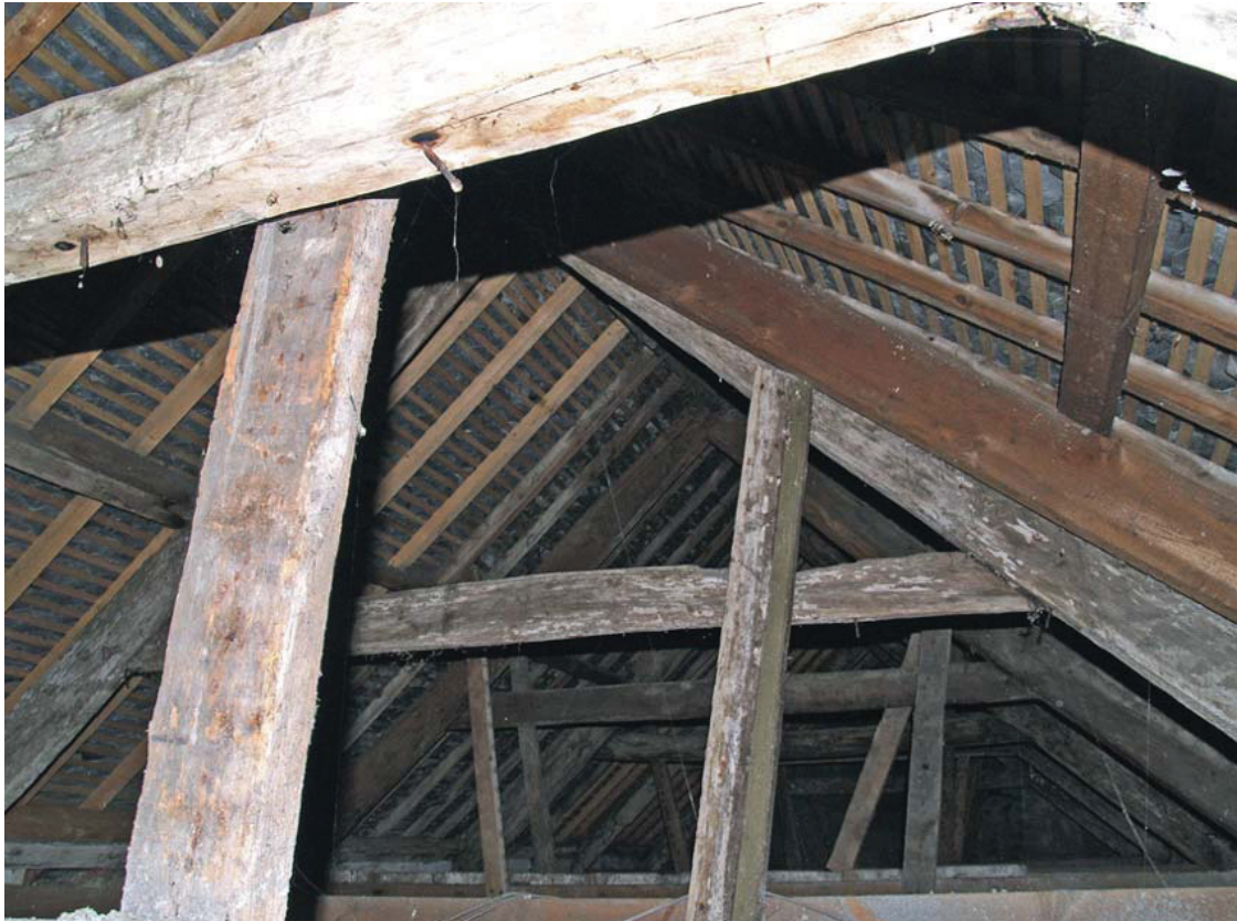
31. Old Standard: original 7-bay roof structure over front range (note lime-wash)
