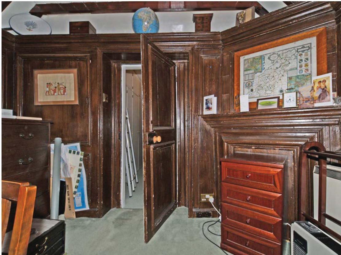
25. Keigwin: bolection-moulded panelled room over porch
