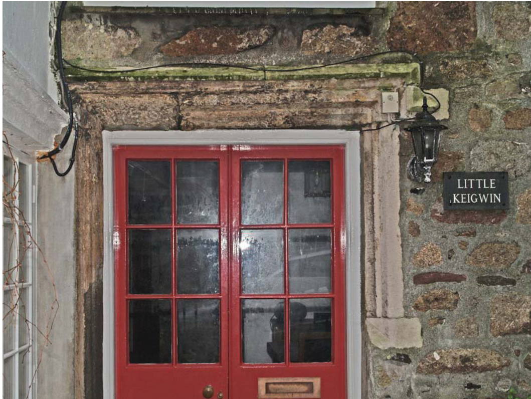
5. Little Keigwin: lintel and jamb remains of freestone 3-light mullioned window
