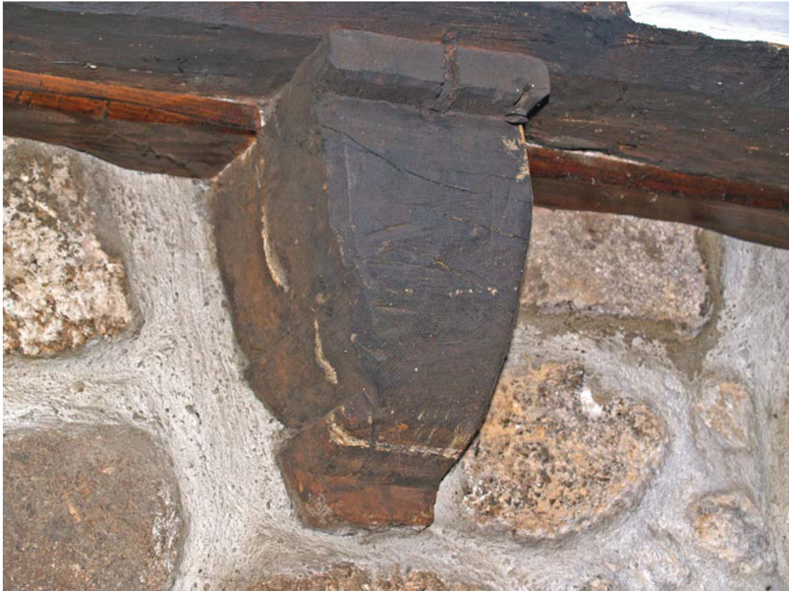
27. Little Keigwin: principal ground-floor room, moulded corbel under 1 st -floor fireplace
