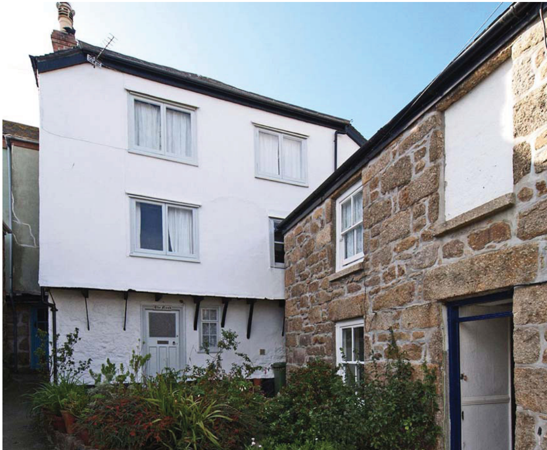
41. Context: jettied rear at south end of Chapel Street and Wesley House
