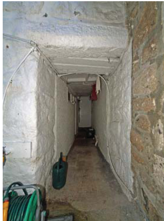
10. Keigwin: doorway from rear court to rear
