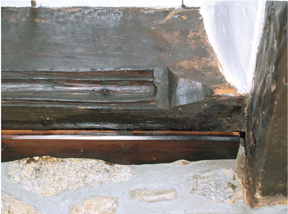
15. Keigwin: hall ceiling detail with moulded joist and stop
