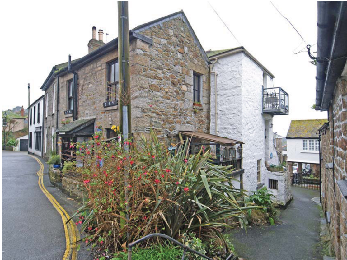
37. Context: Chapel Street and Keigwin Place: buildings north-east of Keigwins
