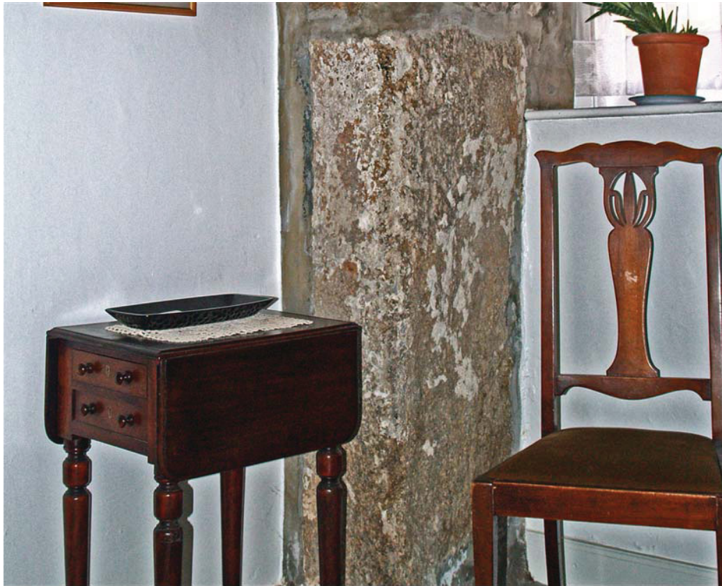
11. Keigwin: chamfered jamb of hall fireplace
