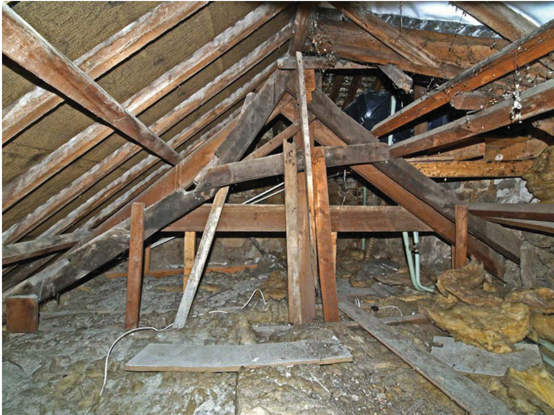
19. Keigwin: roof over rear range; original smoke-blackened truss at west end
