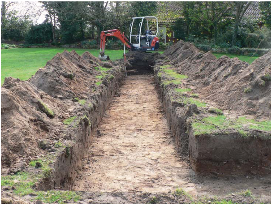
North west/south east trench from north
