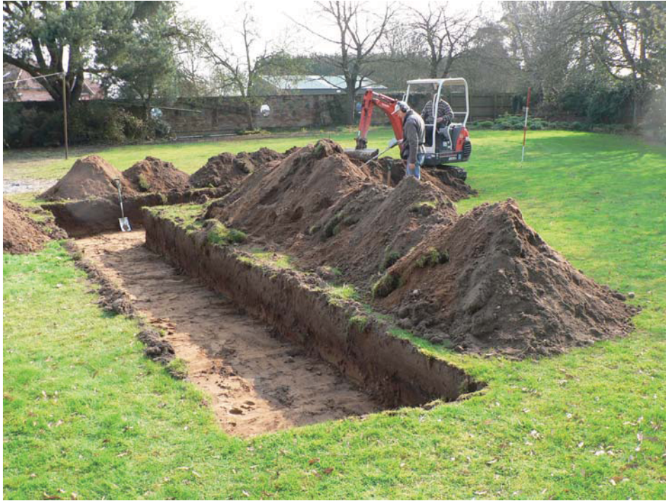
South west/north east trench from west
