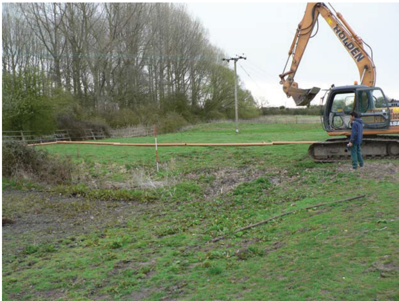
Before works start from north west
