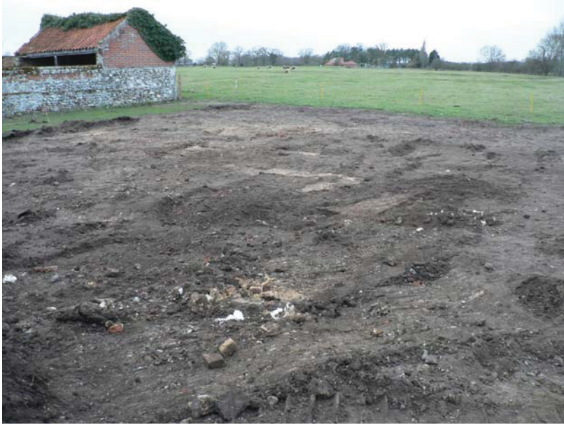
View from SE, pad 0011 in foreground, foundations 0007 & 0009 beyond
