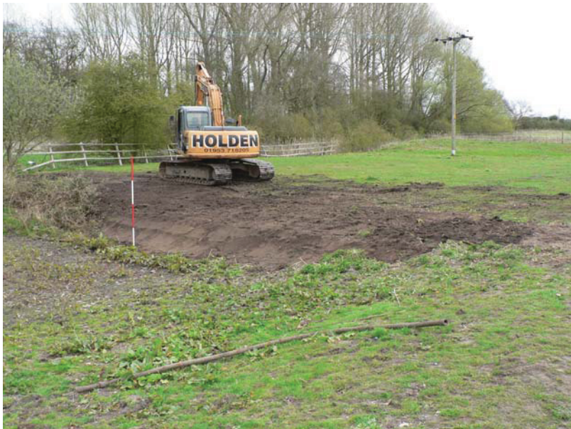
After concealment of pipe from north west
