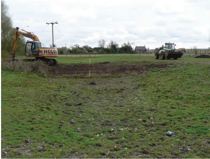
After concealment of pipe from north
