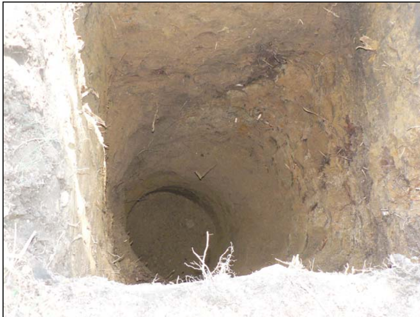
Post pit excavated to 3m in ?quarry pit fill
