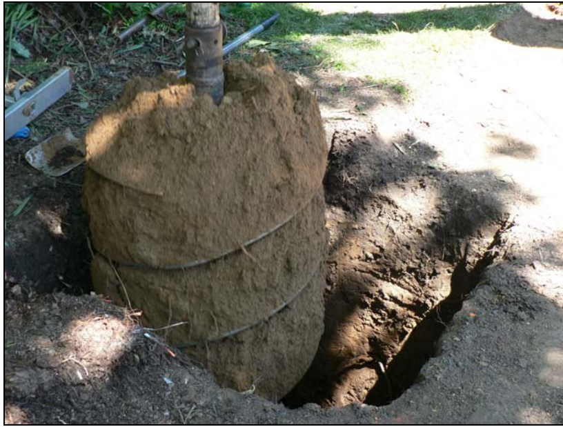
Coring head in operation- post pit in part of footprint over large ?quarry pit
