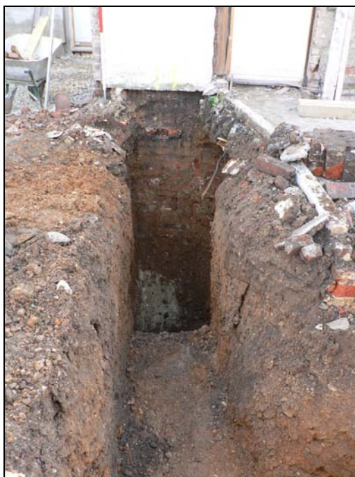
Northern trench from west showing existing cellar foundation & natural white sand below (A on Fig.)natural gravel deposit
