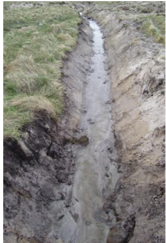
Figure 4b – old drain re-excavated
