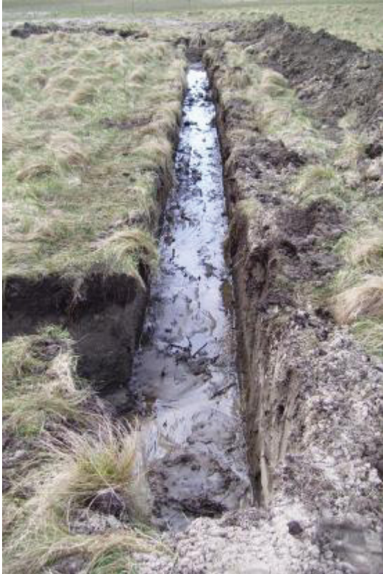
Figure 4a – new drainage for septic tank
