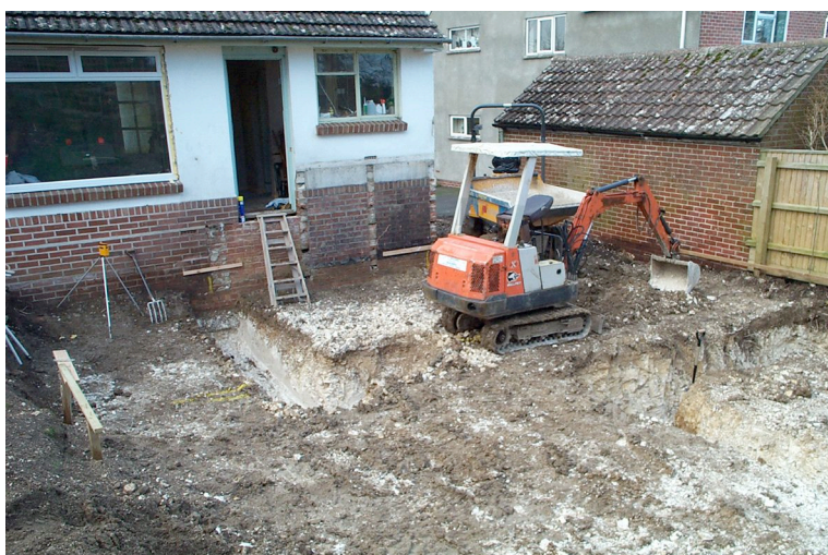
Plate 3: Footings trench against rear of bungalow
