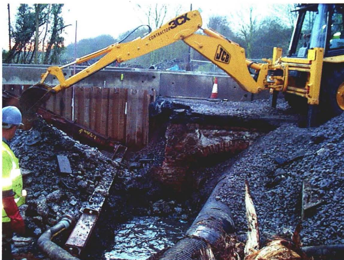
Fig. 2: Excavations in progress showing brick arch of existing bridge
