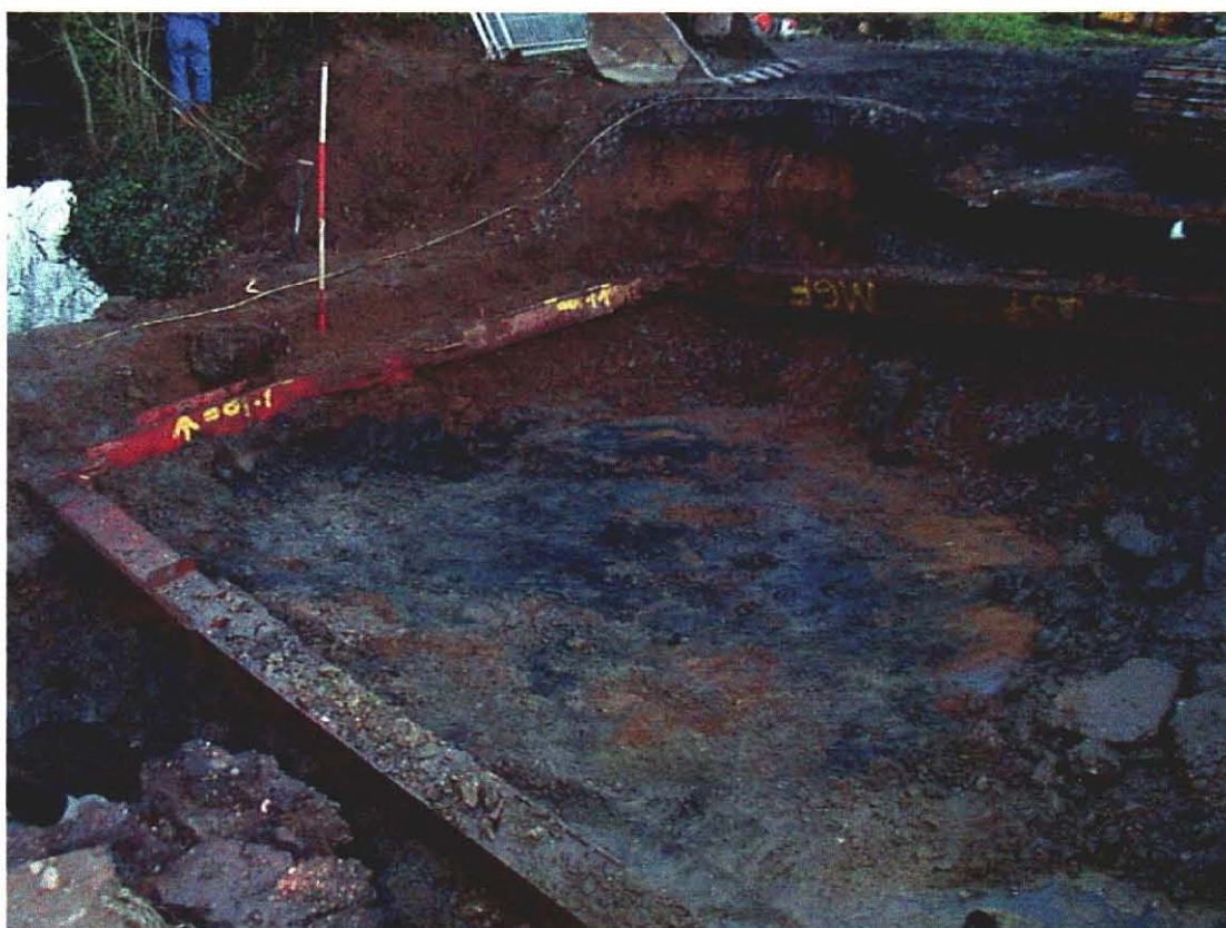
Fig. 3: Old stream channel deposits below road surfaces
