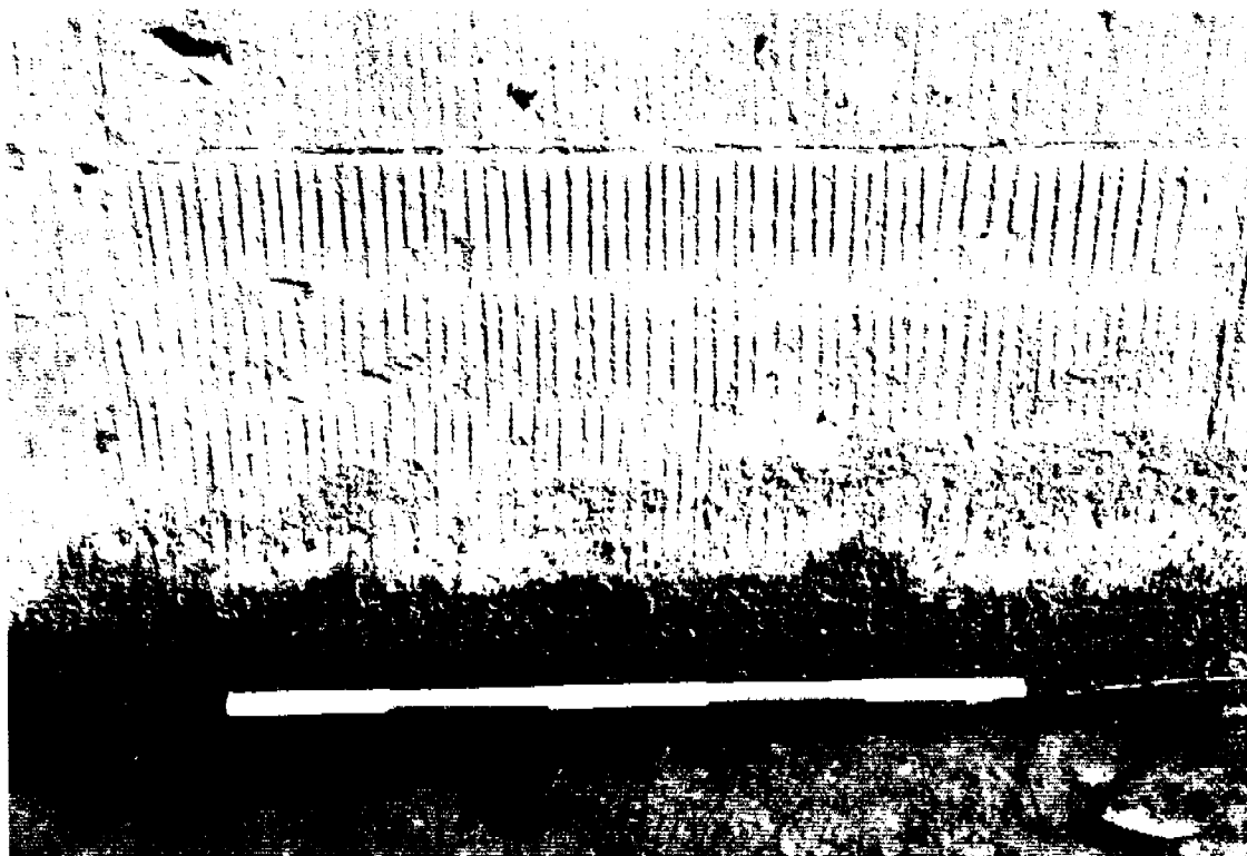
Fig 20: Phase 4 'corduroy' tooling
