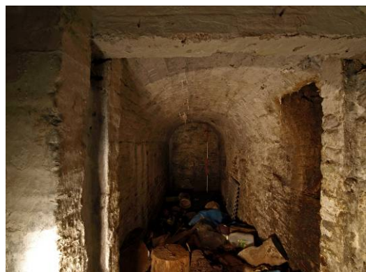
Plate 82 Coal Cellar (Room 38) looking north
