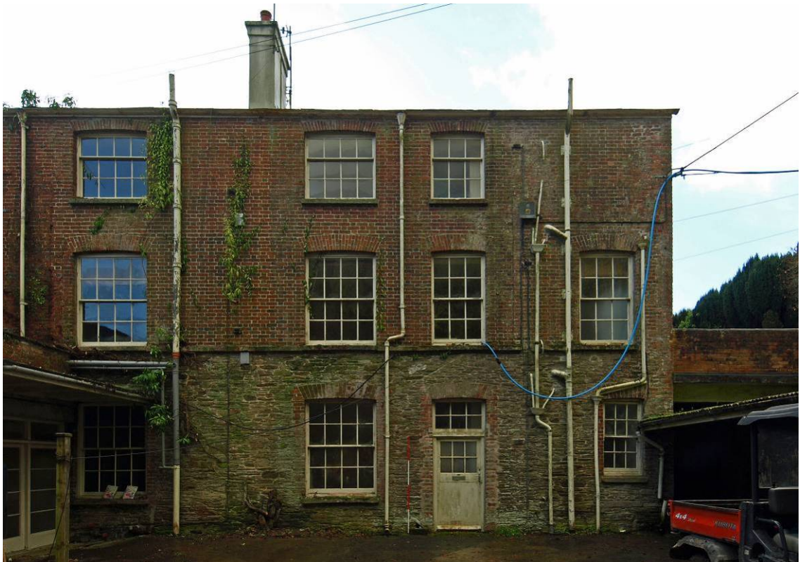
Plate 23 Rear Wing, north elevation
