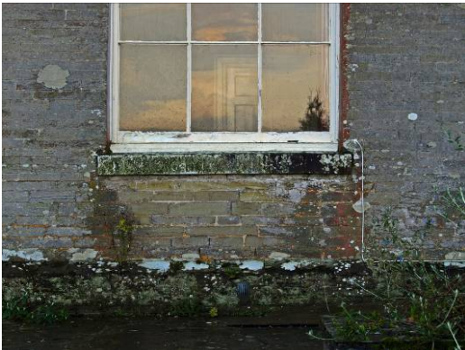
Plate 8 Window sill right of doorway
