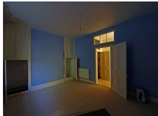
Plate 63 Room 19, looking southeast showing panelled cupboards flanking blocked fireplace and later 19 th century four-panel door.
