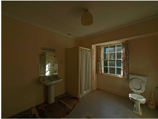
Plate 47 Bathroom (Room 46) in probable former stair wing.
