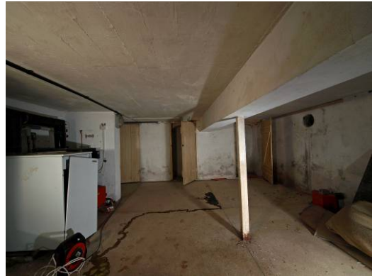
Plate 56 East Range, original basement (Room 31) looking north.
