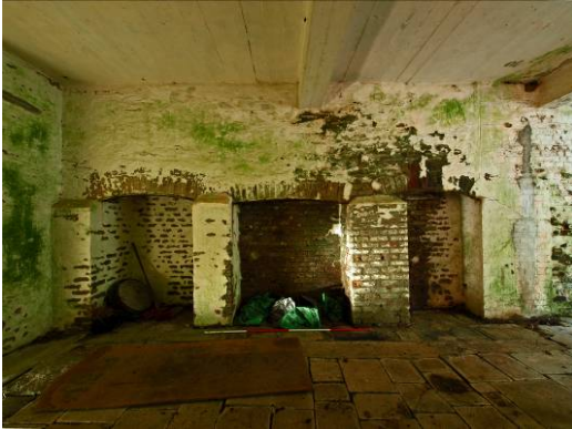
Plate 59 Former Kitchen (Room 15) at west end of Rear Wing, truncated probably 1925, the fireplaces surviving under 1950s flat roof
