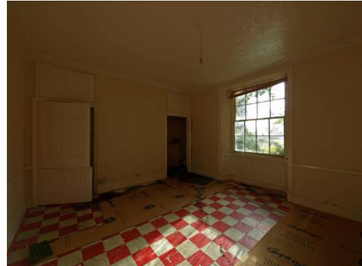
Plate 62 Rear Wing, ground floor, Room 21, looking southeast showing panelled cupboards flanking blocked fireplace and c1831 sash window
