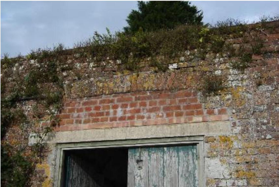
Plate 130 Additional lintel with arch head infill repairing an opening in the south elevation of the Workshop and Stores building.
