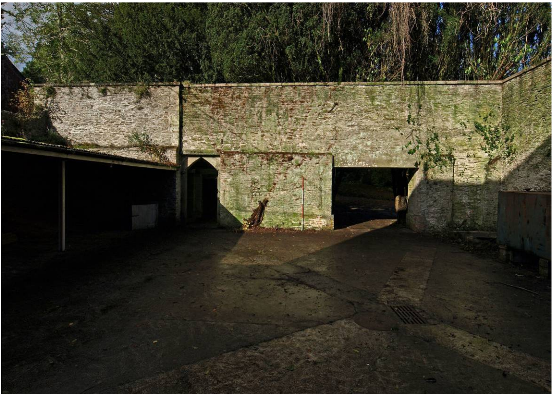
Plate 26 Courtyard, north wall (remains of north range)
