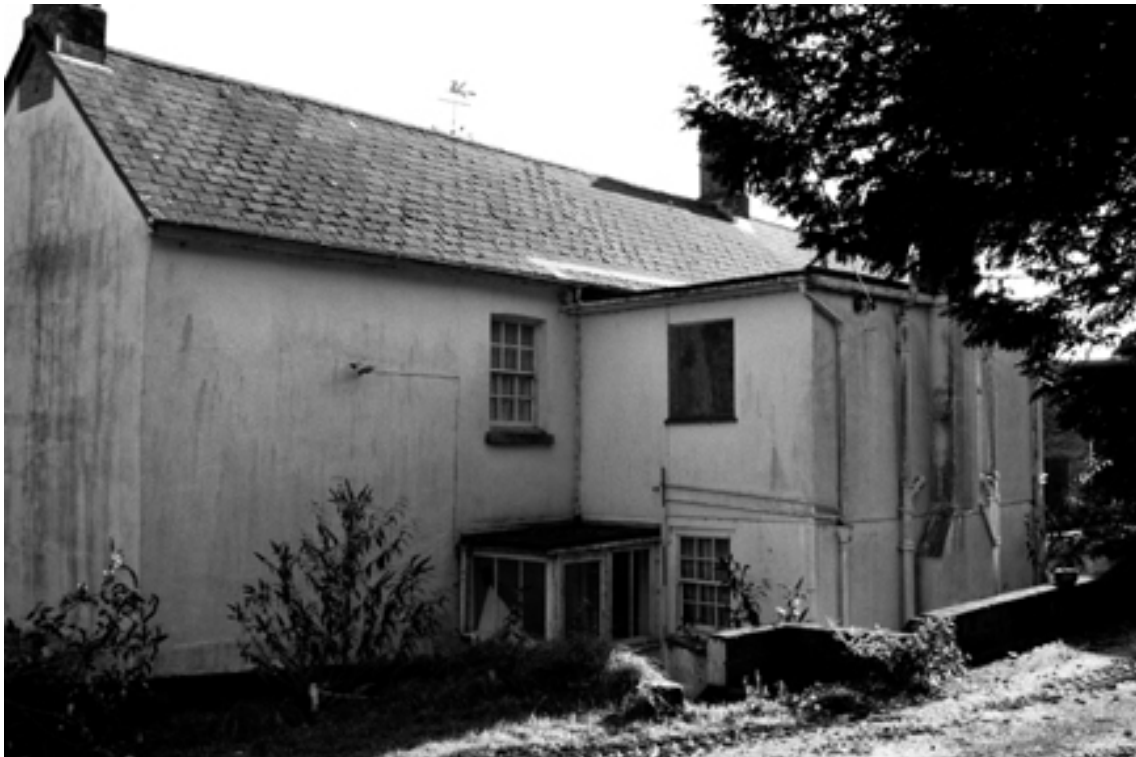
Plate 121 The Bothy Building looking southeast showing western extension.
