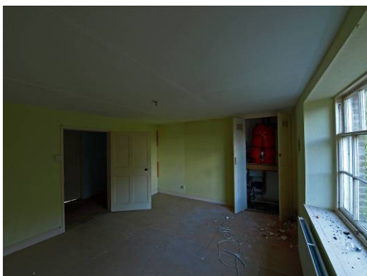
Plate 73 Rear Wing, second floor Room 64 looking west, showing c.1831 panelled doors and sash window.
