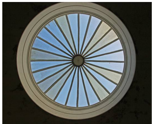
Plate 52 Former principal stair hall (Room 50), roof oculus detail.
