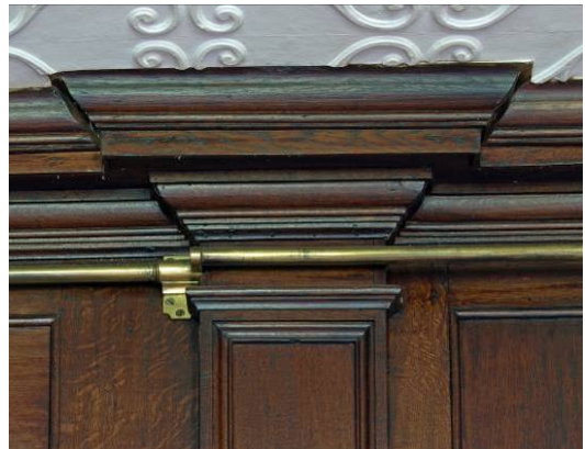
Plate 87 East Range, South Reception Room 3.
