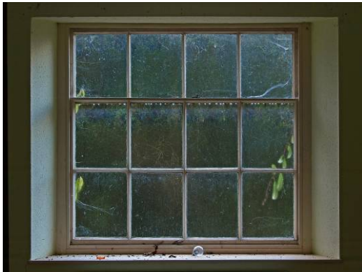
Plate 72 Rear Wing, second floor Room 63 north window c.1831 four over eight-pane sash.
