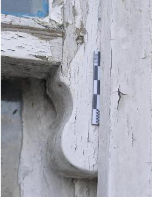
Plate 122 Detail of a horned sash window type 1
