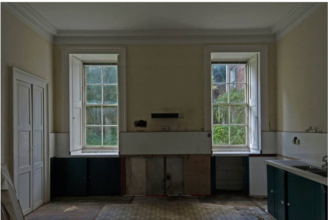
Plate 32 East Range, Rear South Room 4, west windows probably replaced in 1831
