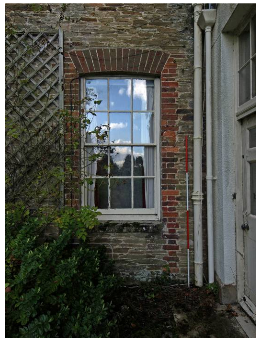
Plate 21 Rear Wing, south wall: former doorway
