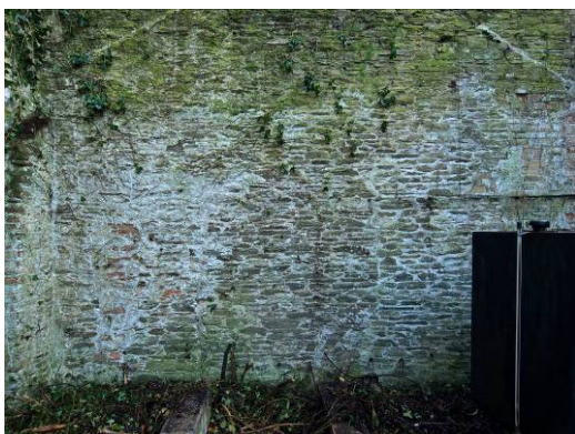
Plate 24 Courtyard east side, evidence of former openings and former roof line
