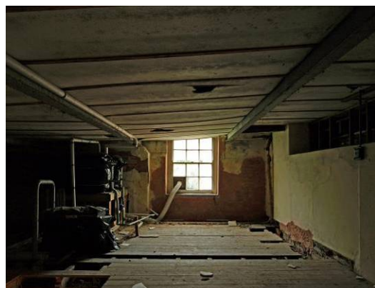
Plate 58 Attic (Room 70) above southwest corner of East Range, looking west.
