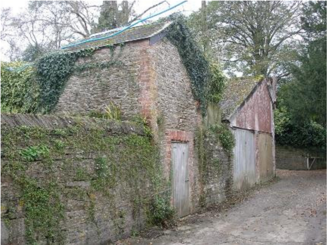
Plate 108 Woodside outhouse looking northwest
