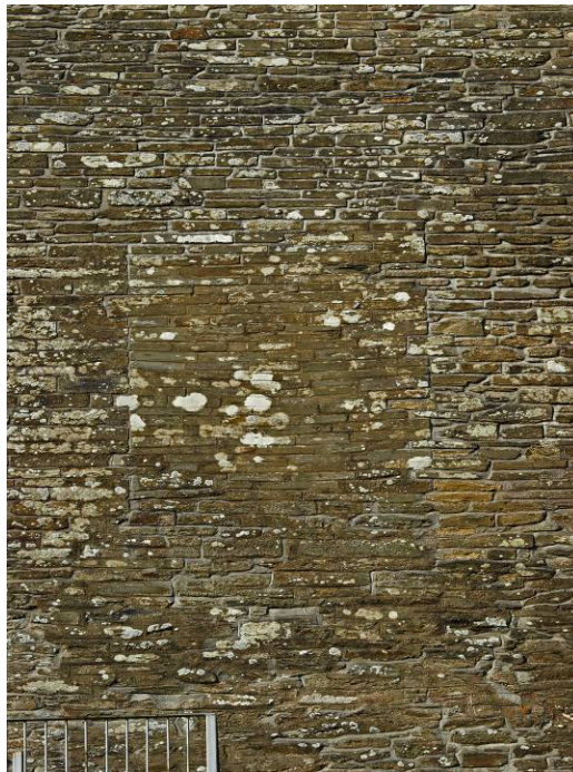
Plate 12 South end of East Range detail showing blocked first-floor window.
