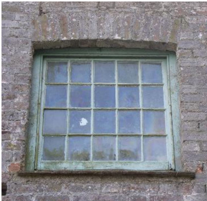
Plate 138 Detail of tilting window, north elevation, Motor House.
