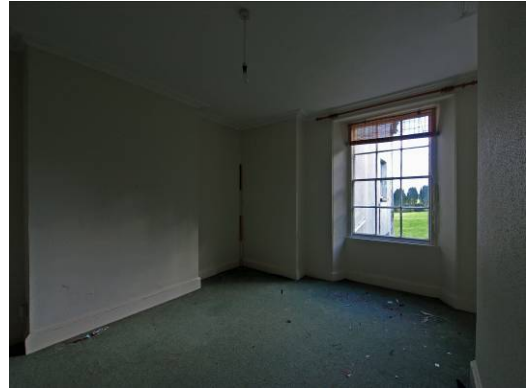
Plate 68 Rear Wing, first floor, Room 56 looking southeast showing blocked fireplace, c.1831 sash window, ceiling cornice, and pre-1831, thicker walling left of window
