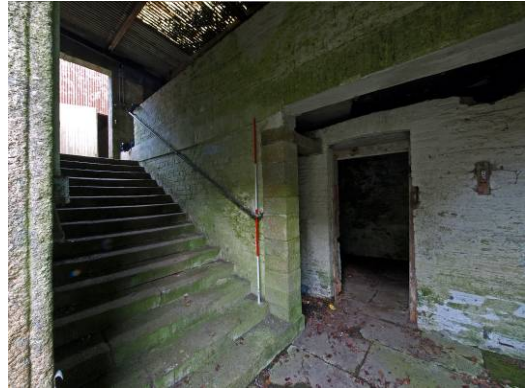
Plate 4 Northwest Wing: granite staircase in Room 33, looking northwest, with cellar doorway, right.
