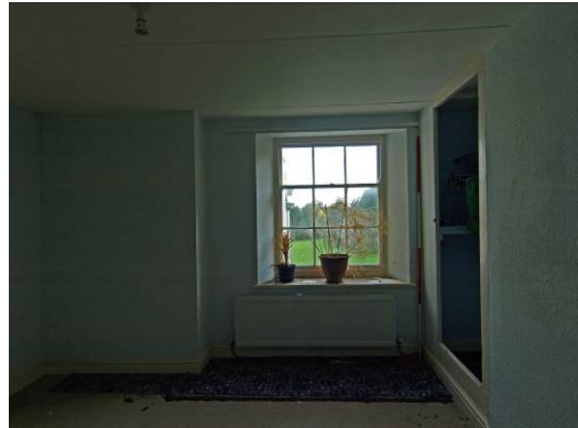
Plate 74 Rear Wing, second floor Room 65 looking south showing c.1831 sash window, and earlier thicker, walling to left.
