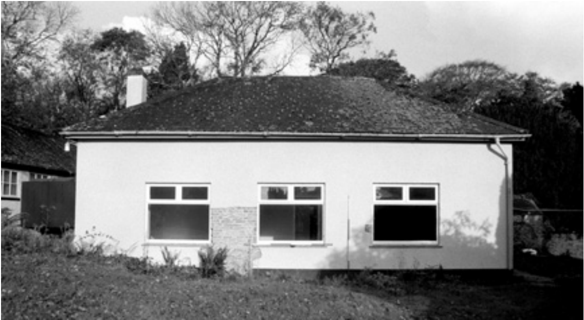
Plate 110 Woodside south elevation
