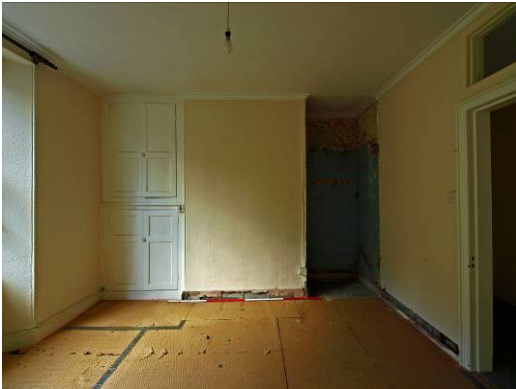
Plate 65 Rear Wing, first floor, bedroom (Room 55) looking east showing cupboards flanking blocked fireplace
