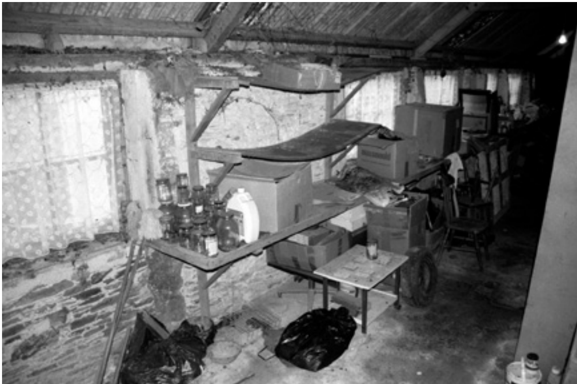
Plate 101 The interior of the workshop looking southeast
