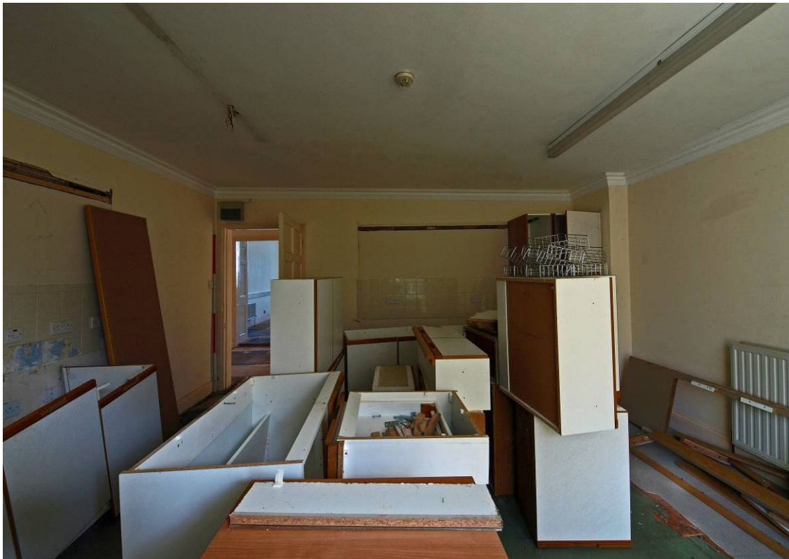
Plate 46 East Range, rear bed chamber (Room 45), added when the East Range was extended c1790
