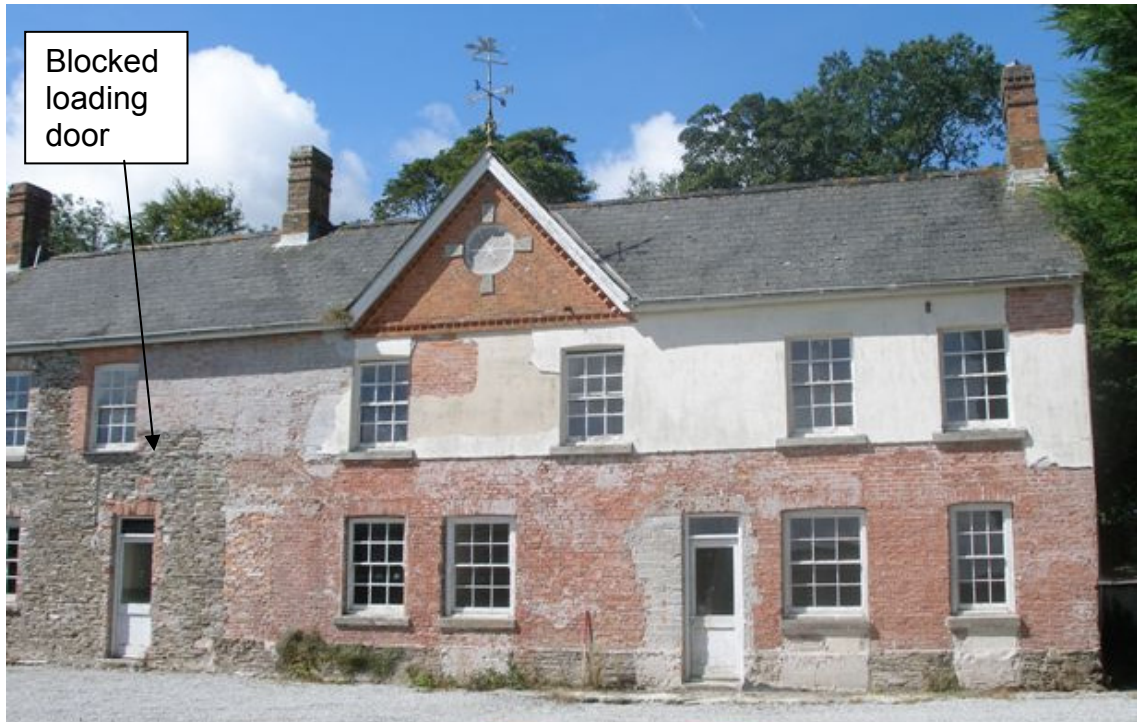
Plate 120 East elevation of the Bothy Building with Flemish bond brickwork, common from the 18 th century onwards.
