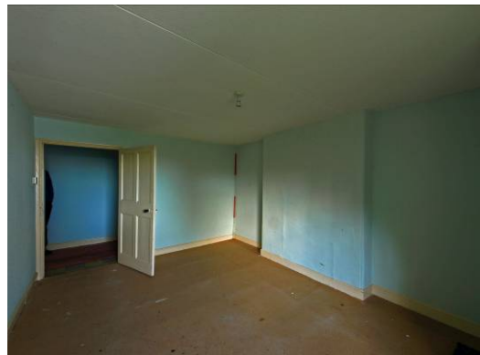
Plate 75 Rear Wing, second floor Room 65 looking northeast, showing panelled door and blocked fireplace.
