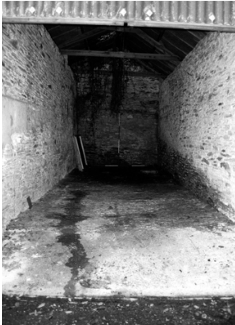
Plate 106 The interior of the northern bay of the garage, looking west
