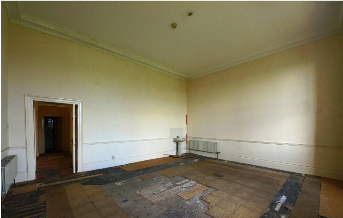
Plate 42 East Range, north bed chamber (Room 40) looking northwest.
