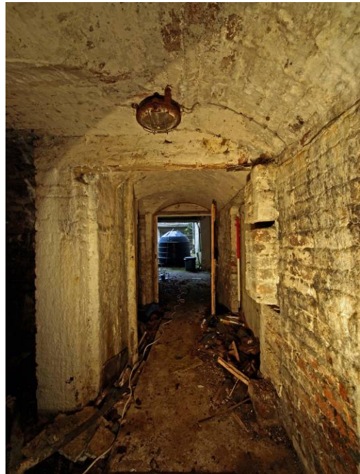
Plate 81 Coal Cellar passage (Room 25) looking east.
