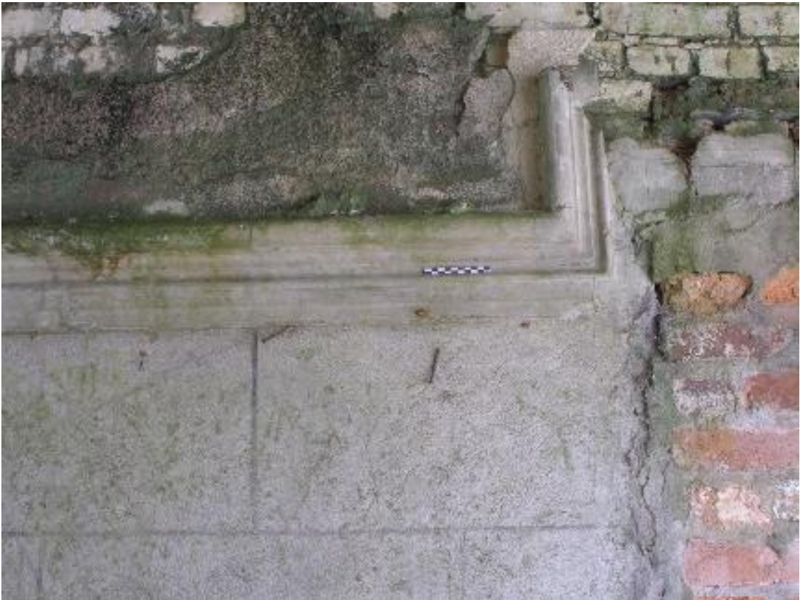
Plate 132 Detail of moulding in the Stores building
