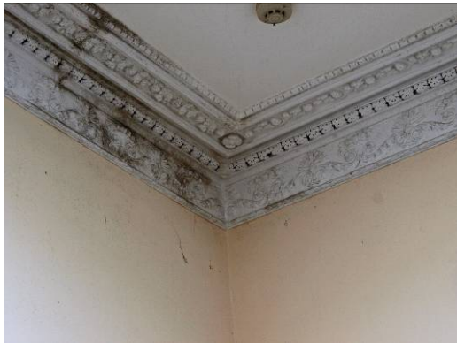
Plate 96 Central Hall (Room 50), c.1831 cornice to former stair hall.
