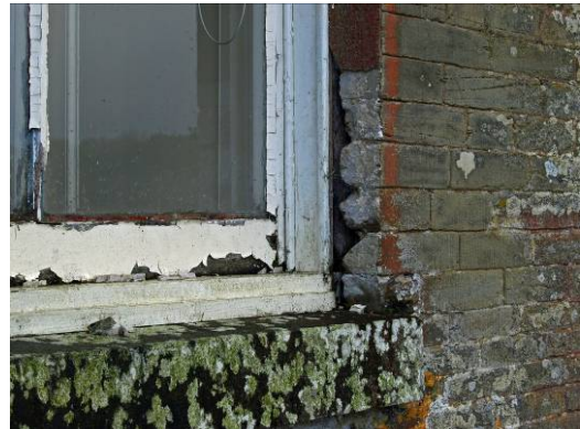
Plate 10 East Front, window jamb far right showing jamb stonework cut back
