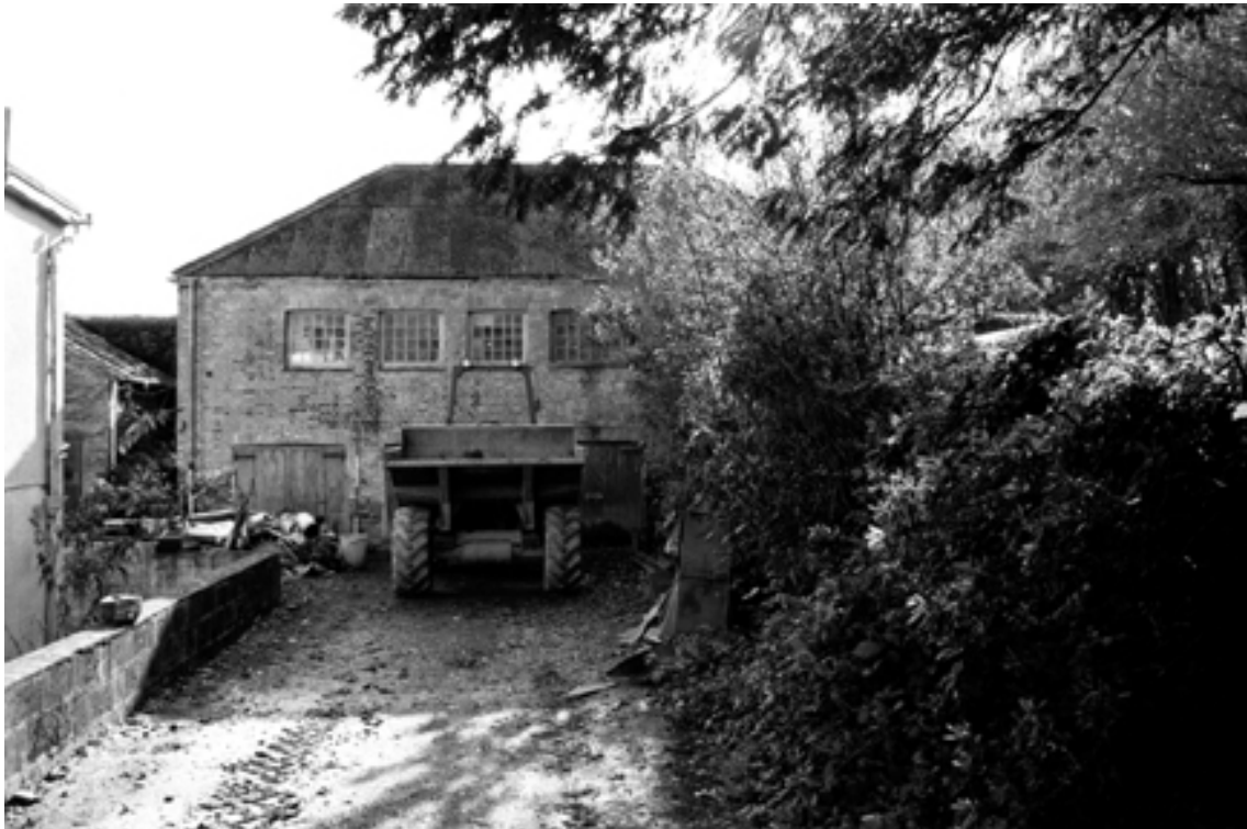
Plate 136 North elevation of the Motor House
