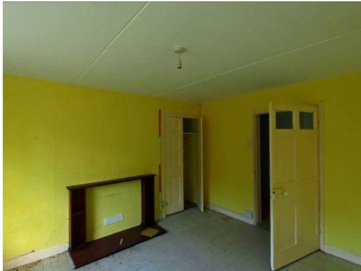
Plate 71 Rear Wing, second floor, Room 62, looking southeast showing fireplace, and c.1831 panelled cupboard and door.
