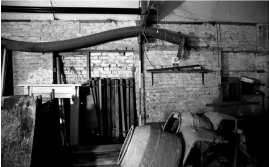
Plate 139 The woodworking ventilation pipe is visible in the first-floor of the Motor House with blocked window openings, looking south.
