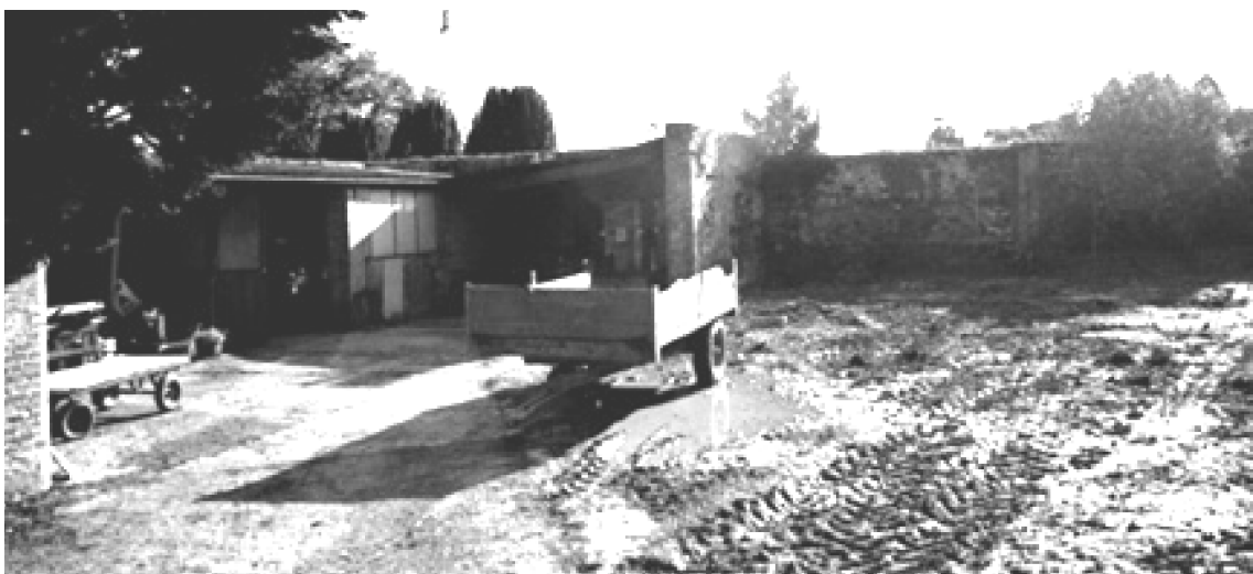
Plate 126 Workshop and Stores, looking southeast
