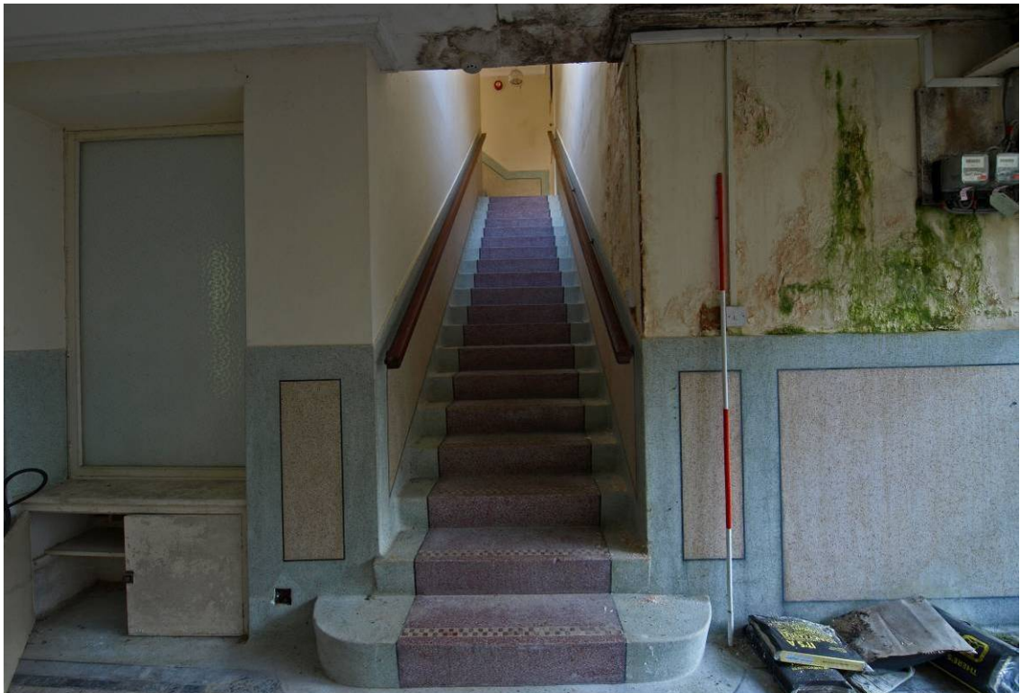
Plate 36 East Range, 1950s rear entrance hall (Room 9) with terrazzo detail.
