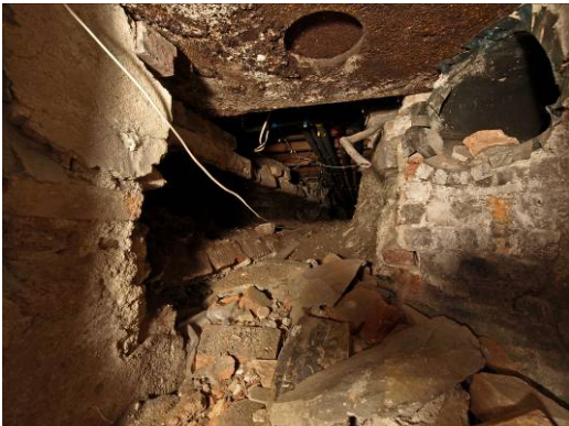
Plate 54 East Range rear basement (Room 30), inserted brick and copper flues looking south.
