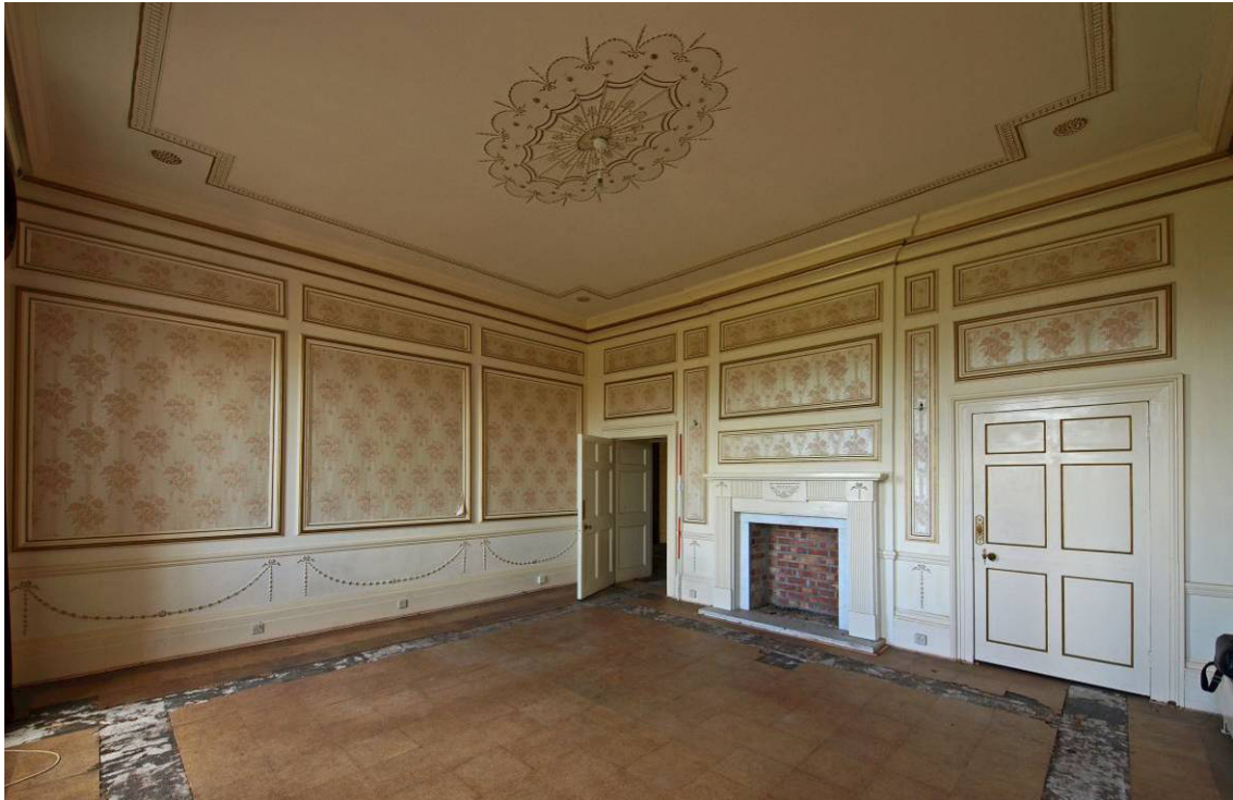
Plate 27 East Range, North Reception Room 1 with early 18 th century panelled scheme
