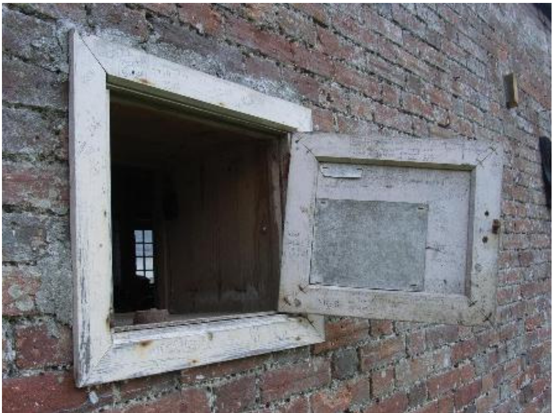
Plate 140 The telephone hatch in the Motor House, looking northeast.
