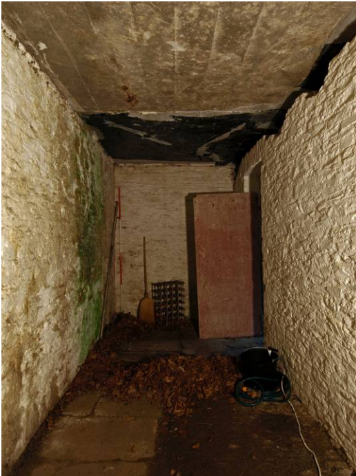
Plate 3 Northwest Wing: Cellar (Room 34) looking east
