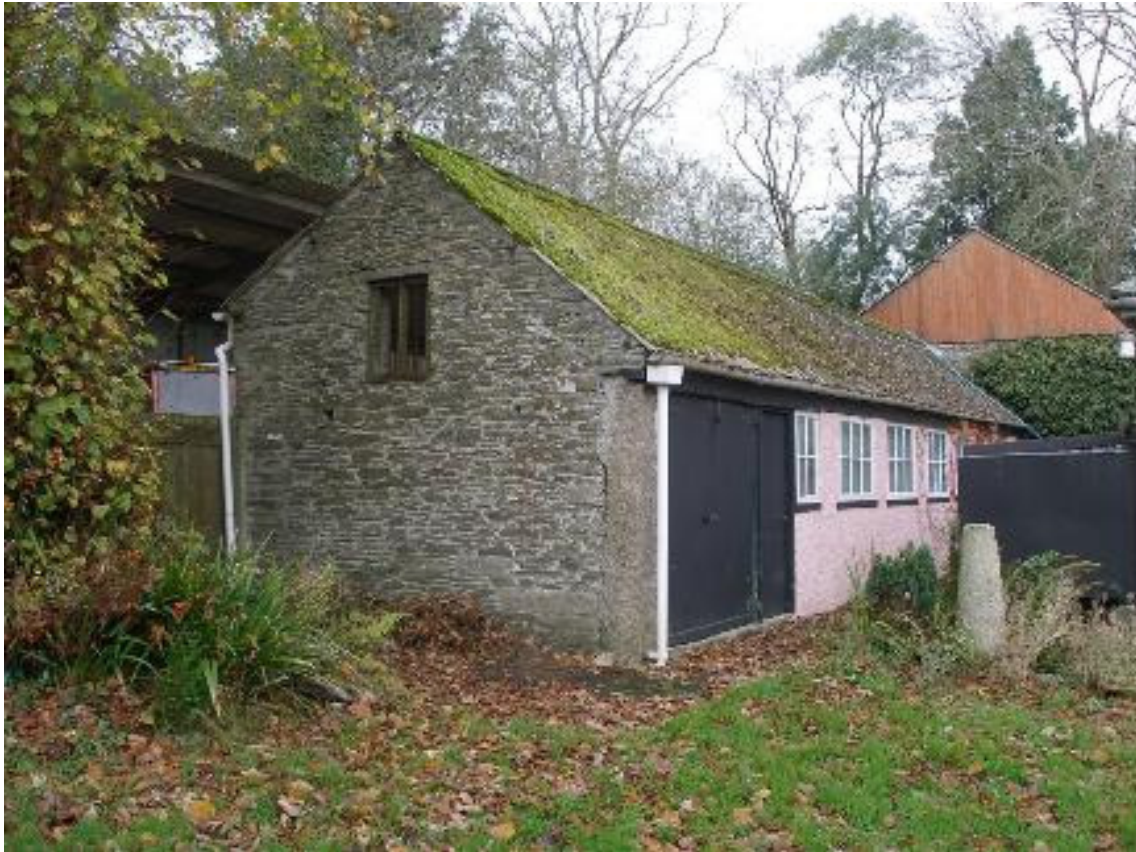
Plate 102 The workshop looking northwest.
