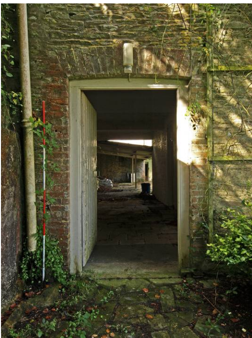
Plate 20 Rear Wing, south wall: doorway re-modelled from former window.
