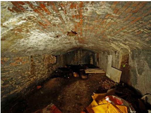
Plate 78 Coal Cellar (Room 36) looking south
