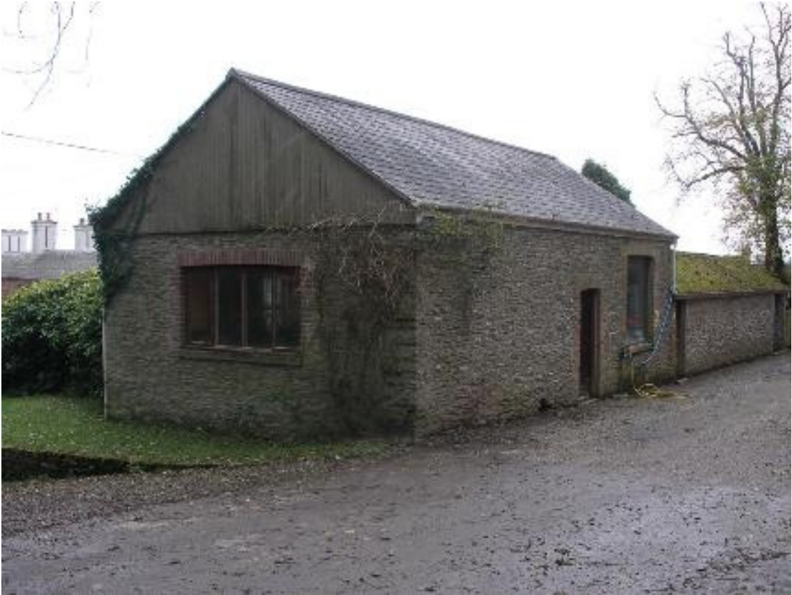
Plate 103 The office looking southeast
