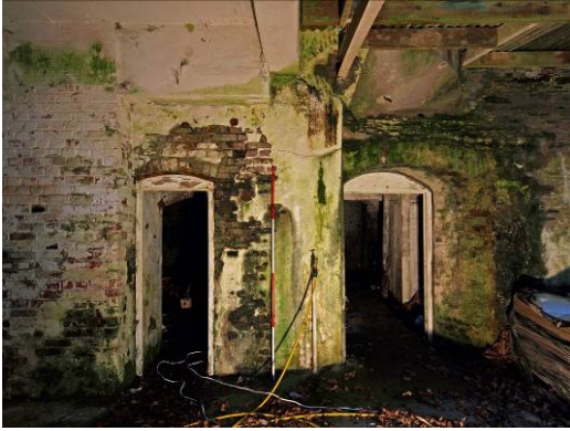
Plate 77 Coal Cellar doorways looking west
