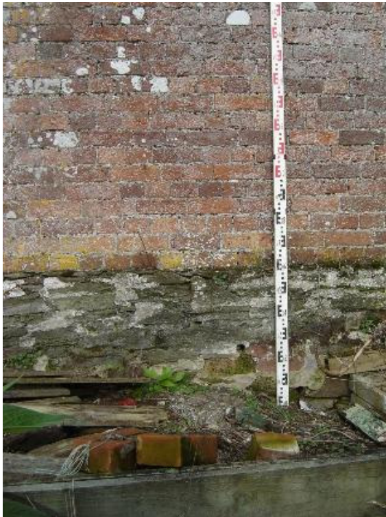
Plate 128 Foundation of the Workshop and Stores, south elevation
