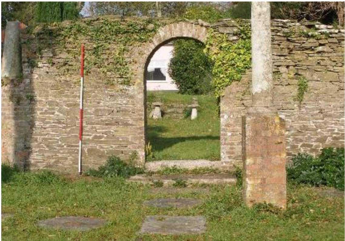
Plate 118 Brick relieving arch, part of a building shown on the Tithe Map of 1843, in the Walled Garden with granite pillar reused from the pond area.
