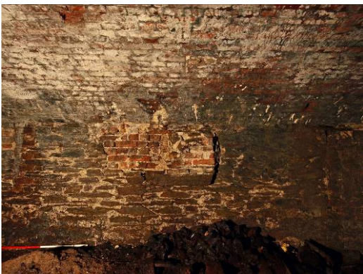
Plate 79 Coal Cellar (Room 36) looking east, showing blocked remains of probable oven.
