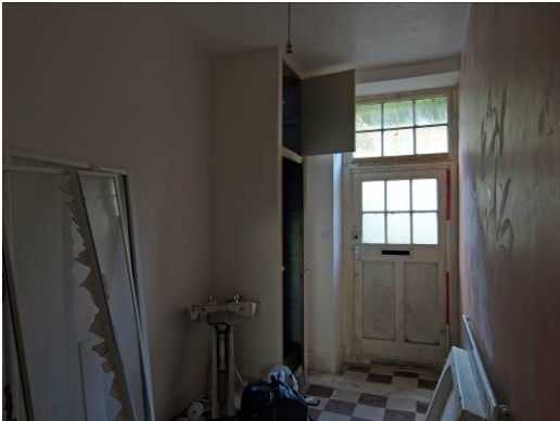
Plate 60 Rear Wing lobby (Room 17), looking north.
