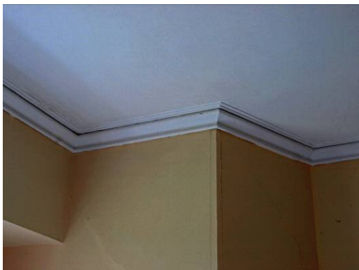
Plate 97 Room 46, this room created c.1831 within former probable stair wing, the thicker wall in the corner is part of the pre-1831 Rear Wing.
