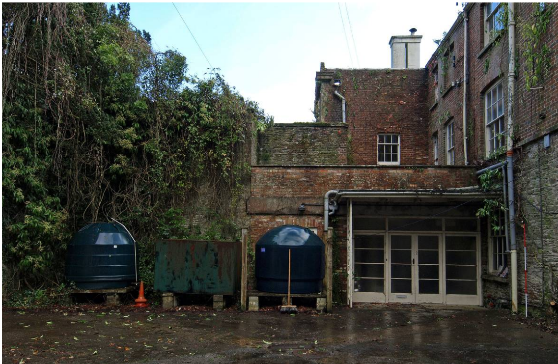
Plate 14 East Range, rear (west) elevation, north end
