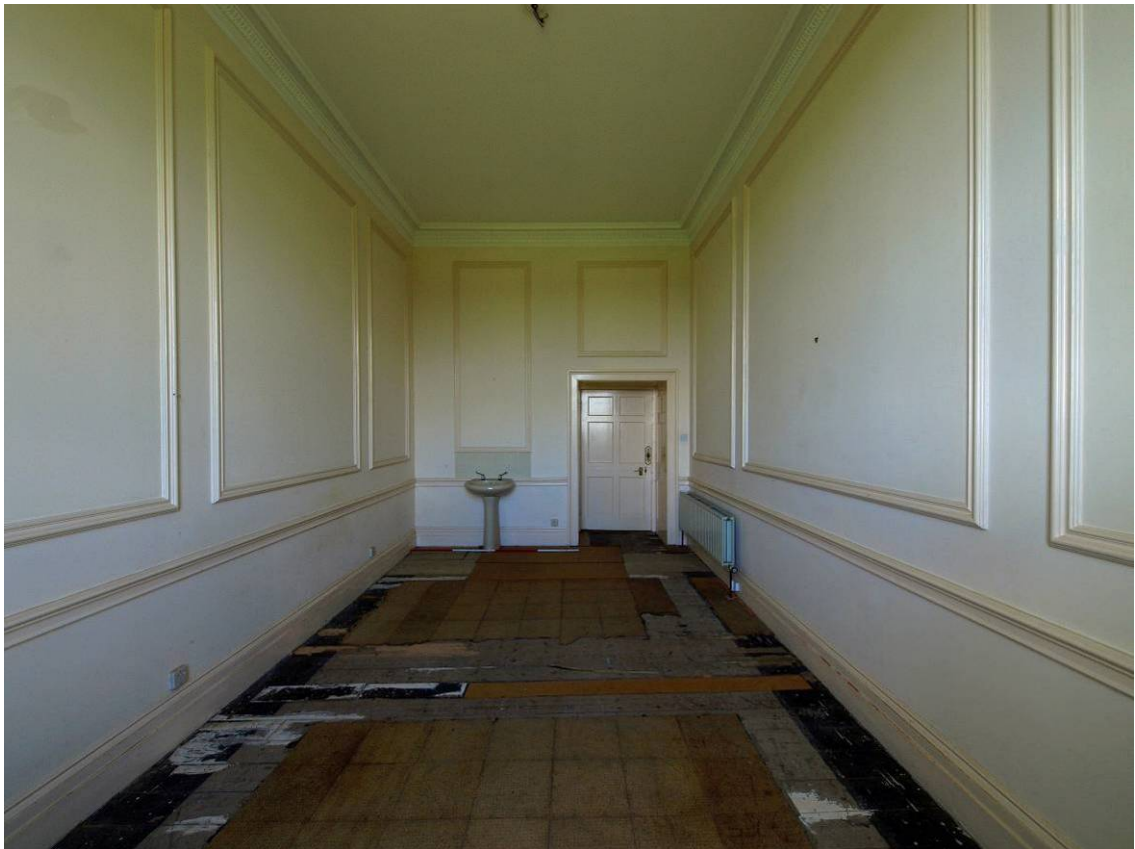
Plate 43 East Range, dressing room (Room 41) early 18 th century scheme
