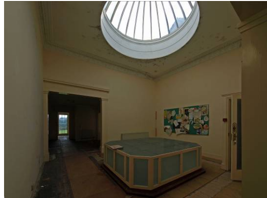
Plate 50 Former principal stair hall (Room 50), probably part of the 1831 scheme by Henry Harrison.
