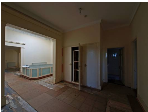
Plate 48 North landing vestibule (Room 49), to southwest and former principal stair hall.
