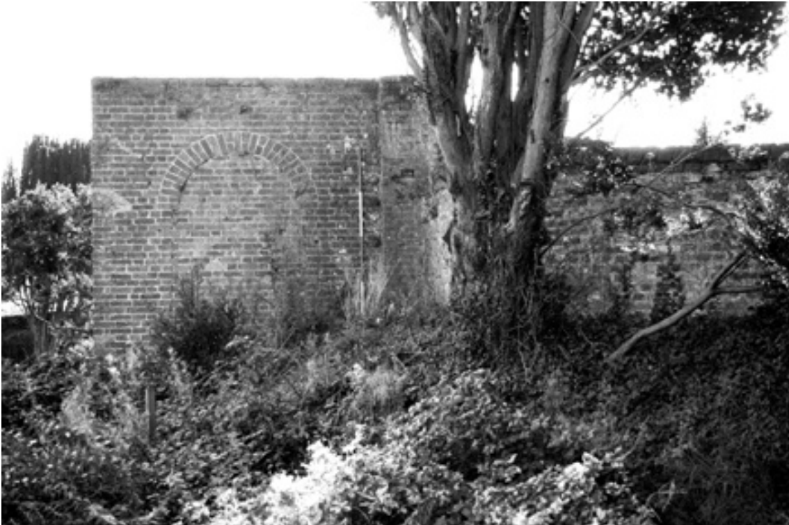
Plate 129 Blocked arched opening in the Flemish bond rebuilt walling of the north elevation of the Workshop and Stores building.
