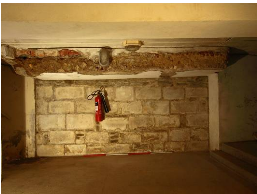
Plate 55 East Range basement (Room 30), stone ashlar walling under probable remains of original floor level.
