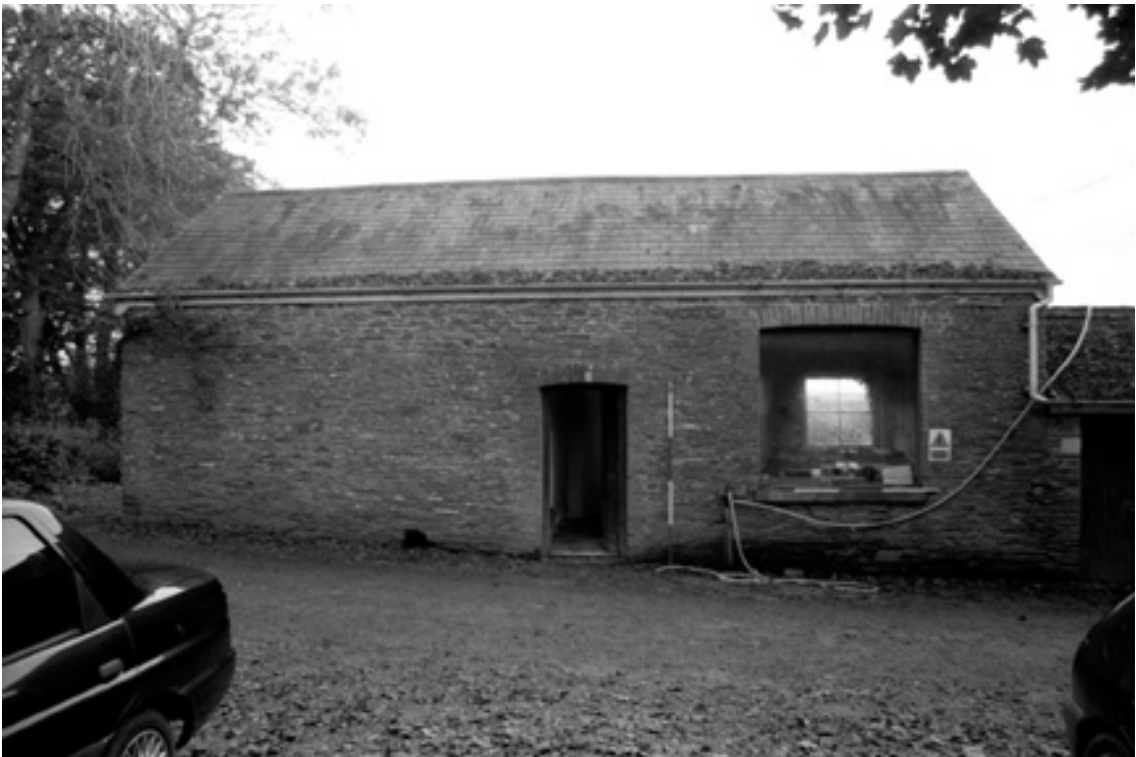
Plate 104 The office west elevation
