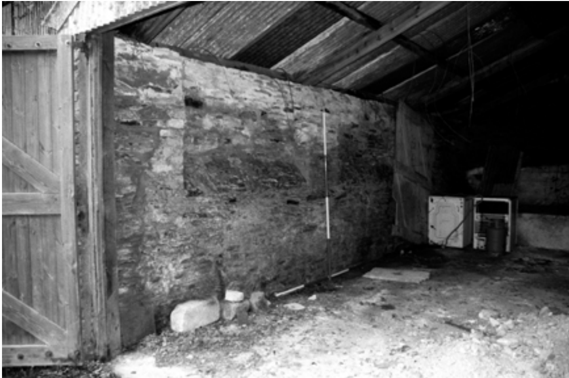
Plate 107 The interior of the southern part of the garage, looking southwest
