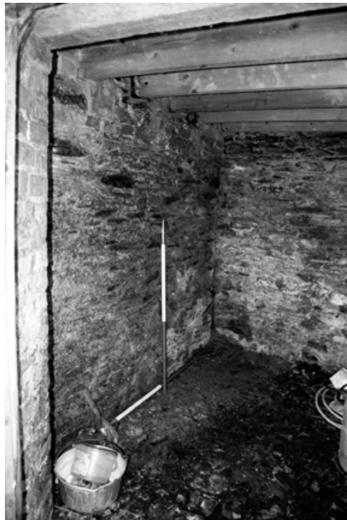
Plate 109 The ground floor interior of Woodside outhouse looking southwest
