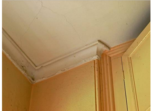
Plate 86 Room 5, probably created c.1831 when converted from a stair hall.
