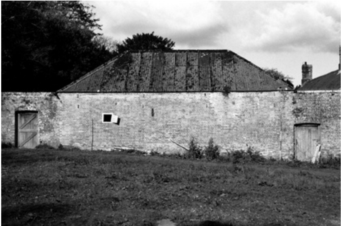
Plate 137 South elevation of the Motor House, showing communicating telephone hatch.
