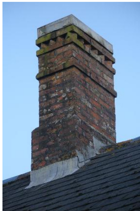
Plate 125 Detail of chimneystack with dog-toothed brickwork.
