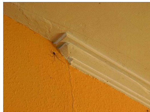
Plate 70 Rear Wing, first-floor service passage (Room 59), c.1831 ceiling cornice detail
