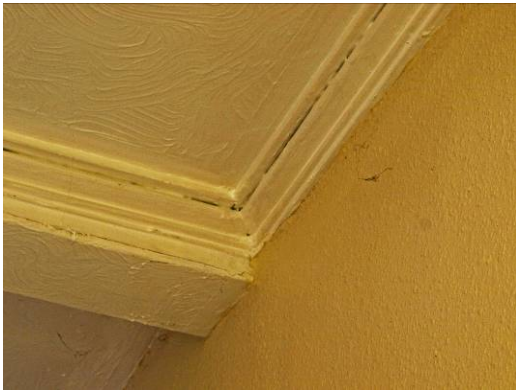
Plate 90 Rear Wing, ground-floor service Passage (Room 24)
