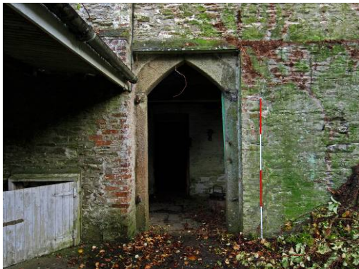
Plate 1 Northwest Wing: doorway to Room 33, the doorway constructed from probable 16 th or 17 th century granite fragments
