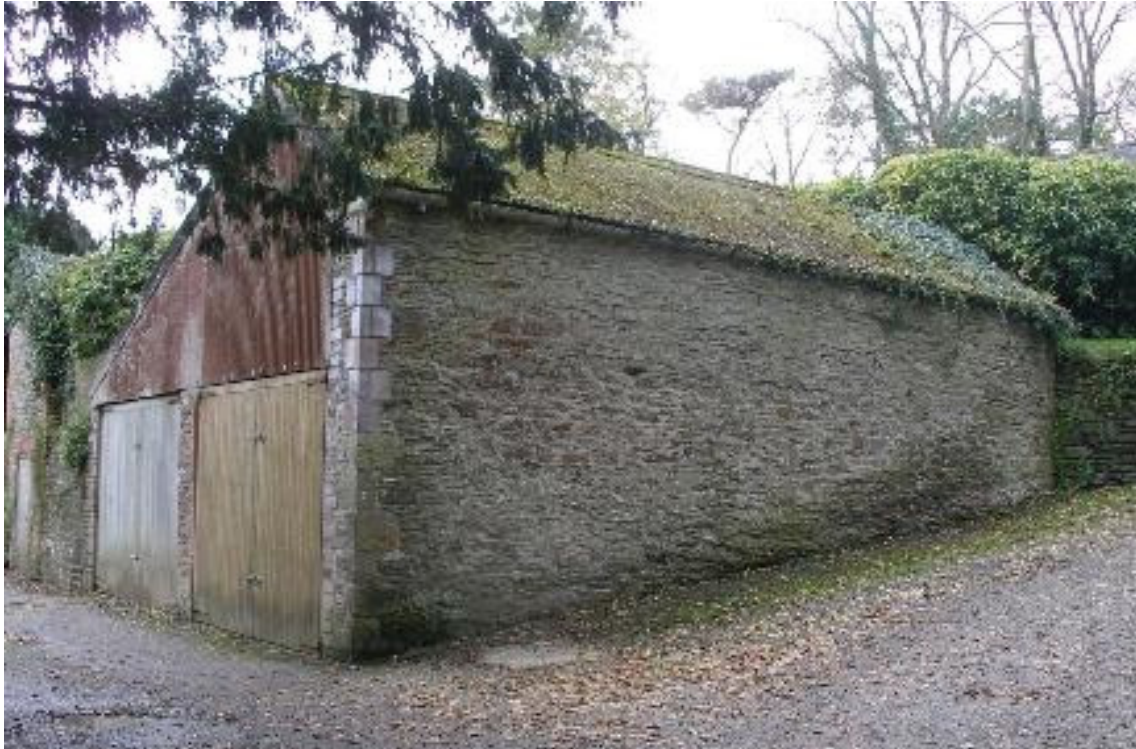
Plate 105 The garage looking southwest
