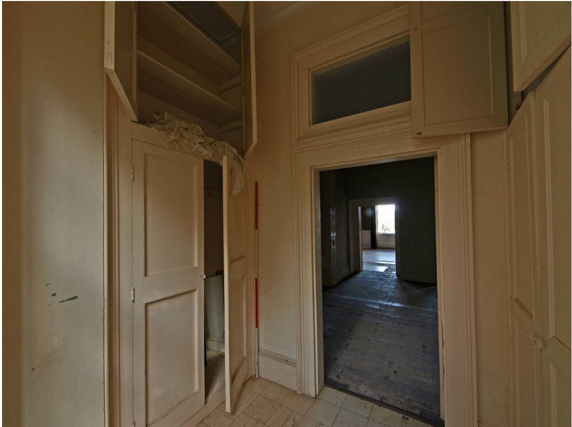
Plate 33 East Range, rear lobby (Room 5) in probable former stair wing, converted to room c1831
