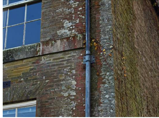
Plate 9 Platband inserted probably in 1831
