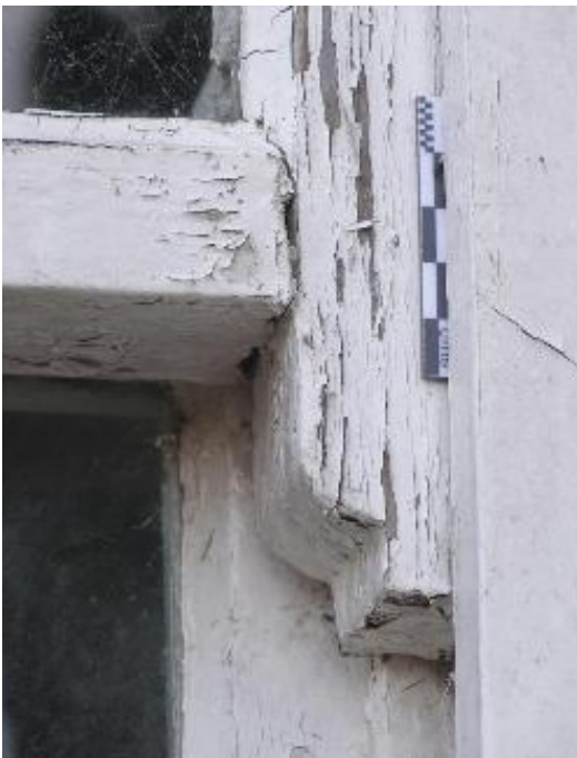
Plate 123 Detail of a horned sash window type 2
