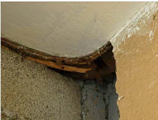
Plate 66 Rear Wing, first floor, Room 55 looking southeast showing curved ceiling detail from former c.1831 stair hall to east.
