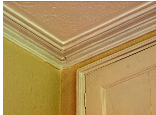
Plate 93 Rear Wing, Room 21, probable servants' parlour
