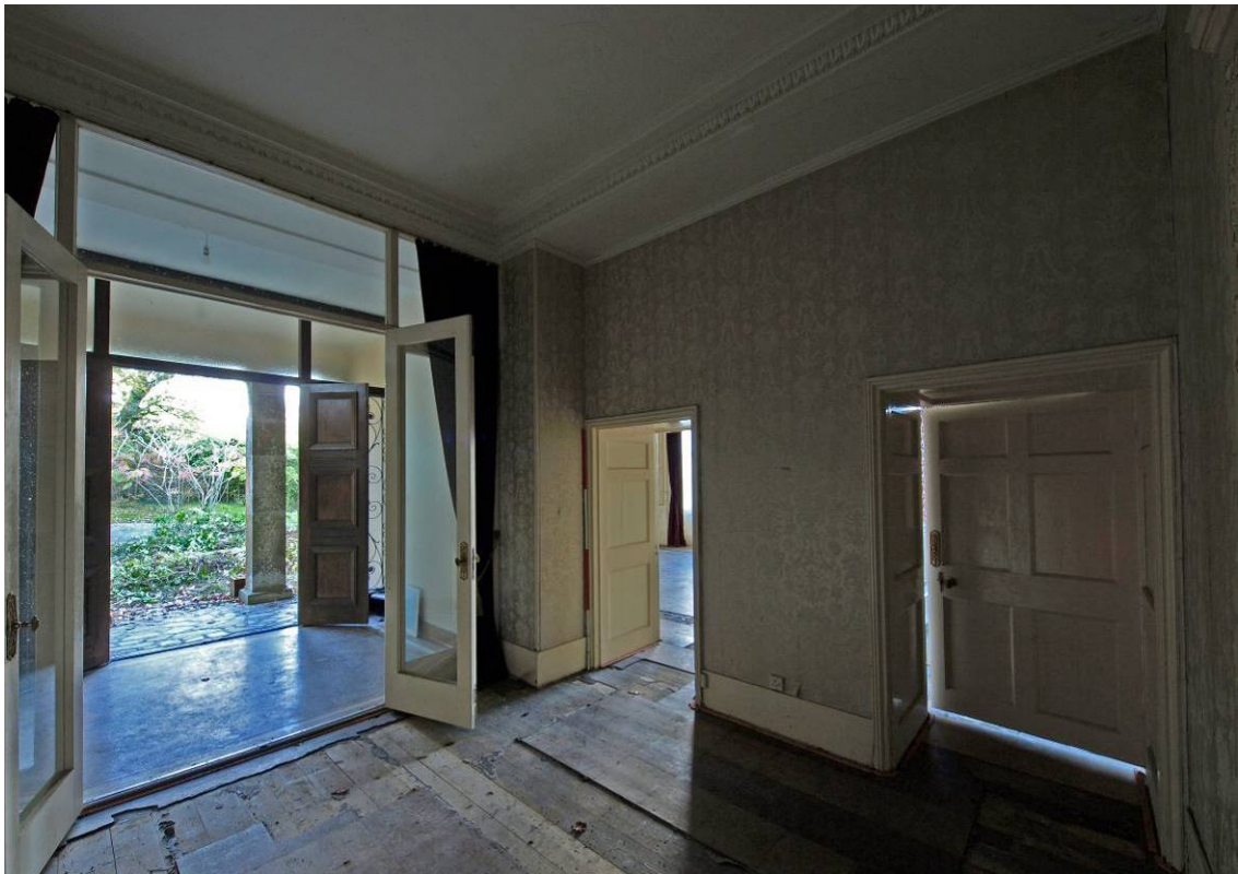
Plate 39 East Range, north vestibule (Room 12), looking northeast.
