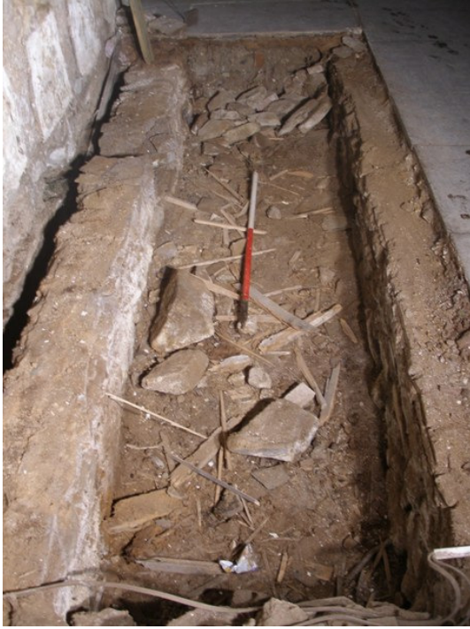
Plate 13 Sleeper walls below nave pew base, south side. Looking west
