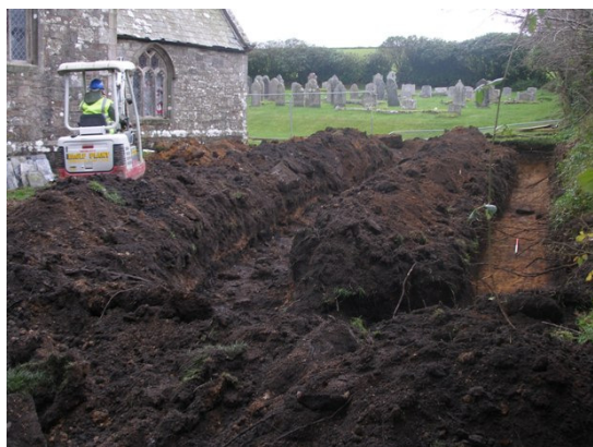
Plate 6 Service excavations to north of Church. Looking southwest.
