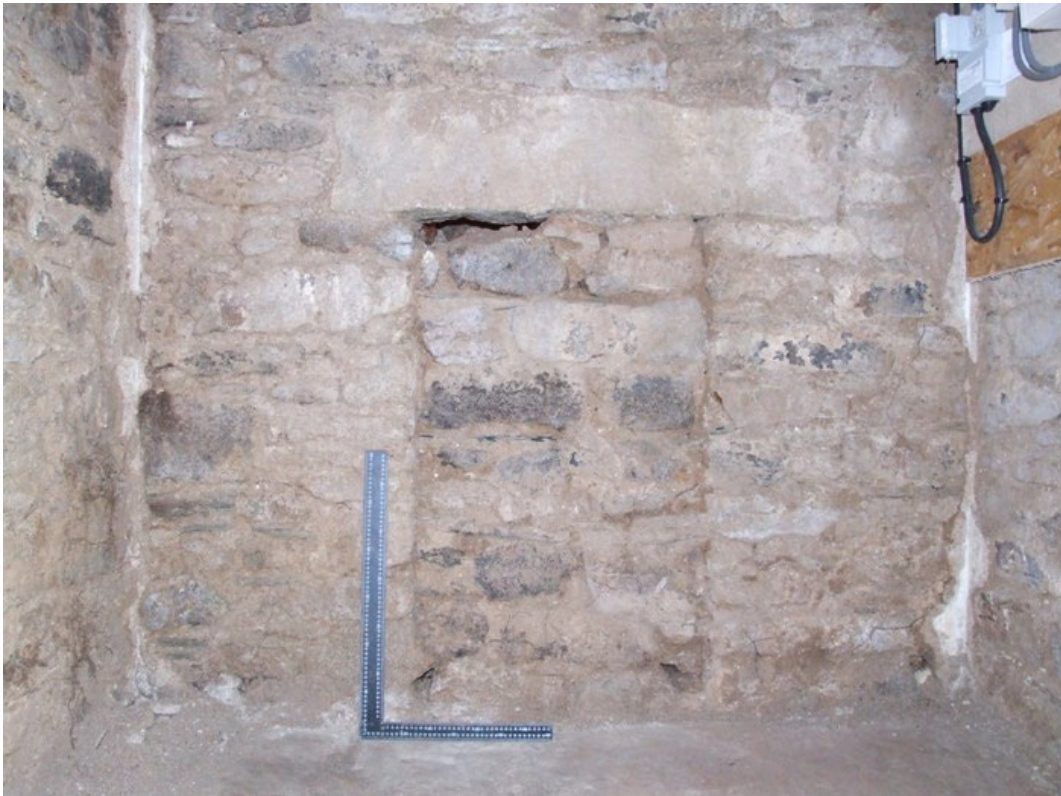
Plate 18 Blocked opening in west wall of vestry.
