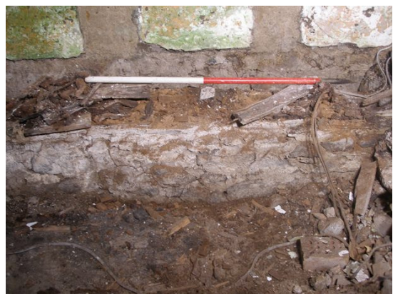
Plate 12 Sleeper wall below nave pew base. Looking north.
