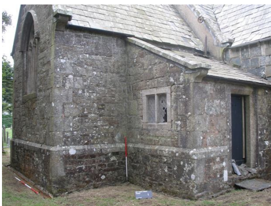
Plate 3 Chancel and lean-to vestry. Looking southwest.
