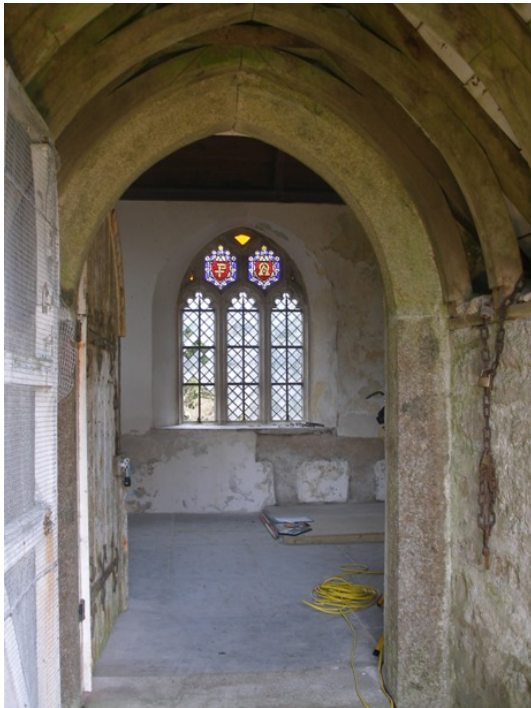
Plate 14 Porch with north window of nave in the background. Iron stanchions in front of the replaced principal lights with original tracery-lights with chi-rho and alpha and omega monograms.
