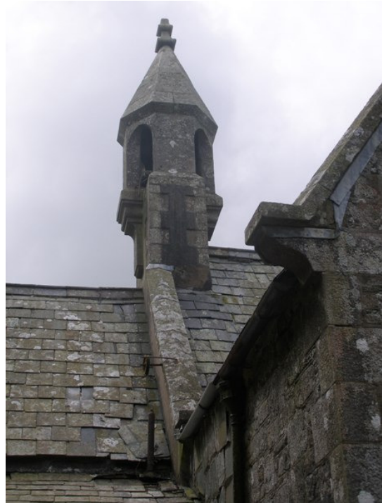
Plate 4 Bellcote and bell pull system. Looking south.
