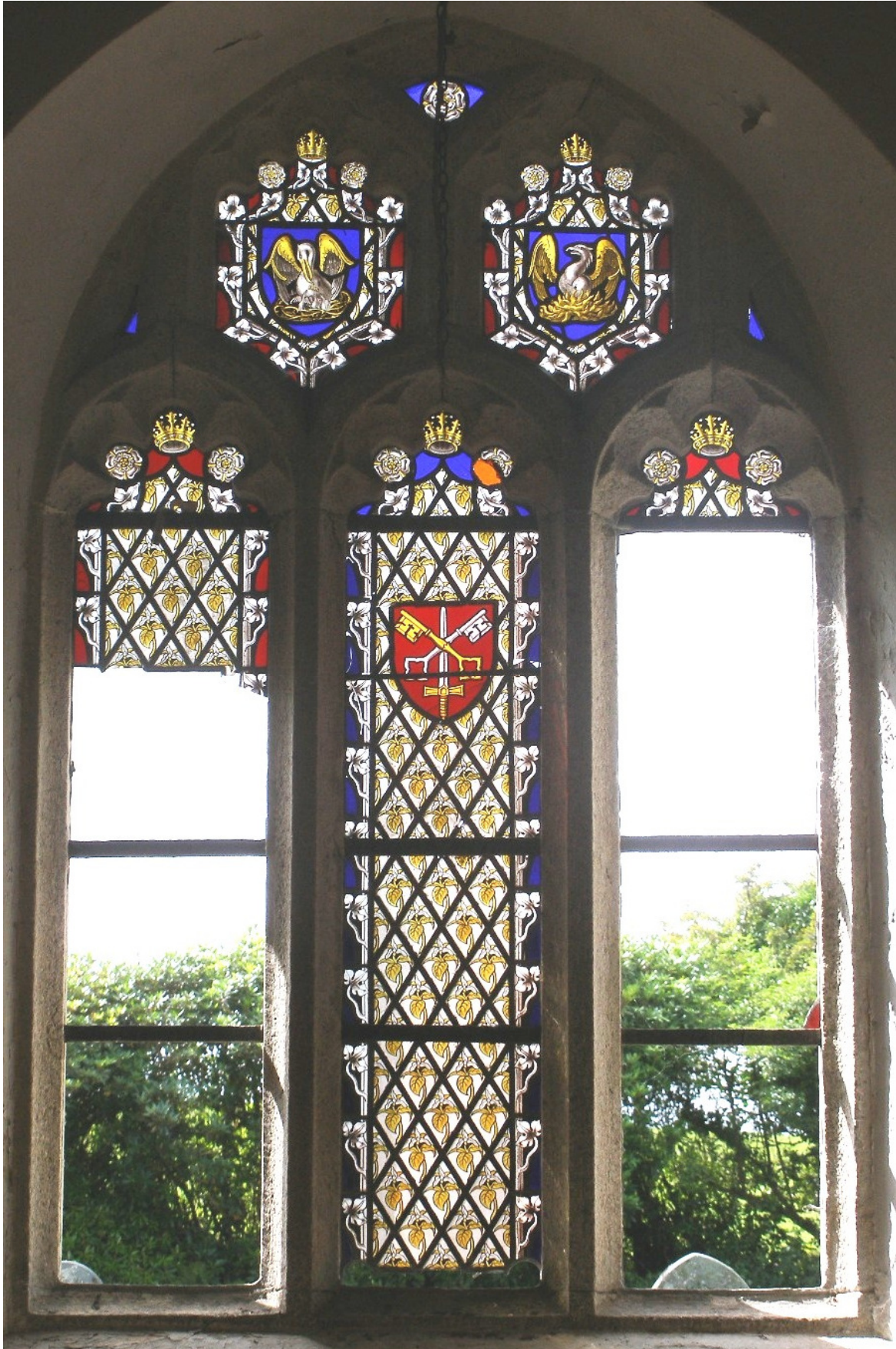
Plate 17 Vandalised west window showing the decorative quarry glass.
