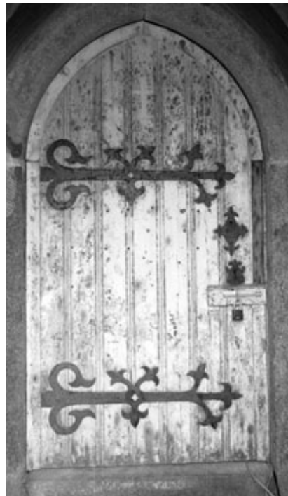
Plate 16 Intricate iron strap hinges on the church door, looking north.
