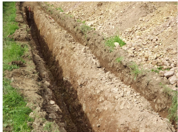
Plate 5 Trench 2 with the geotechnical test trench within. Looking north.
