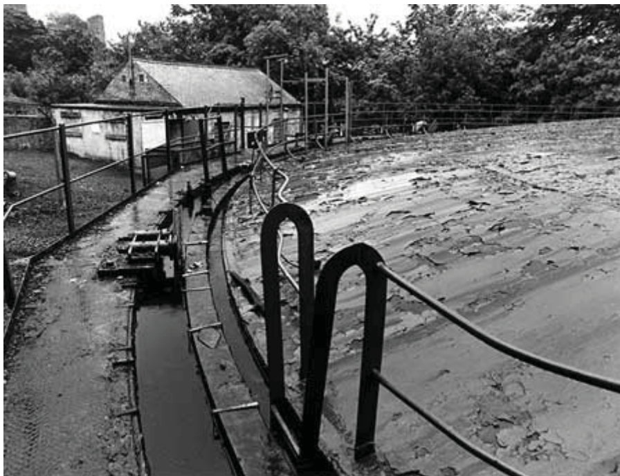
Figure 4: This gasometer in Durham is fully retracted, allowing a close-up view of its domed top. It would rise in telescopic sections, the water helping to create a seal (© English Heritage, NMR)
