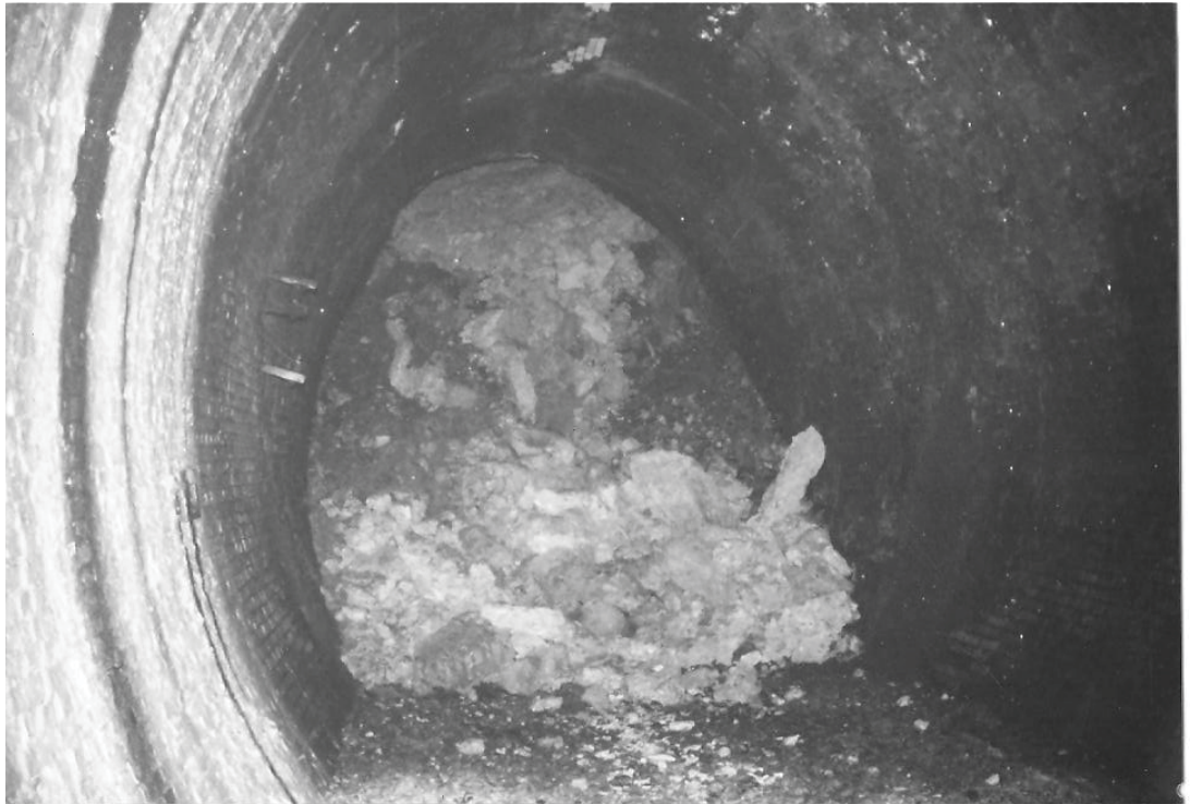
Figure 37 Tunnel collapse at Burdale photographed in the 1970s (photo courtesy of Mike Elliott)
